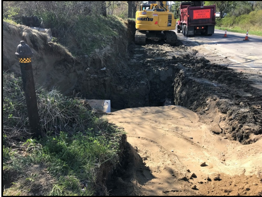
Photograph 1 – Wednesday, May 09 th – Field inlet installation along with 15" hdpe drainage pipe.
