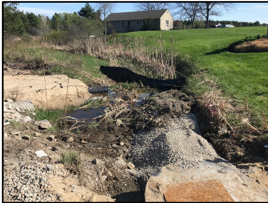
Photograph 3 - Wednesday, May 09 th – Drain manhole and catch basin installation along with outlet pipes
