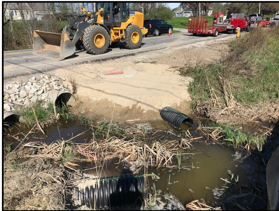
Photograph 2: Wednesday, May 09 th – Catch Basin and outlet pipe installation.
