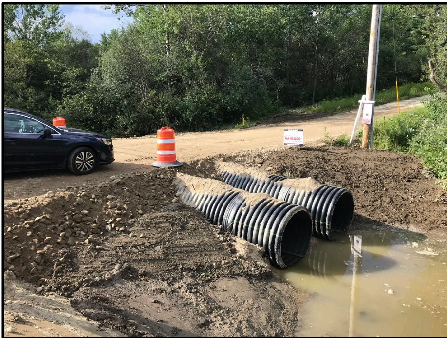
Photograph 4 - Friday, August 3 rd – New Culverts at Bunkers Way
