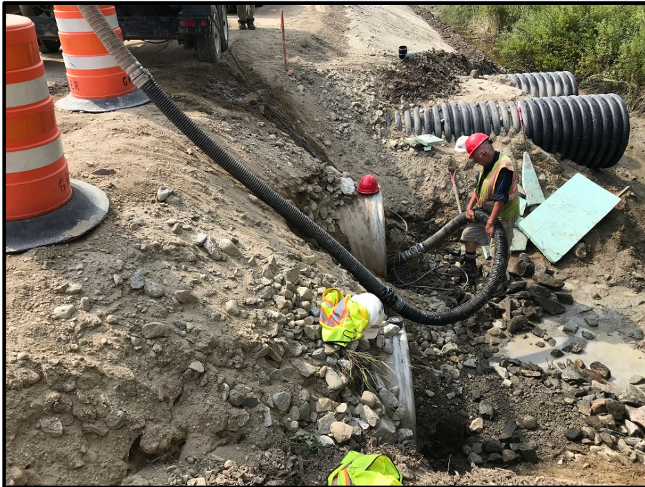
Photograph 7 - Tuesday, August 7 th – Cleaning culverts for slip lining
