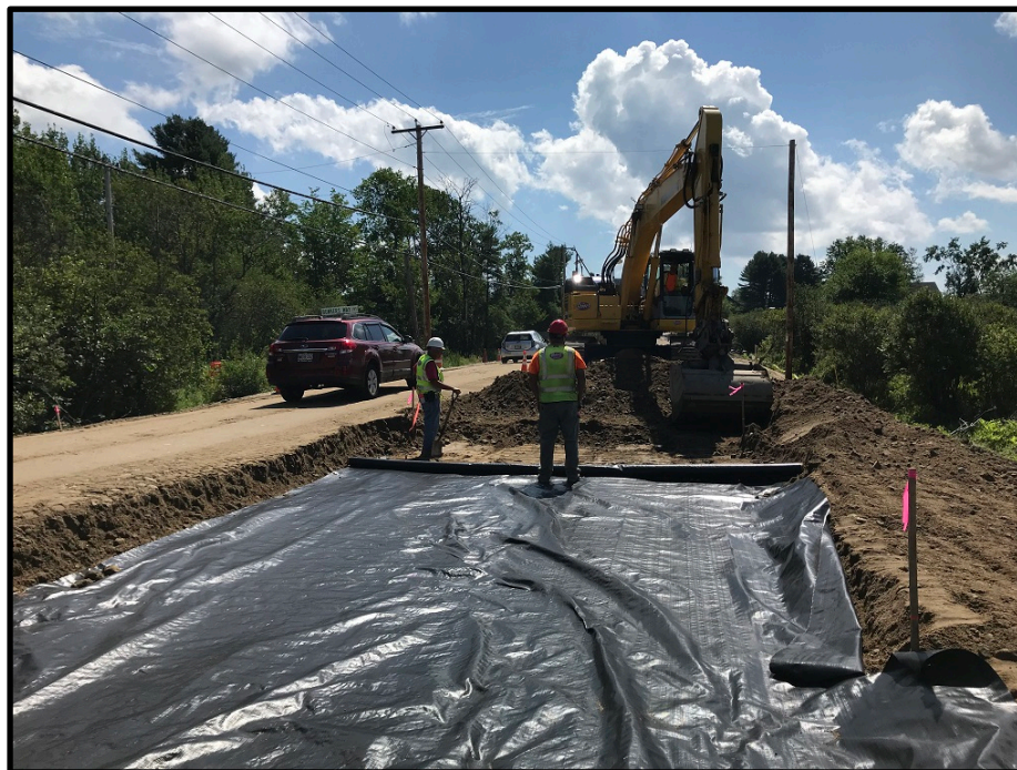
Photograph 2: Thursday, August 2 nd – Excavating to base great for full depth road reconstruction
