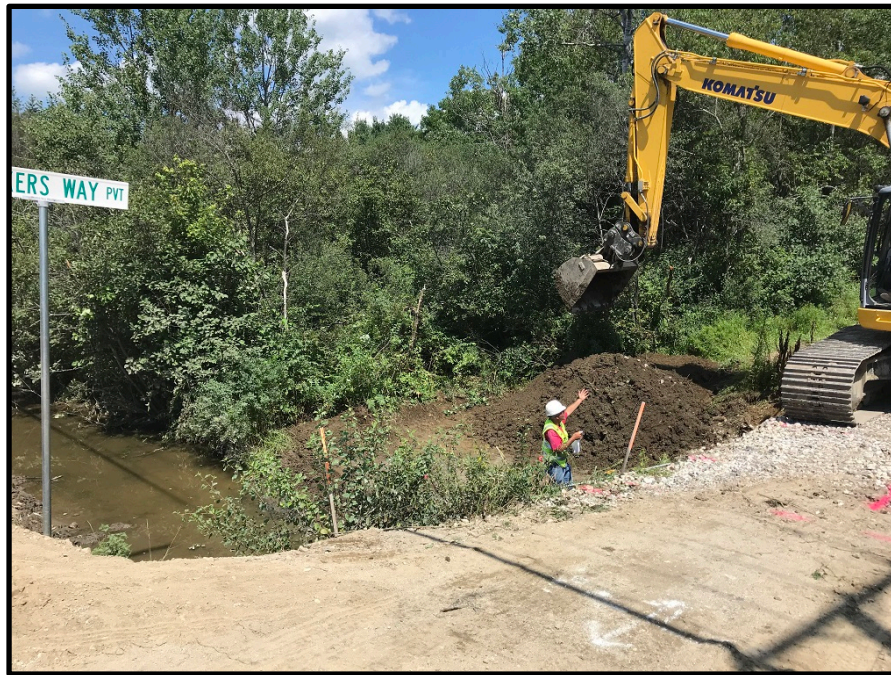
Photograph 3 - Friday, August 3 rd – Preparing for culvert installation at Bunkers Way
