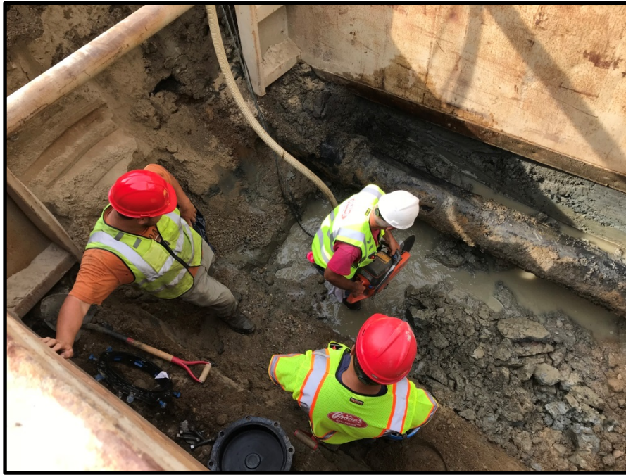
Photograph 5 - Monday, July 30 th – Preparing to make connection with existing water main
