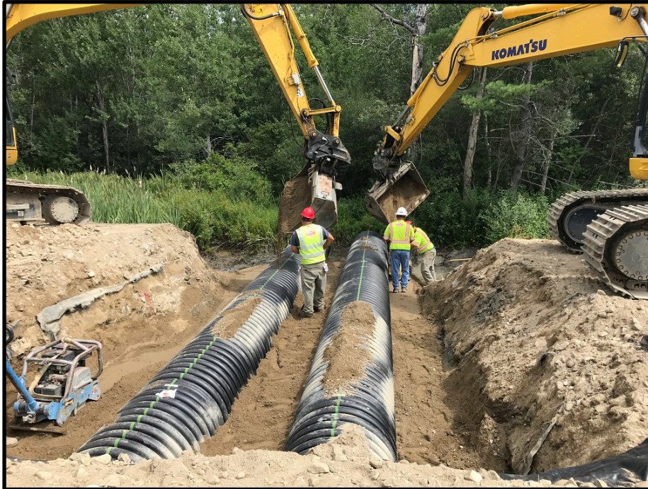
Photograph 9 - Wednesday, August 1 st – Compacting around culverts at approximate STA 7+00
