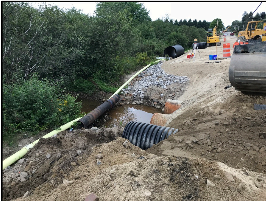
Photograph 10 - Wednesday, August 1 st – Outlet for 36 inch culvert at approximate STA 9+80
