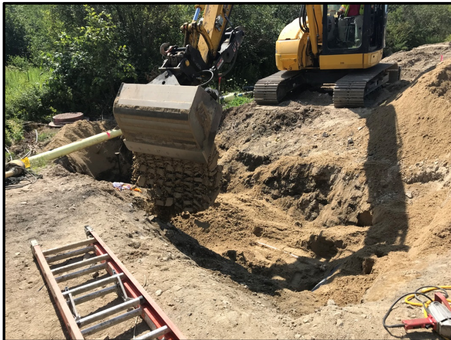
Photograph 8 - Tuesday, July 31 st – Backfilling around service for October Farms Way
