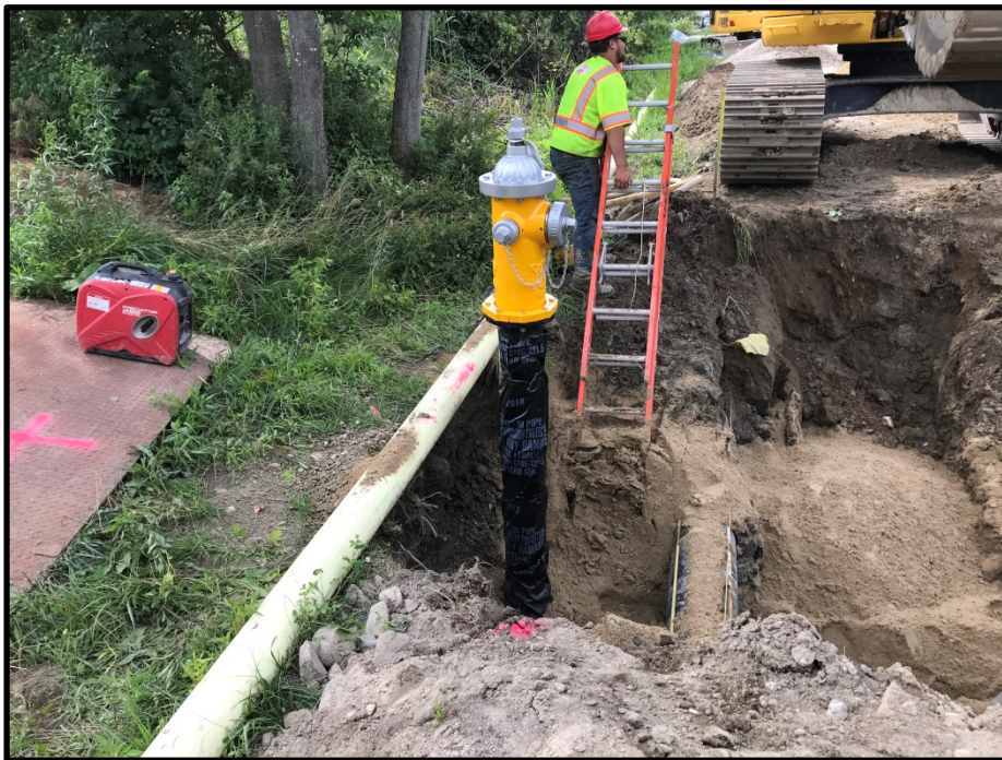
Photograph 6 - Monday, July 30 th – Installed hydrant at east end of the project
