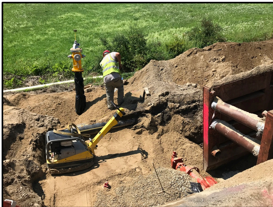
Photograph 4 - Friday, July 27 th – Compacting sand around hydrant assembly
