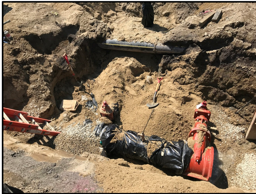
Photograph 3 - Friday, July 27 th – Installing hydrant assembly and air release valve
