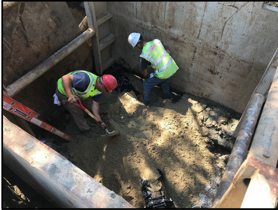
Photograph 3 - Friday, July 20 th – Placing sand over 45 degree bends near PWD pump house
