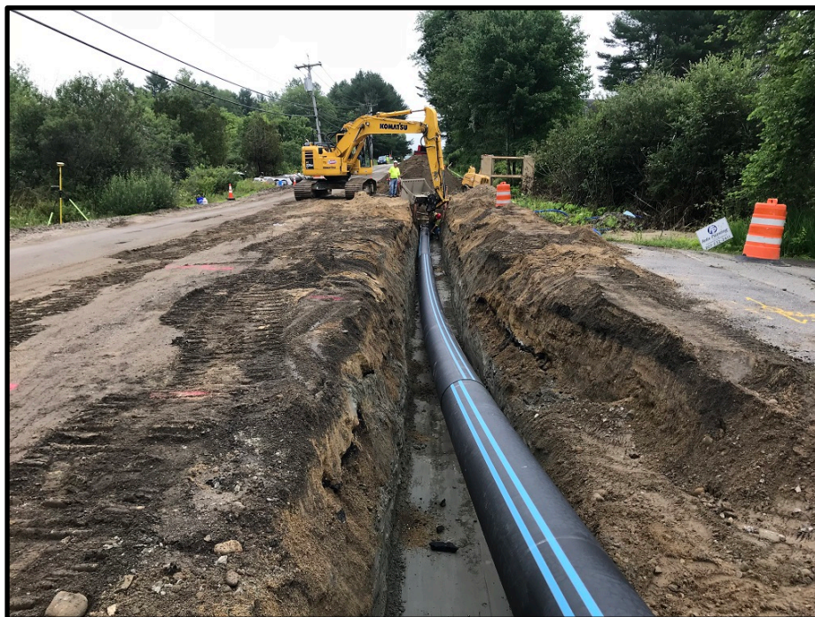
Photograph 6 - Monday, July 23 th – Installing 16 inch HDPE water main
