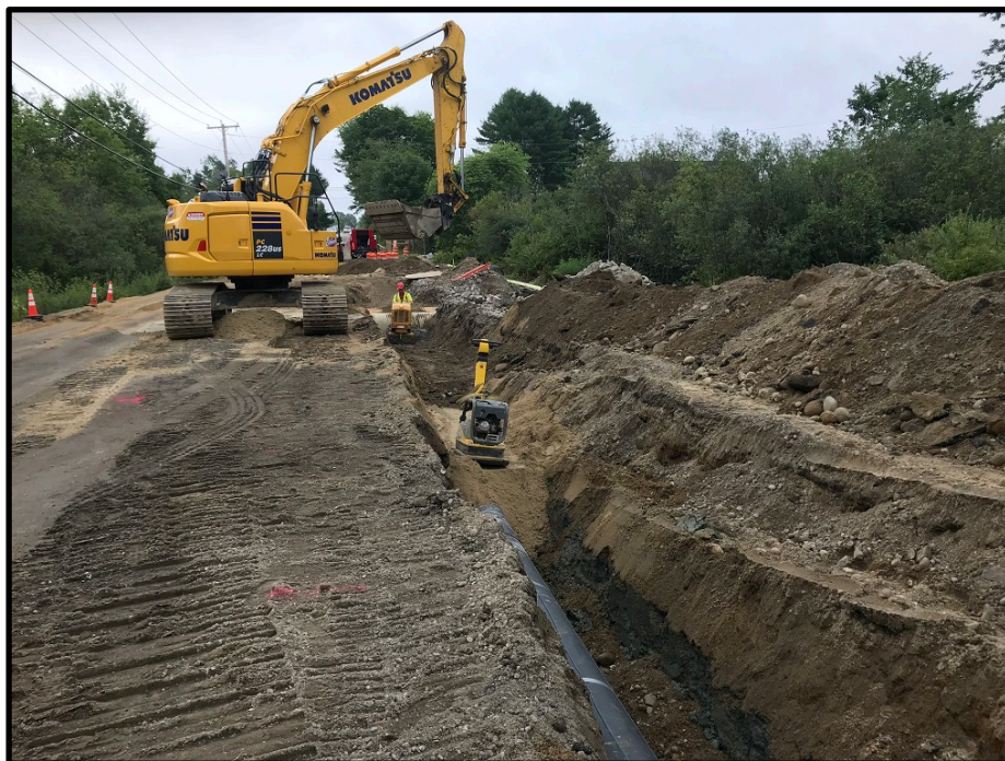
Photograph 8 - Tuesday, July 24 th – Backfilling 16 inch HDPE water main
