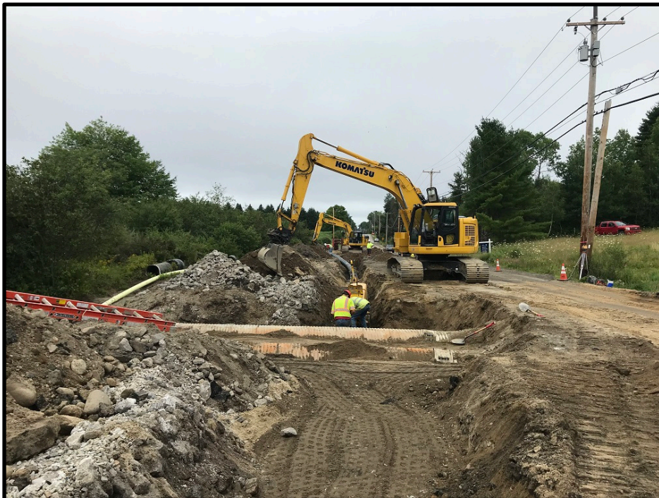
Photograph 7 - Tuesday, July 24 th – Installing 16 inch HDPE water main
