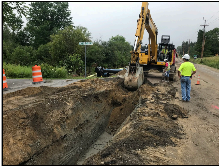
Photograph 5 - Monday, July 23 th – Excavating to install 16 inch HDPE water main
