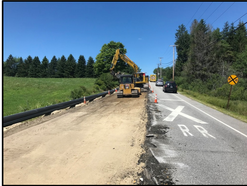
Photograph 1 – Thursday, July 19 th – Removing pavement near rail road tracks
