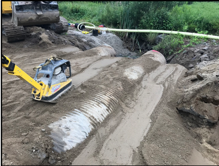
Photograph 9 - Wednesday, July 25 th – Compacting around culverts after going under them with the 16 inch HDPE water main
