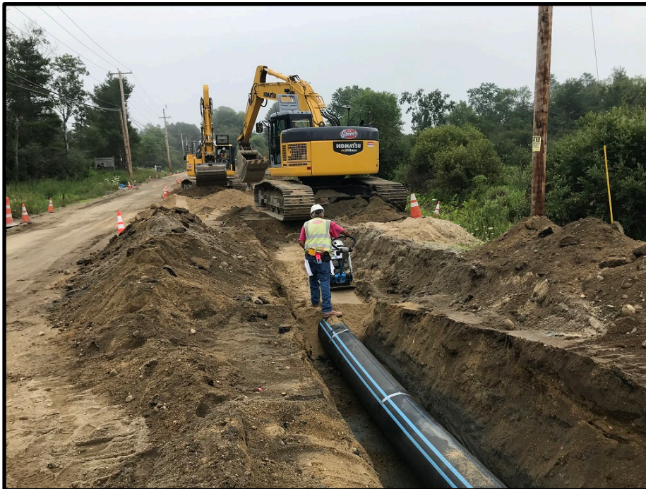
Photograph 10 - Wednesday, July 25 th – Compacting the sand over the 16 inch HDPE water main
