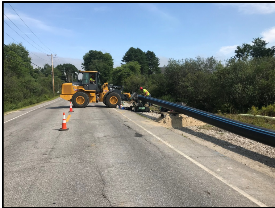
Photograph 5 - Monday, July 16 th – Fusing 16 inch HDPE water main
