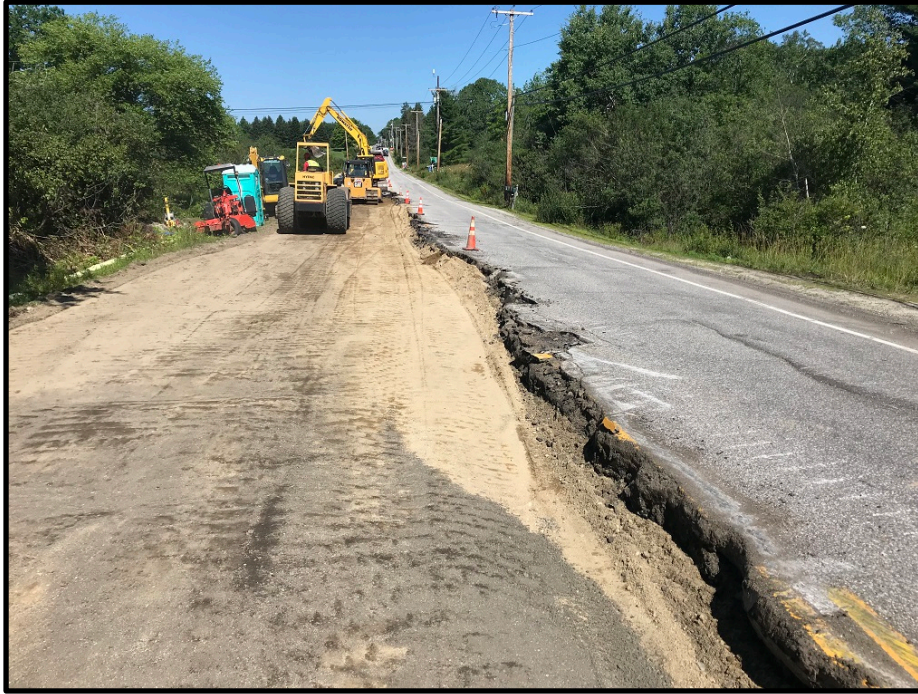
Photograph 9 - Wednesday, July 18 th – Removing pavement on south side of Tuttle Road
