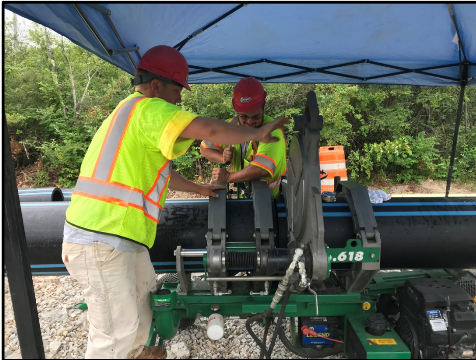
Photograph 7 - Tuesday, July 17 th – Fusing 16 inch HDPE water main
