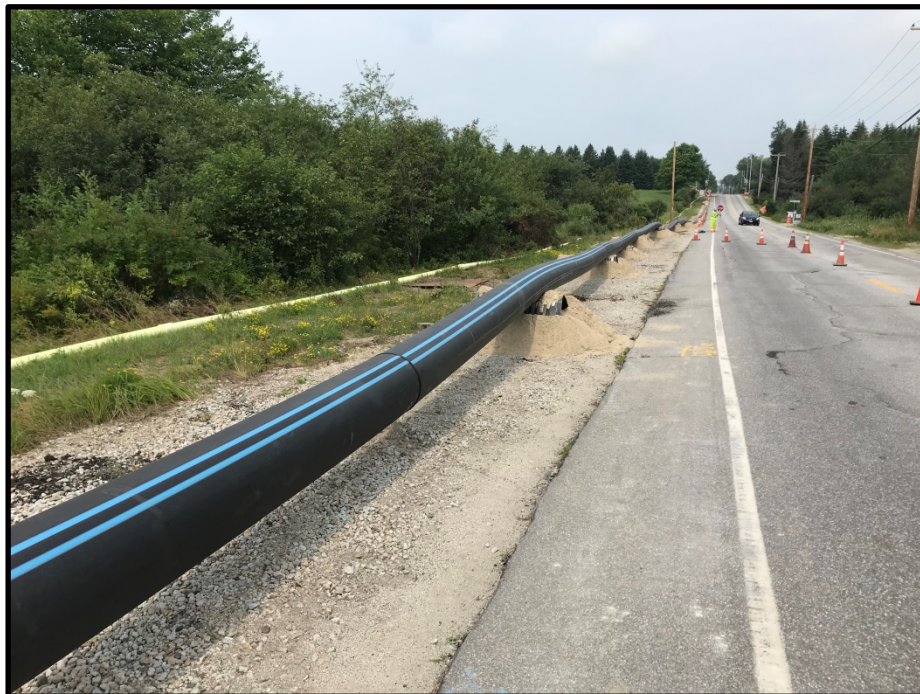
Photograph 8 - Tuesday, July 17 th – 16 inch HDPE water main fusing complete
