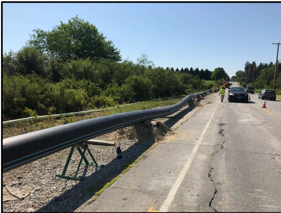
Photograph 4 - Friday, July 13 th – Fused 16 inch HDPE water main approx. half done
