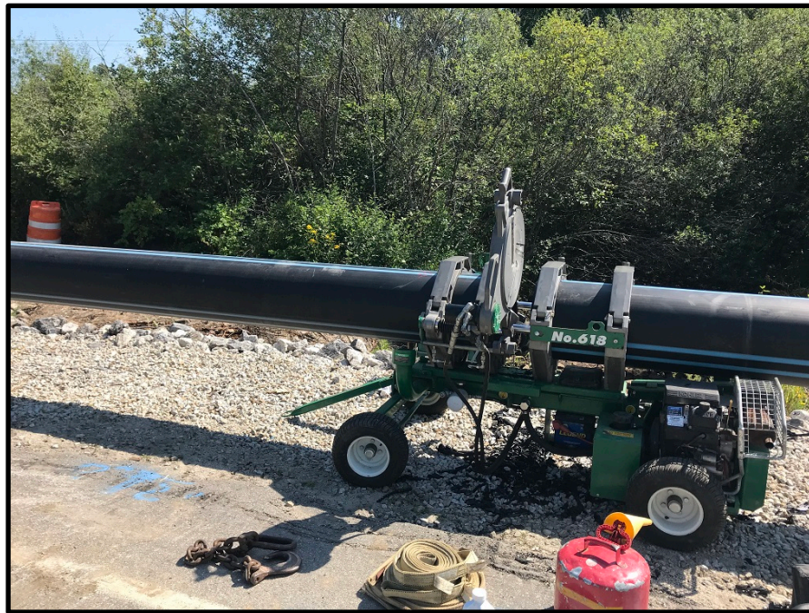
Photograph 3 - Friday, July 13 th – Fusing 16 inch HDPE water main
