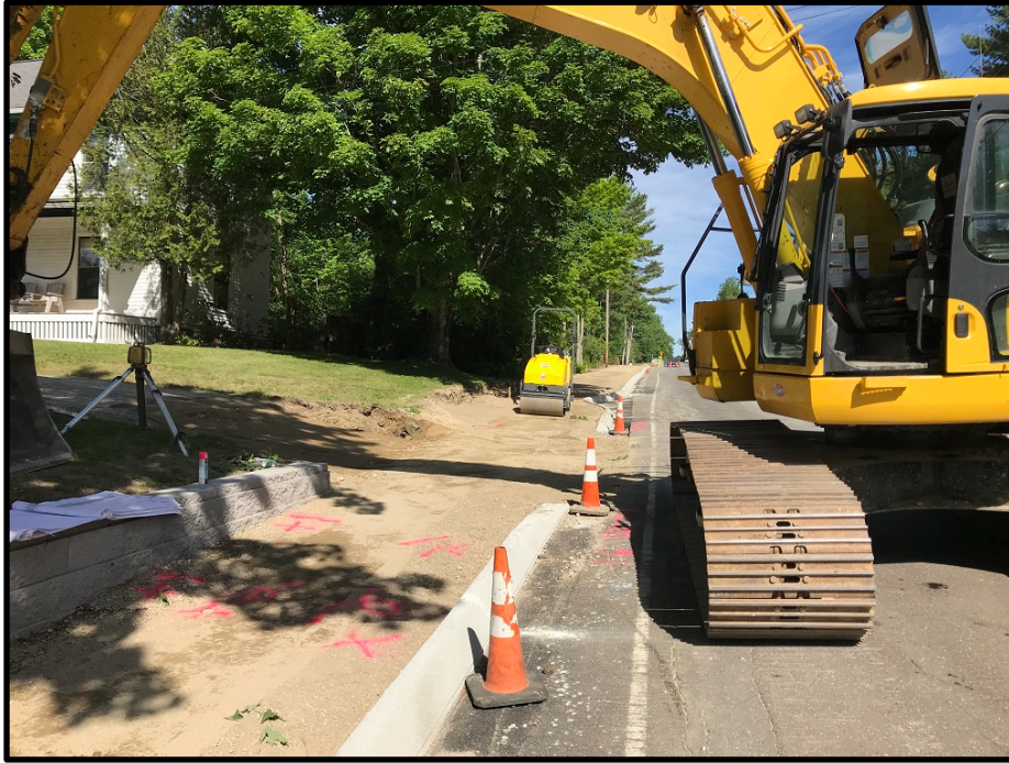
Photograph 9 - Wednesday, June 20 th – Placing gravel for sidewalk at 280 Tuttle Road
