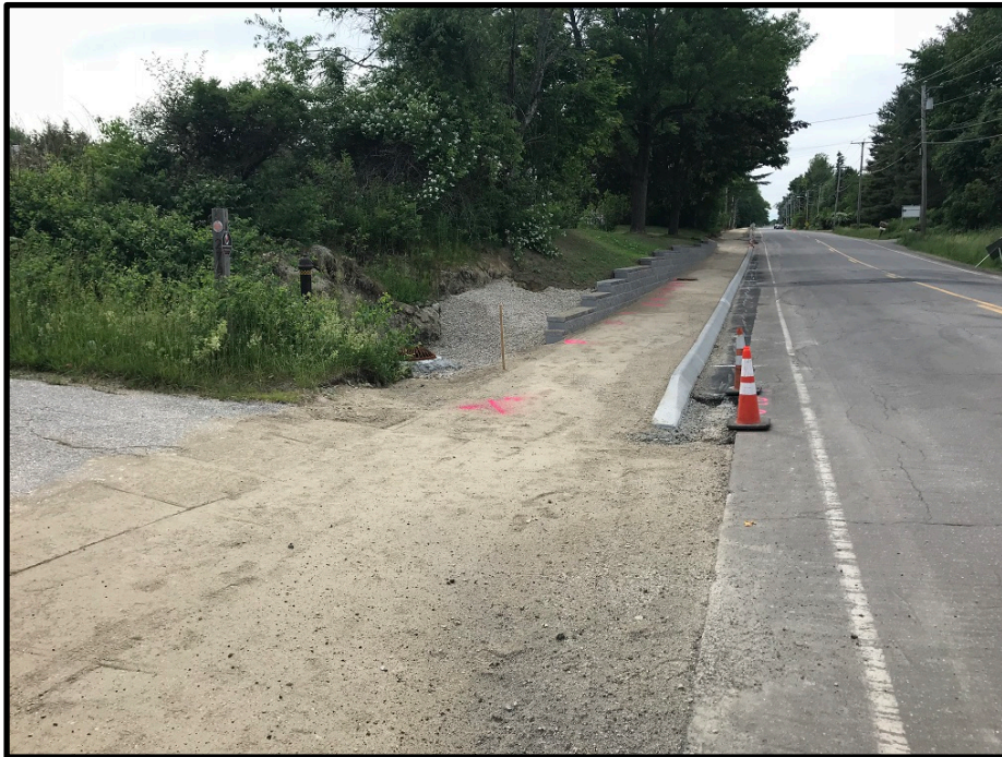
Photograph 10 - Wednesday, June 20 th – Placing and grading gravel for sidewalk near 272 Tuttle
