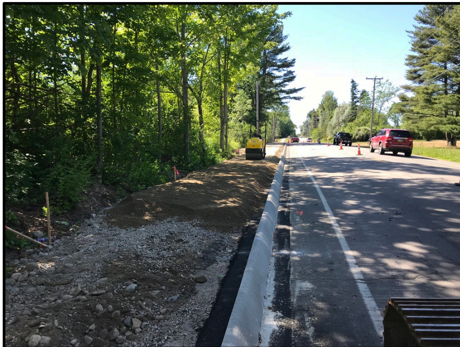
Photograph 8 - Tuesday, June 19 th – Compacting gravel for sidewalk extension
