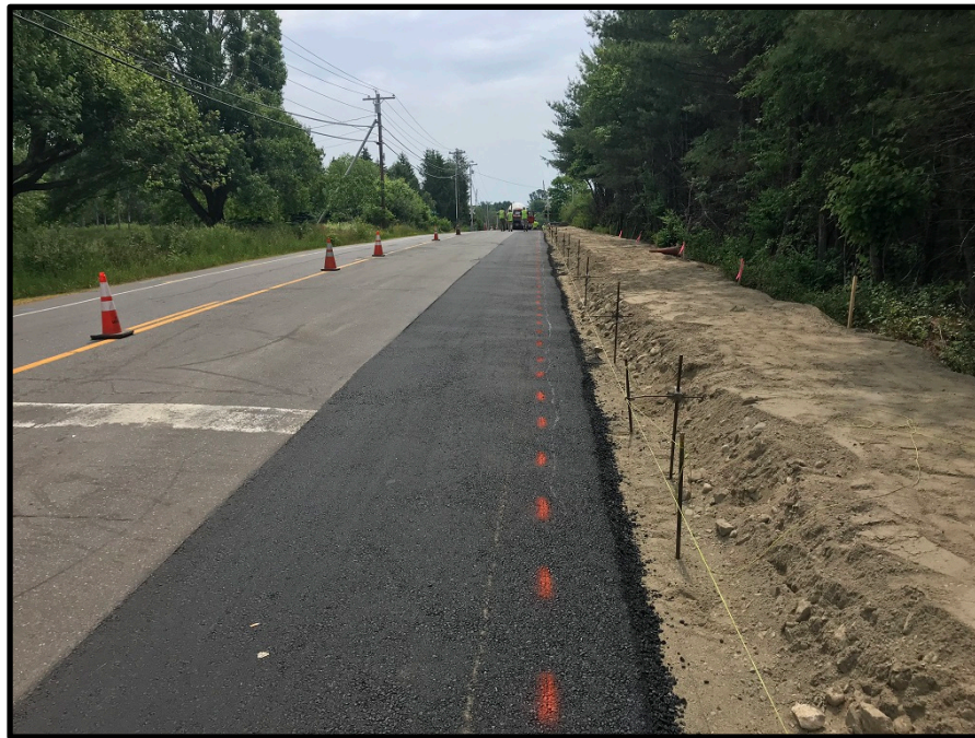
Photograph 5 - Monday, June 18 th – Laying out for curb near rail road tracks
