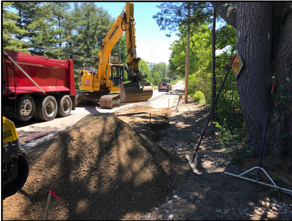
Photograph 7 - Tuesday, June 19 th – Placing and grading gravel for sidewalk at 290 Tuttle Road
