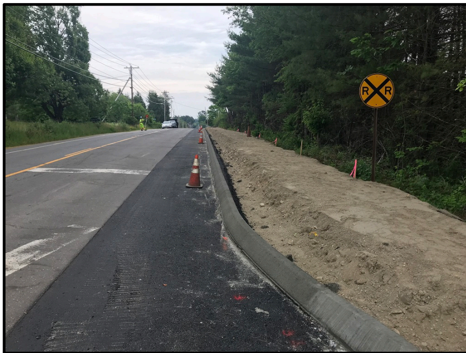
Photograph 6 - Monday, June 18 th – Concrete slipform curb near rail road tracks
