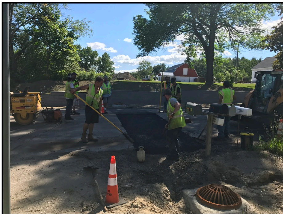
Photograph 4 - Friday, June 15 th – Paving cross trench in front of 280 Tuttle Road
