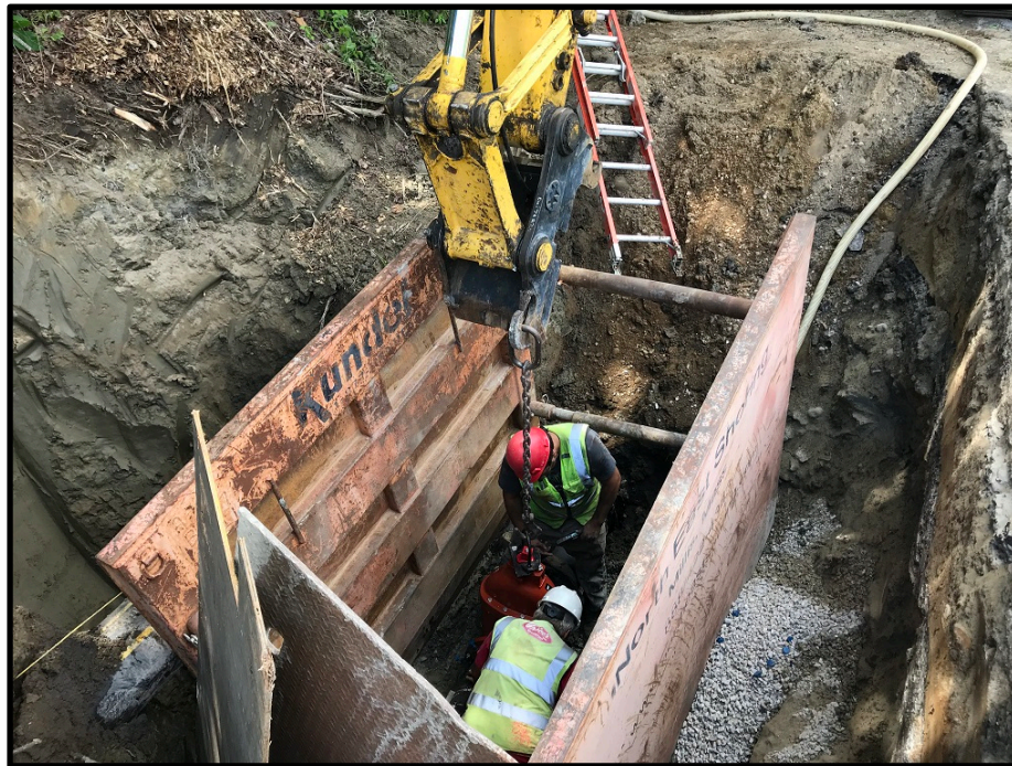
Photograph 2: Thursday, June 21 st – Installing 12 inch gate valve for eventual water main replacement on east side of limit of work.
