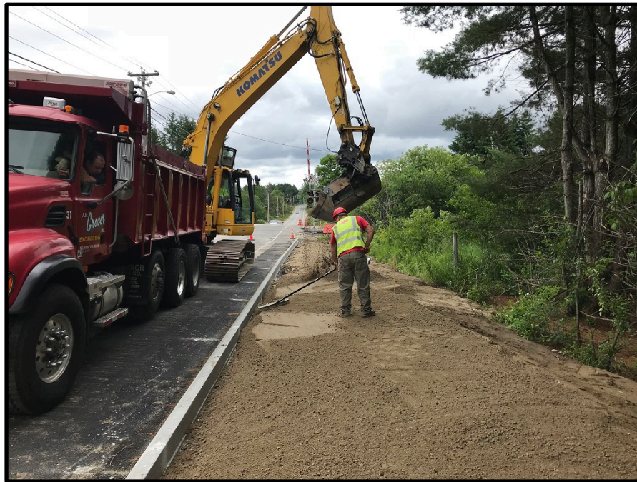
Photograph 5 - Monday, June 25 th – Placing and grading gravel for sidewalk near rail road tracks
