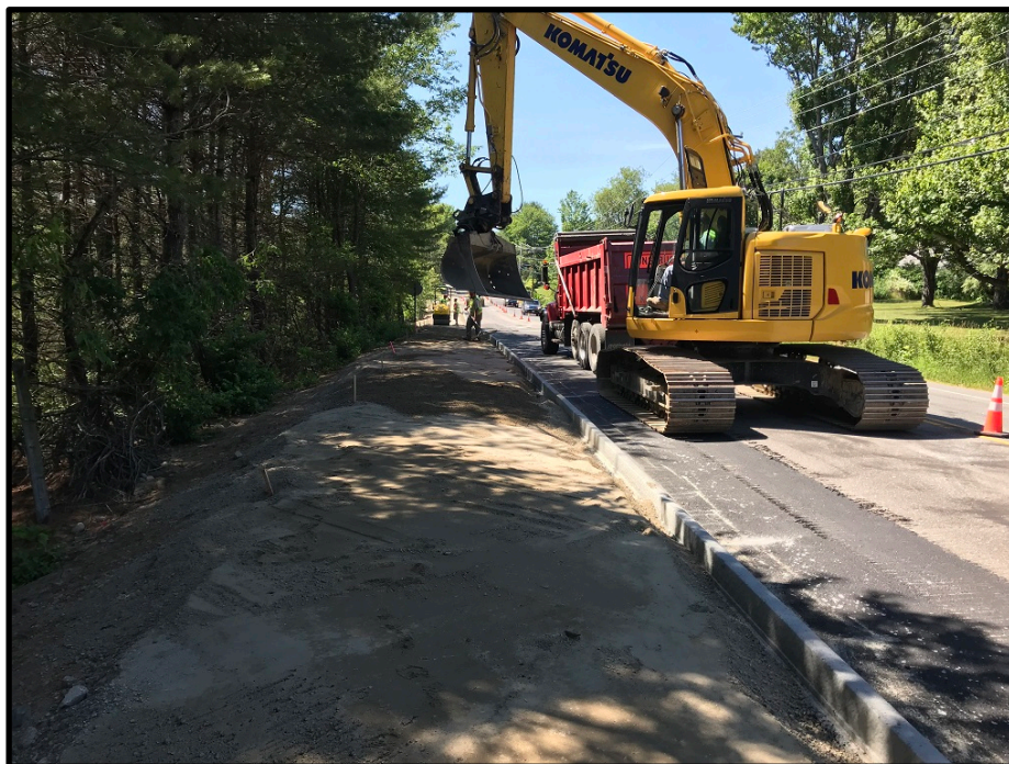
Photograph 4 - Friday, Friday 15 th – Placing and grading gravel on sidewalk near rail road tracks
