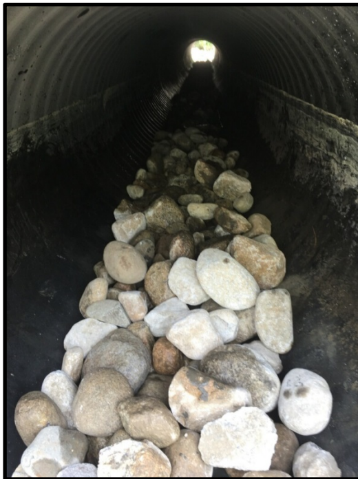
Photograph 10 - Wednesday, June 27 th – Dual 36 inch in culverts imbedded
