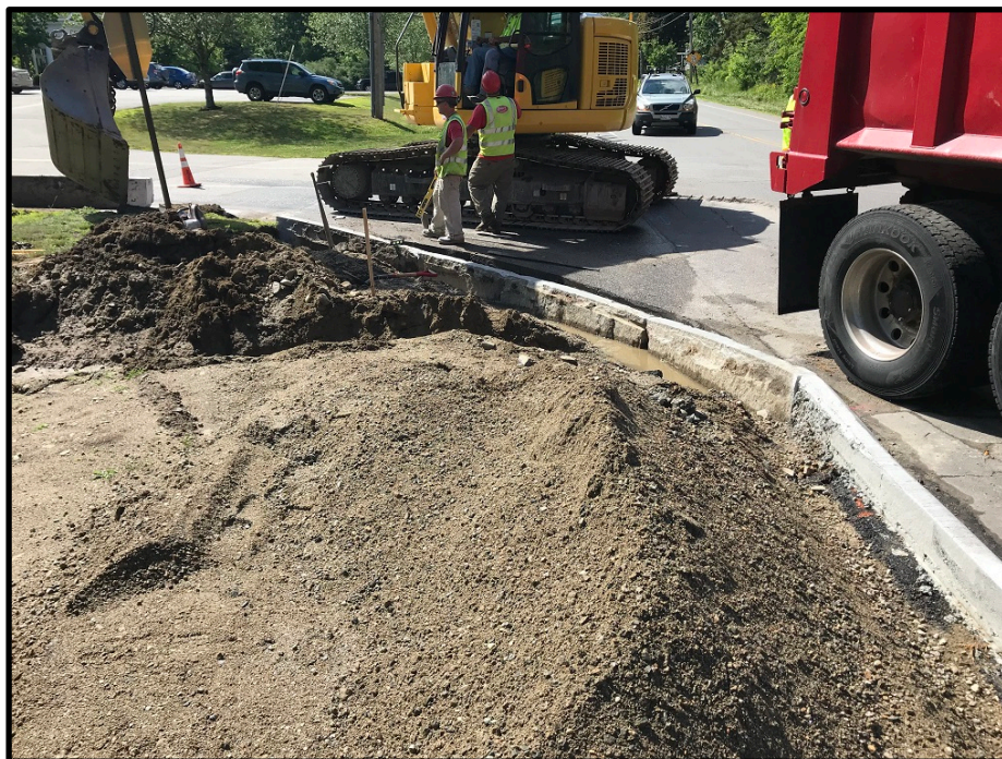
Photograph 6 - Monday, June 25 th – Removing and resetting granite curb at Town Hall
