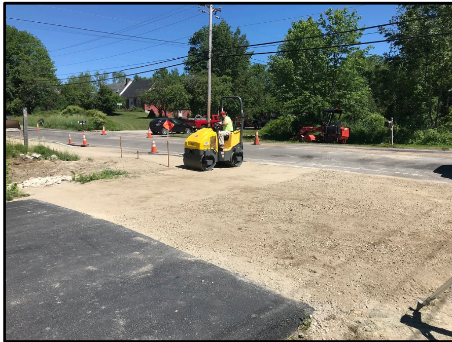
Photograph 3 - Friday, June 22 nd – Rolling gravel in driveway of 272 Tuttle Road
