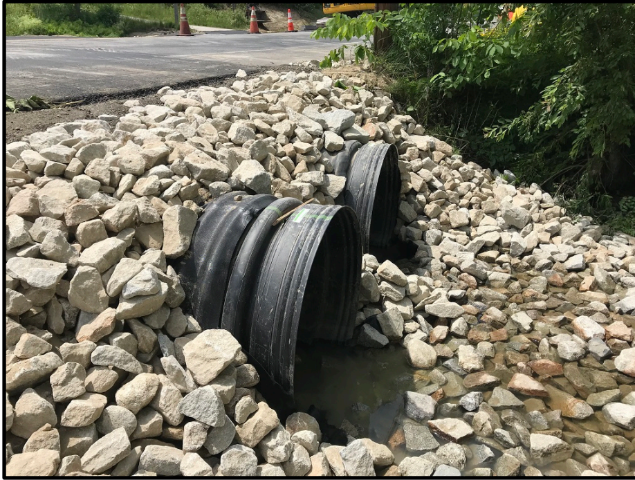
Photograph 9 - Wednesday, June 27 th – Rip rap inlet for dual 36 inch culverts
