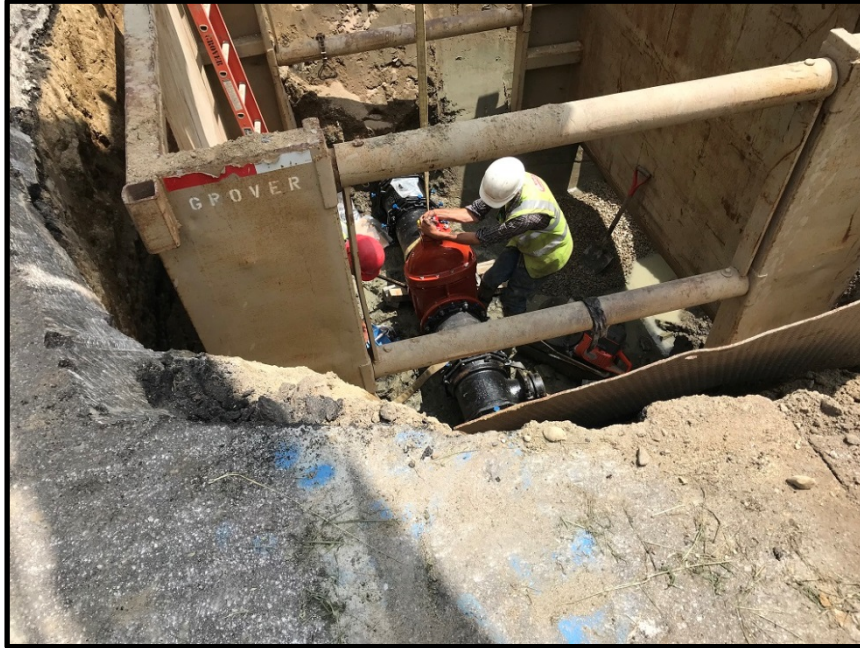
Photograph 1 – Thursday, June 21 st – Installing 12 inch gate valve for eventual water main replacement on west side of limit of work
