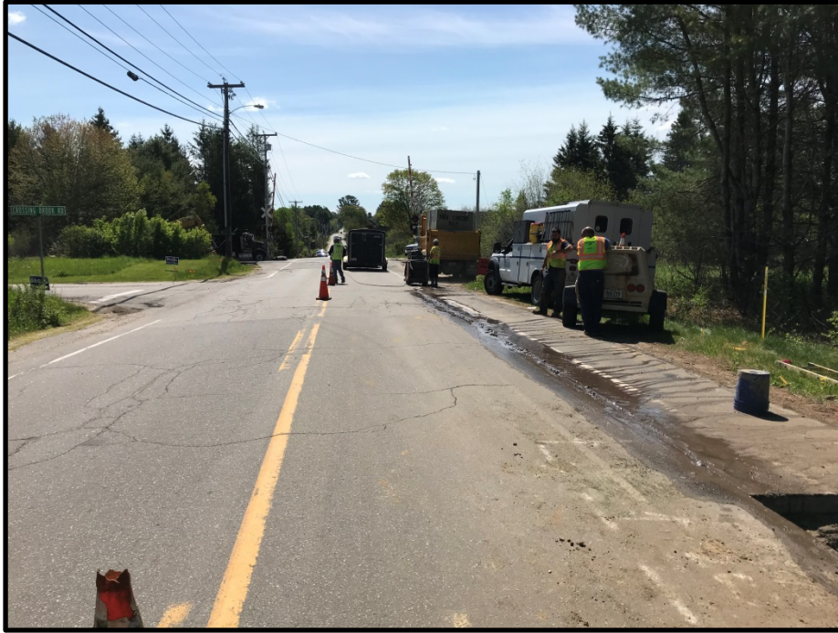
Photograph 9 - Wednesday, May 23 th – Saw cutting pavement for curb installation
