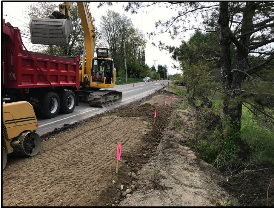
Photograph 7 - Tuesday, May 22 th – Placing subgrade material for sidewalk extension near rail road tracks
