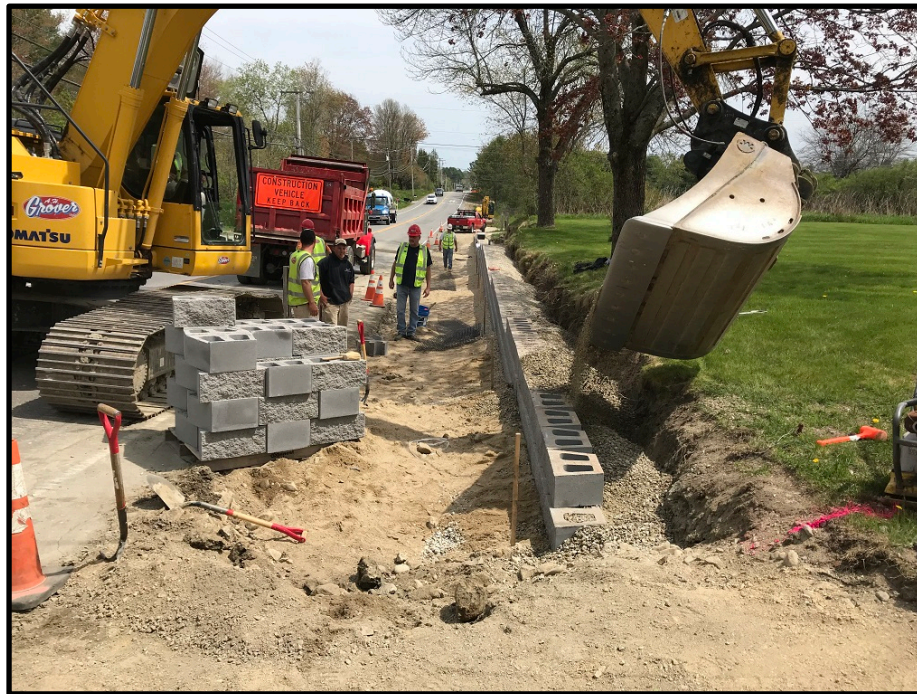
Photograph 2: Thursday, May 17 th – Filling behind block retaining wall in front 280 Tuttle Road
