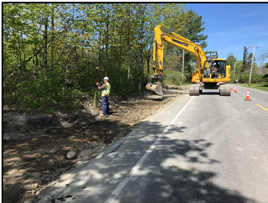
Photograph 4 - Friday, May 18 th – Grading for sidewalk subgrade
