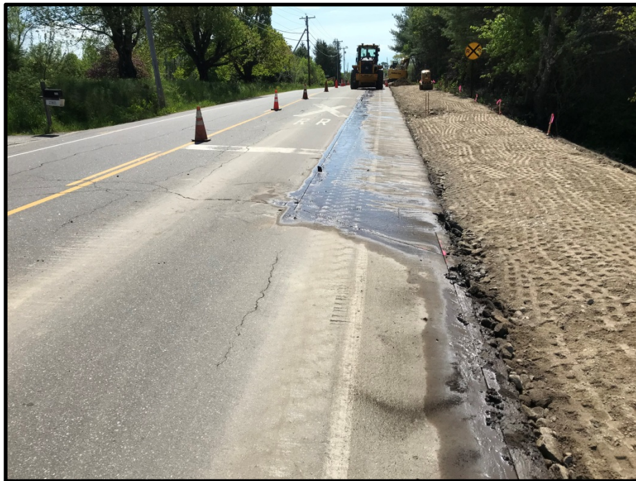
Photograph 10 - Wednesday, May 23 th – Saw cutting pavement for curb installation Road
