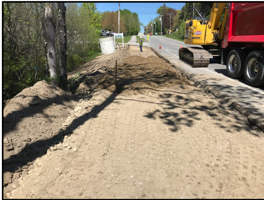
Photograph 5 - Monday, May 21 th – Working on subgrade for sidewalk extension near Town Hall
