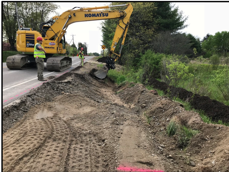
Photograph 8 - Tuesday, May 22 th – Excavating for sidewalk extension near rail road tracks
