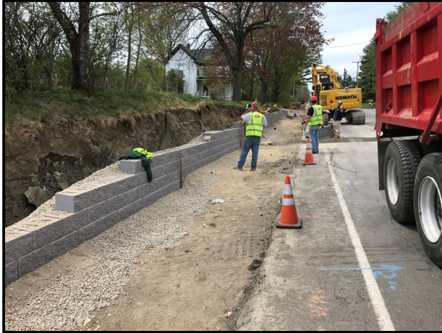
Photograph 1 – Thursday, May 17 th – Constructing block retaining wall in front of 280 Tuttle Road
