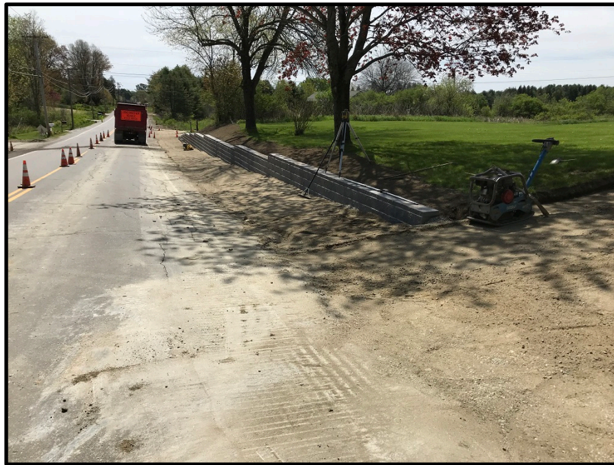
Photograph 3 - Friday, May 18 th – Completed block retaining wall in front of 280 Tuttle Road
