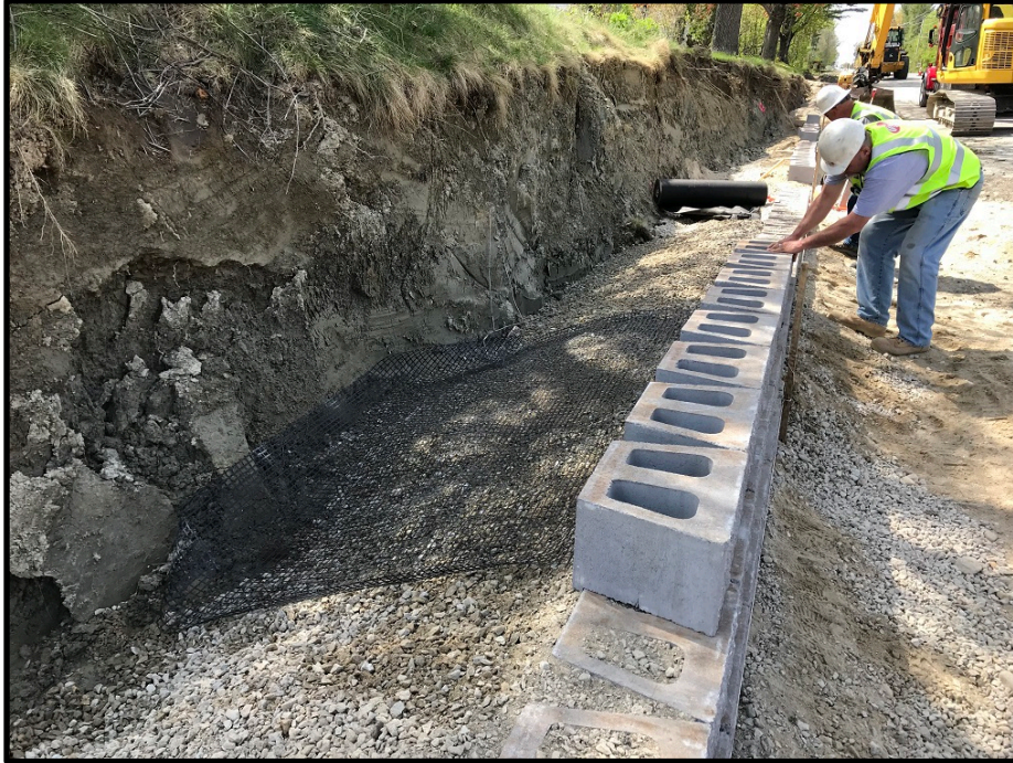
Photograph 9 - Wednesday, May 16 th – Constructing block retaining wall in front of 280 Tuttle Road
