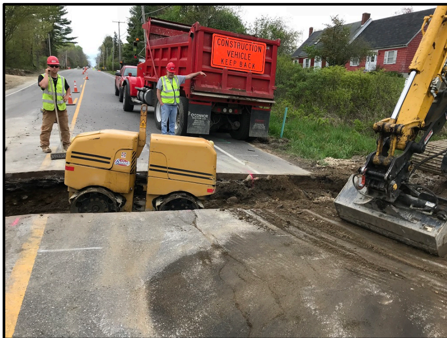
Photograph 8 - Tuesday, May 15 th – Compacting cross trench at field inlet 2
