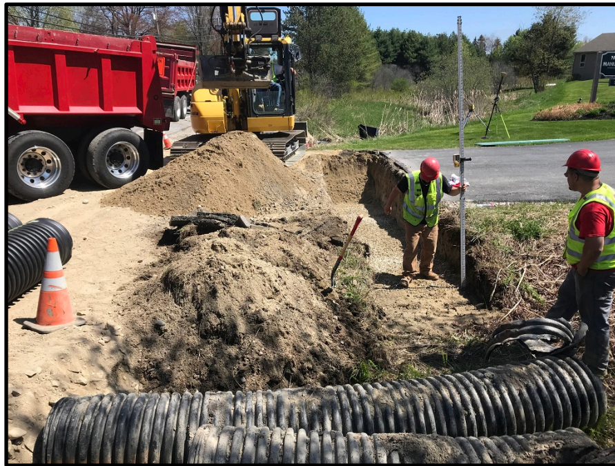
Photograph 5 - Monday, May 14 th – Installing 18 inch HDPE driveway culvert at 272 Tuttle Road
