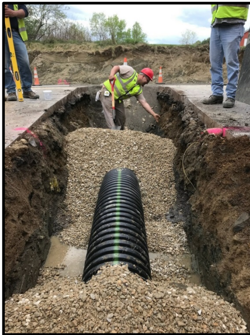
Photograph 7 - Tuesday, May 15 th – 15 inch cross pipe out of drain manhole 1 toward field inlet 2
