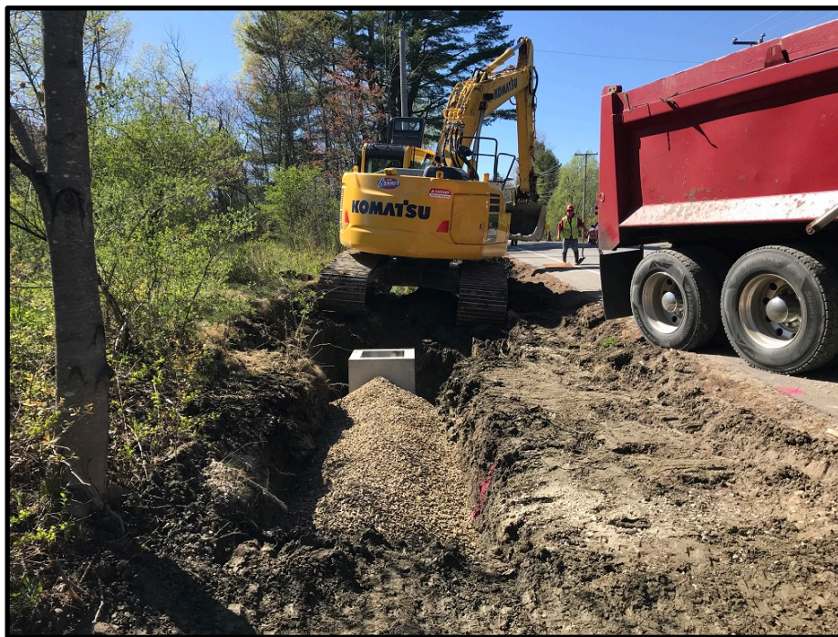
Photograph 4 - Friday, May 11 th – Field inlet 1 installed and 15 inch HDPE connected to it
