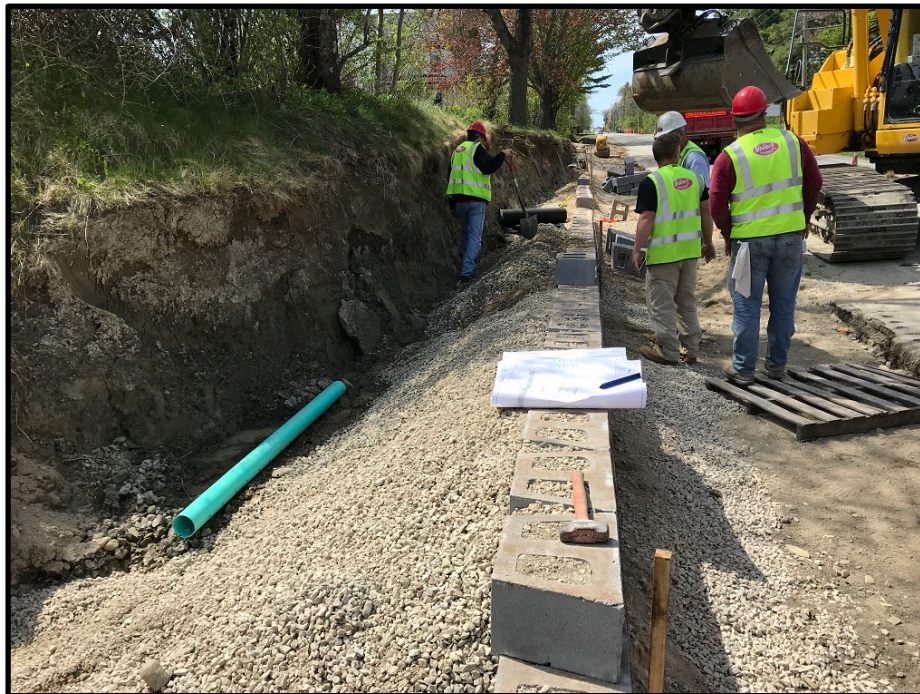
Photograph 10 - Wednesday, May 16 th – Constructing block retaining wall in front of 280 Tuttle Road
