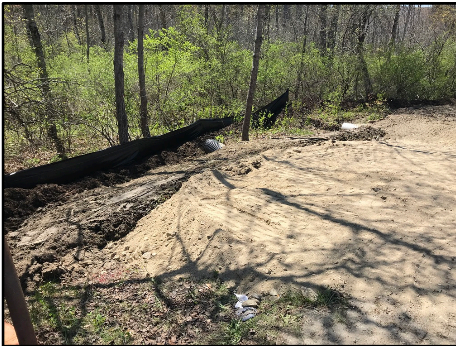
Photograph 6 - Monday, May 14 th – Catch basin1 with 15 inch HDPE outlet pipe
