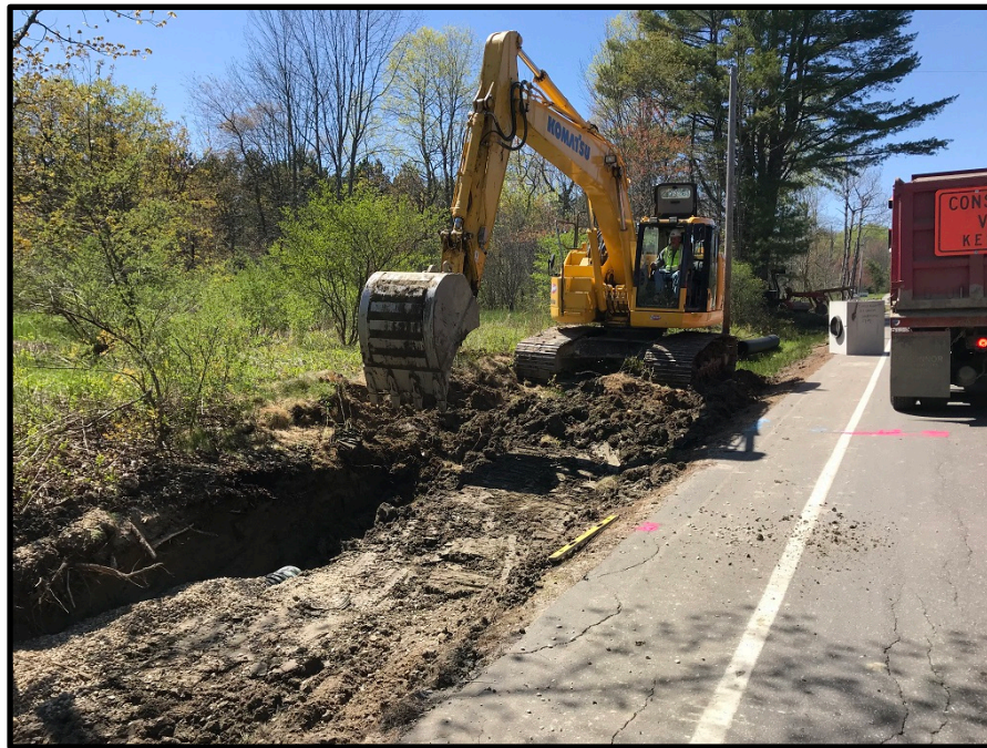
Photograph 3 - Friday, May 11 th – Excavating for field inlet 1
