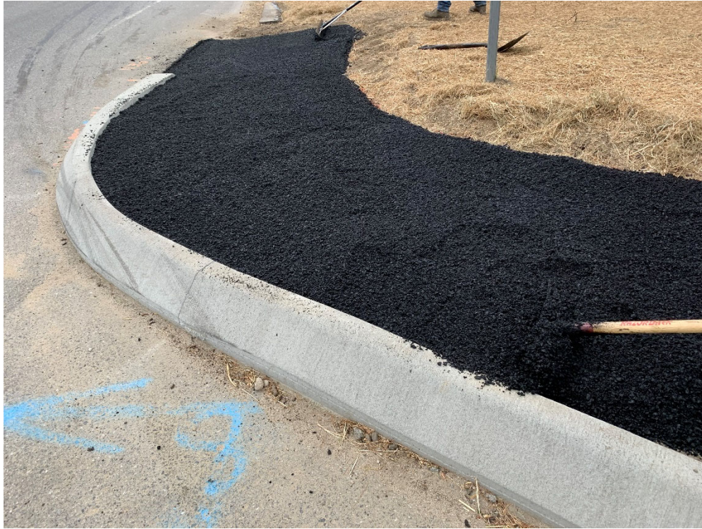
Photo 9 – Placement of 9.5 mm pavement at sidewalk entrance to Crossing Brook Road, looking west.
