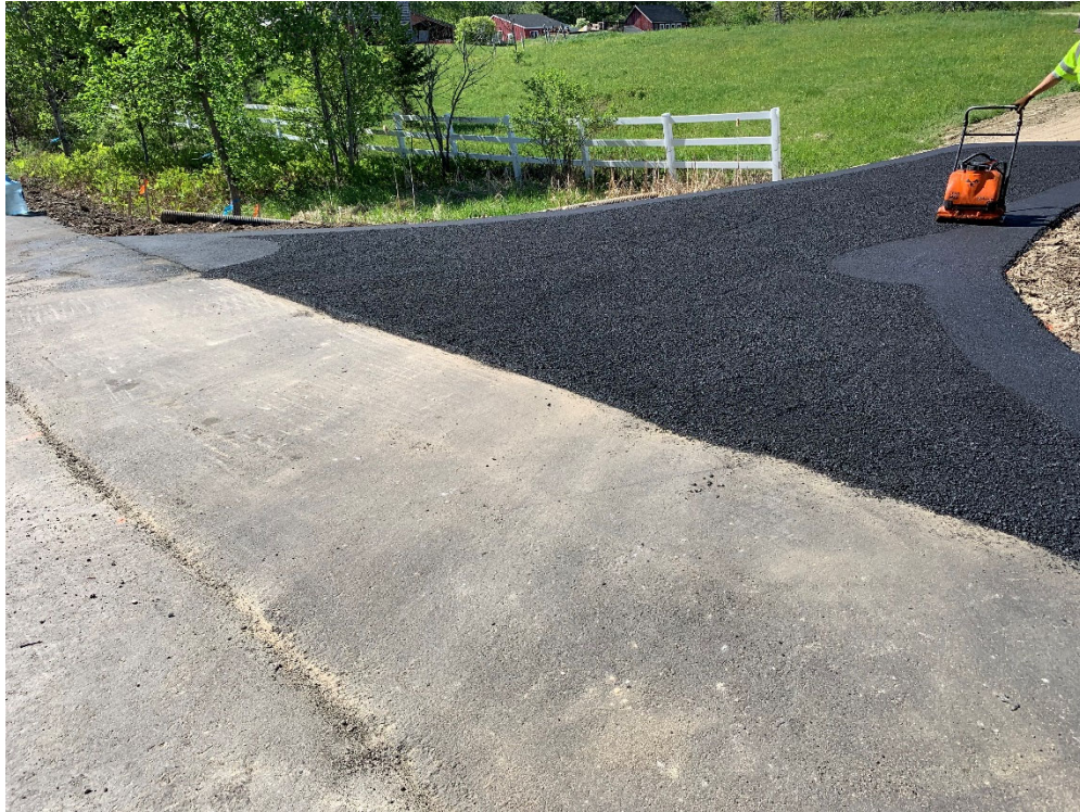
Photo 3 – Compaction of 9.5 mm pavement at entrance to 198 Tuttle Road, looking south.
