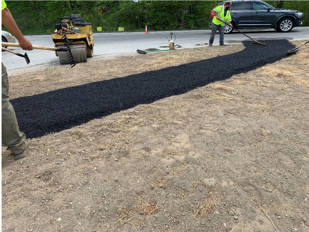
Photo 7 – Placement of 9.5 mm pavement at sidewalk entrance to Twin Brooks, looking southwest.
