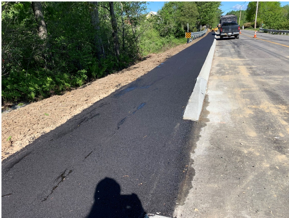
Photo 2 – Placed and compacted 12.5 mm pavement at approximate STA 19+00, looking northwest.
