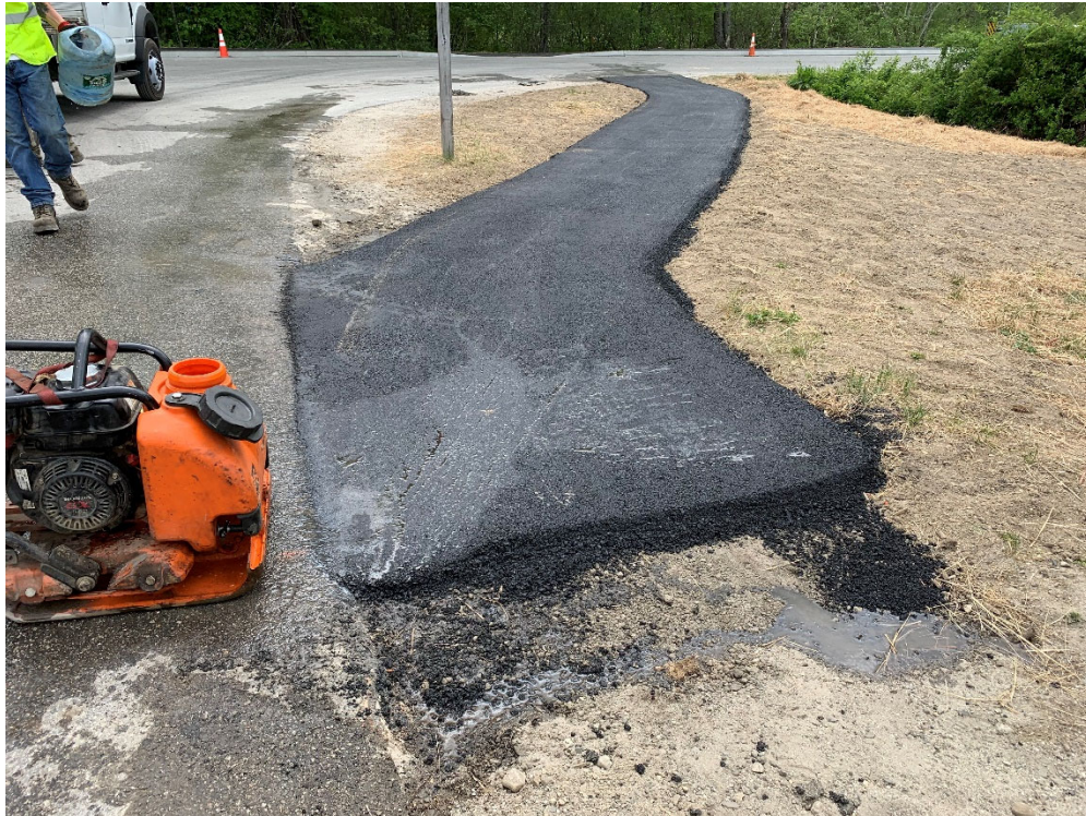
Photo 8 – Compacted pavement at sidewalk entrance to Twin Brooks, looking southwest.
