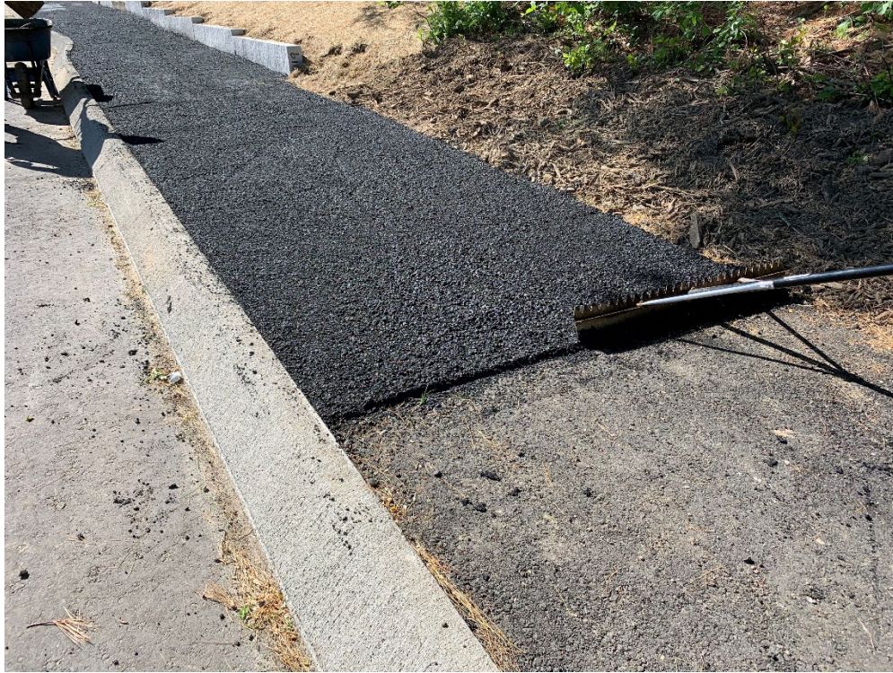
Photo 1 – Placed 12.5 mm pavement at approximate STA 14+00, looking southeast.
