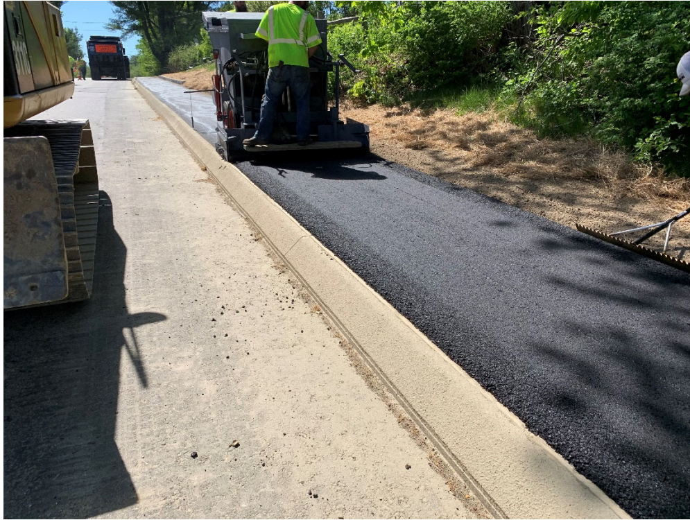
Photo 5 – Placement of 9.5 mm pavement at approximate STA 0+50, looking southeast.
