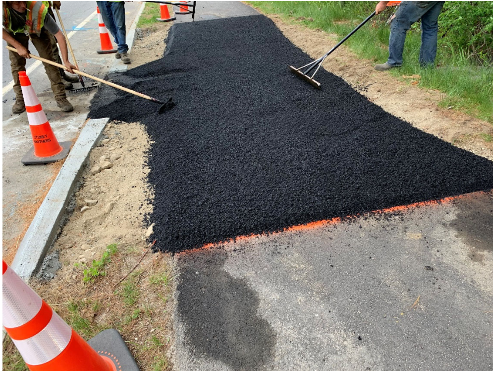
Photo 10 – Placement of 9.5 mm pavement at sidewalk ramp to Crossing Brook Road, looking southeast.
