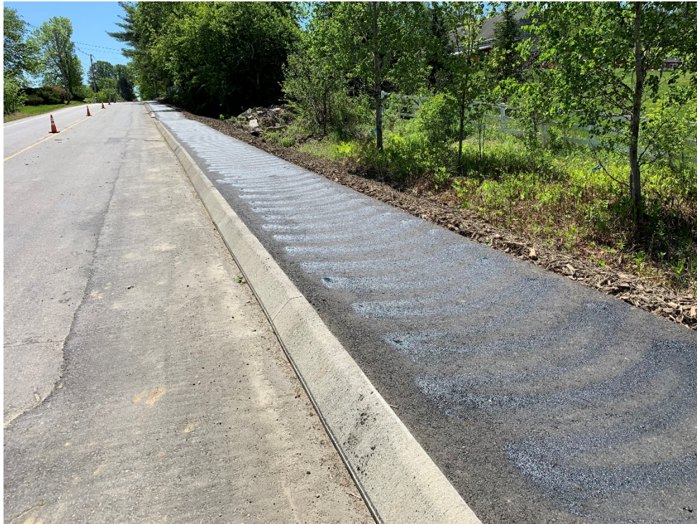
Photo 4 – Tacked binder pavement at approximate STA 12+00, looking southeast.
