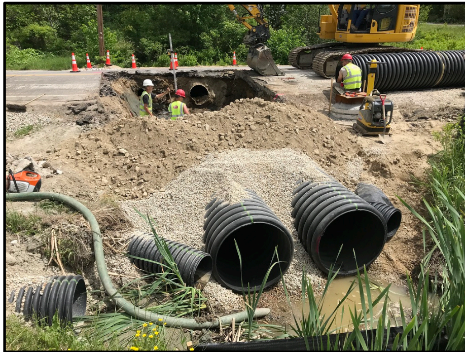
Photograph 2: Wednesday, June 13 th – Installing first two sections of 36 inch HDPE dual culverts
