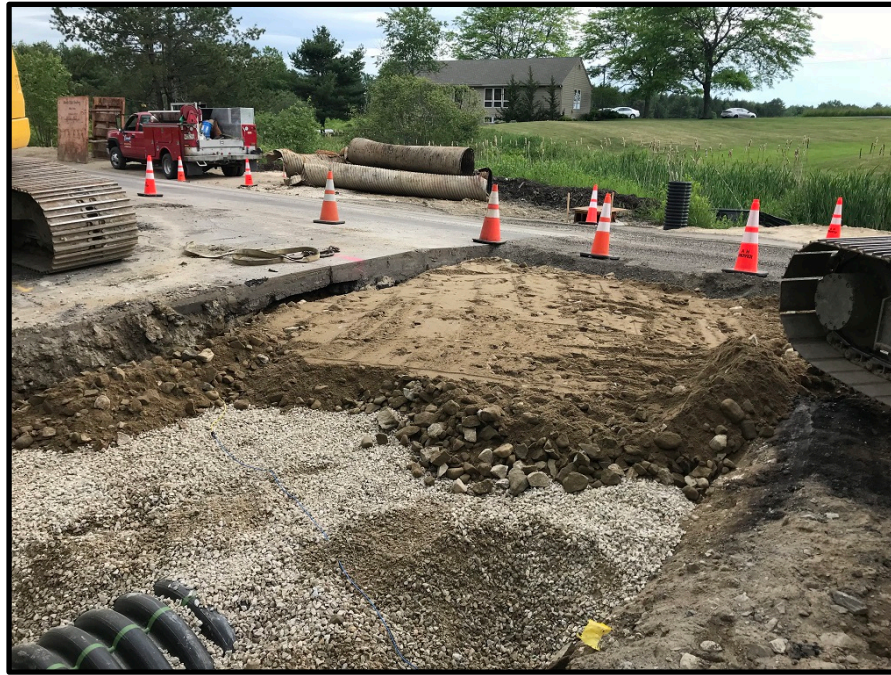
Photograph 3 - Wednesday, June 13 th – Backfilling 36 inch HDPE dual culverts
