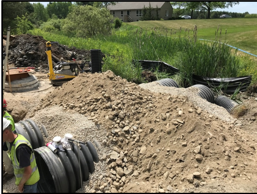
Photograph 1 – Wednesday, June 13 th – Installing first two sections of 36 inch dual culverts
