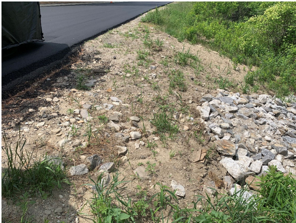
Photo 12 – Disturbed material around the drainage pipe riprap apron adjacent to 225 Tuttle Road, looking northwest.
