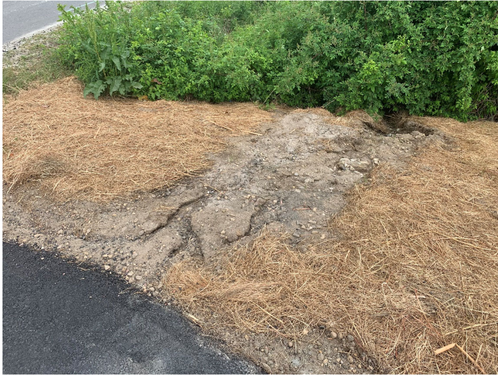
Photo 11 – Erosion rills adjacent to Twin Brook sidewalk entrance, looking northwest.
