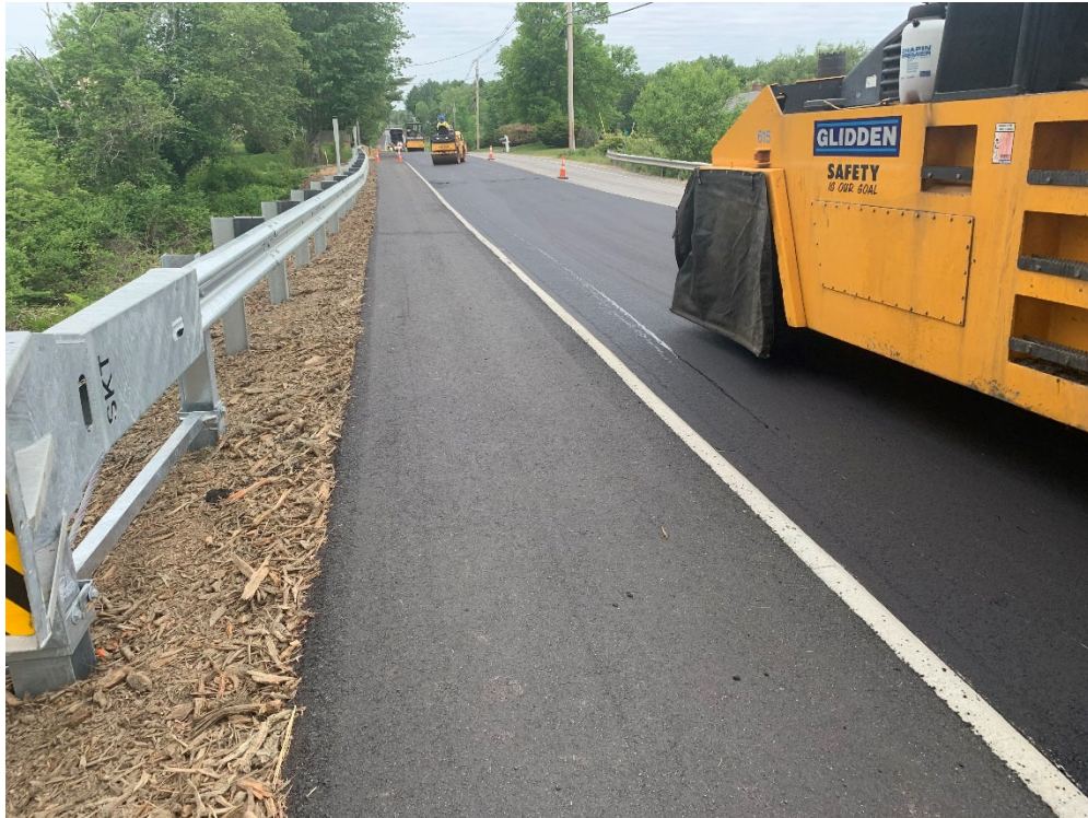
Photo 6 – Roll compaction of surface pavement in southeast lane near 186 Tuttle Road, Looking northwest.
