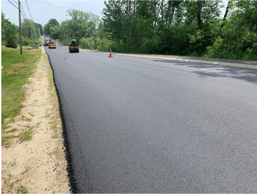
Photo 9 – Compacted surface pavement in northwest lane near 215 Tuttle Road, looking southeast.
