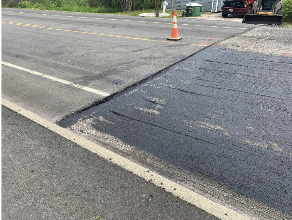
Photo 1 – Tacked pavement joint and surface on southeast travel lane near PWD Sewer Pump Station, looking north.
