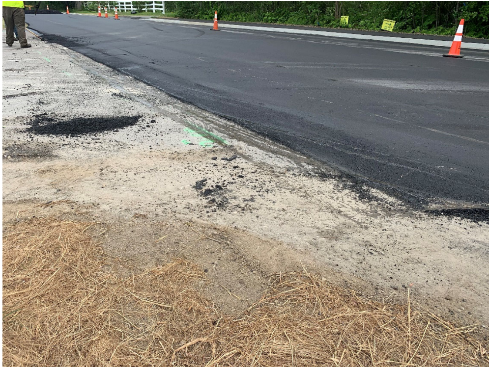
Photo 10 – Surface pavement placement and compaction in Twin Brook entrance joint, looking southeast.
