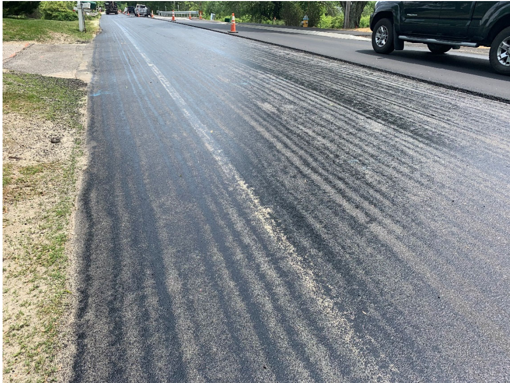
Photo 2 – Tacked existing southeast lane road surface near 197 Tuttle Road, looking southeast.
