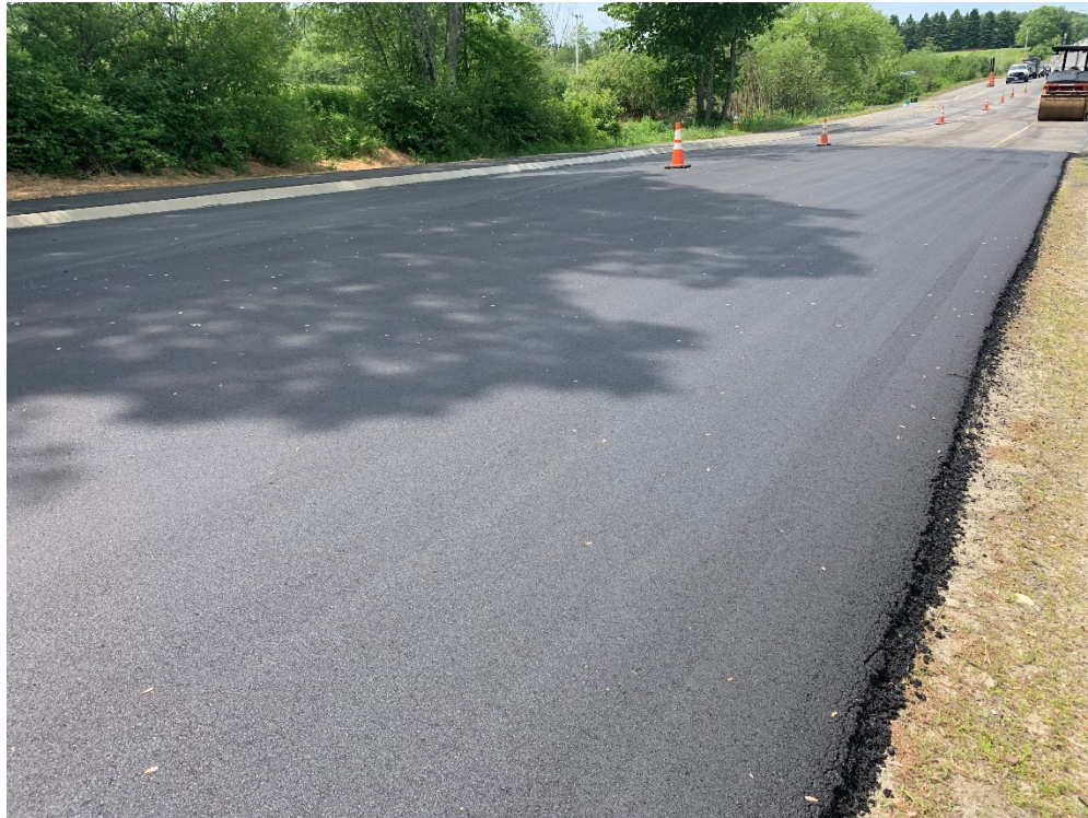
Photo 8 – Compacted surface pavement in northwest travel lane near 225 Tuttle Road, looking northwest.
