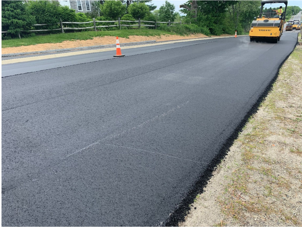
Photo 5 – Roll compaction of surface pavement in northwest lane near 224 Tuttle Road, looking northwest.
