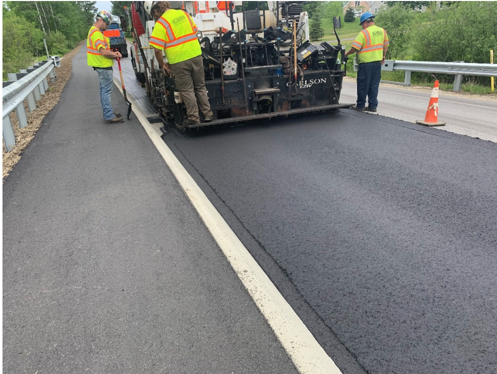
Photo 4 – Surface pavement placement on northwest lane near 12-foot diameter culvert crossing, looking northwest.
