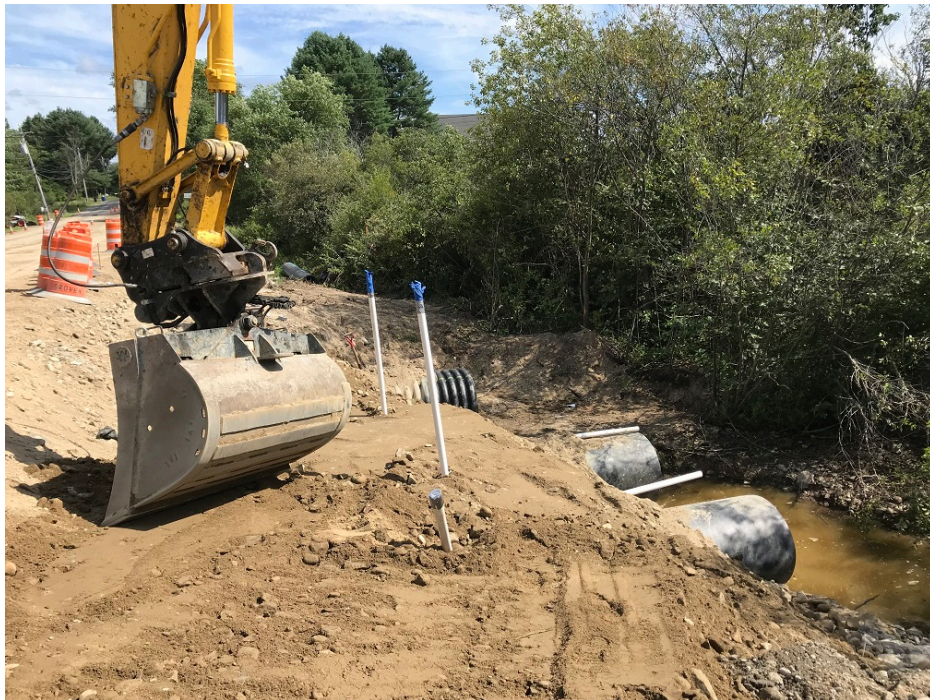
Photo 4 – PVC ports for grouting
