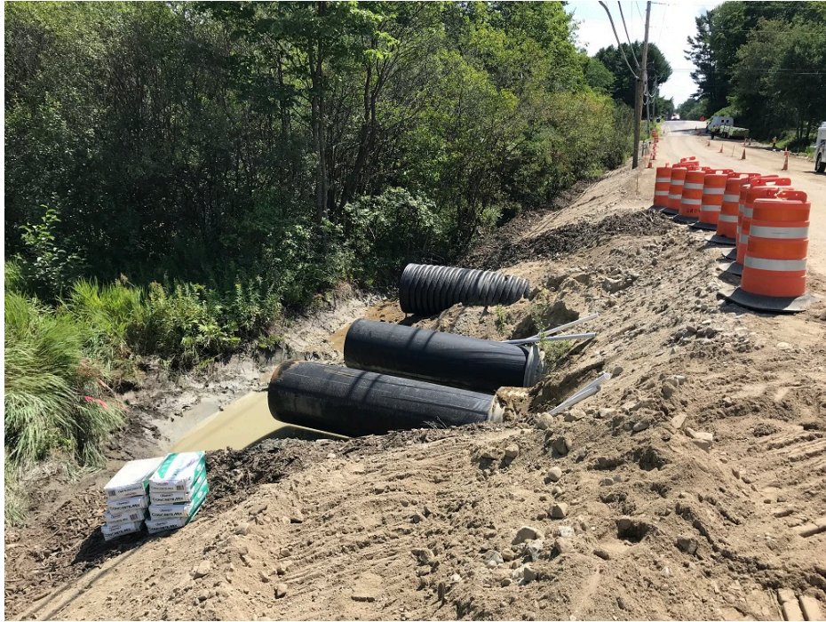
Photo 1 – Slip line culverts installed STA 9+75
