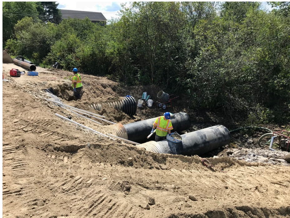
Photo 2 – Placing mortar around void at end of existing culverts
