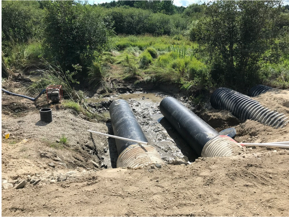
Photo 3 – Slip lined culverts STA 7+00
