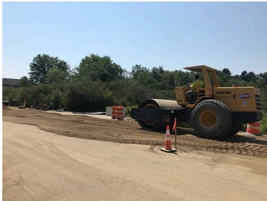
Photo 2 – Compacting base gravel
