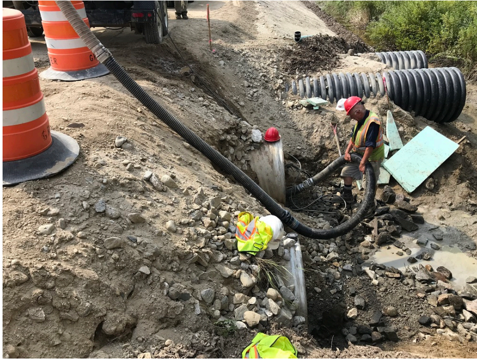
Photo 3 – Cleaning existing cross culverts approximate STA 7+50
