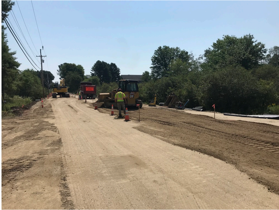
Photo 1 – Placing and grading base gravel
