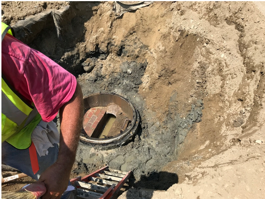
Photo 4 – Cone section taken off so barrel section could be added
