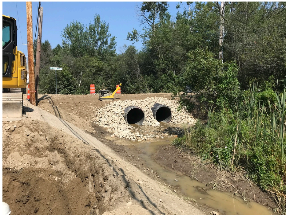
Photo 2 – Rip rap around culverts at Bunkers Way
