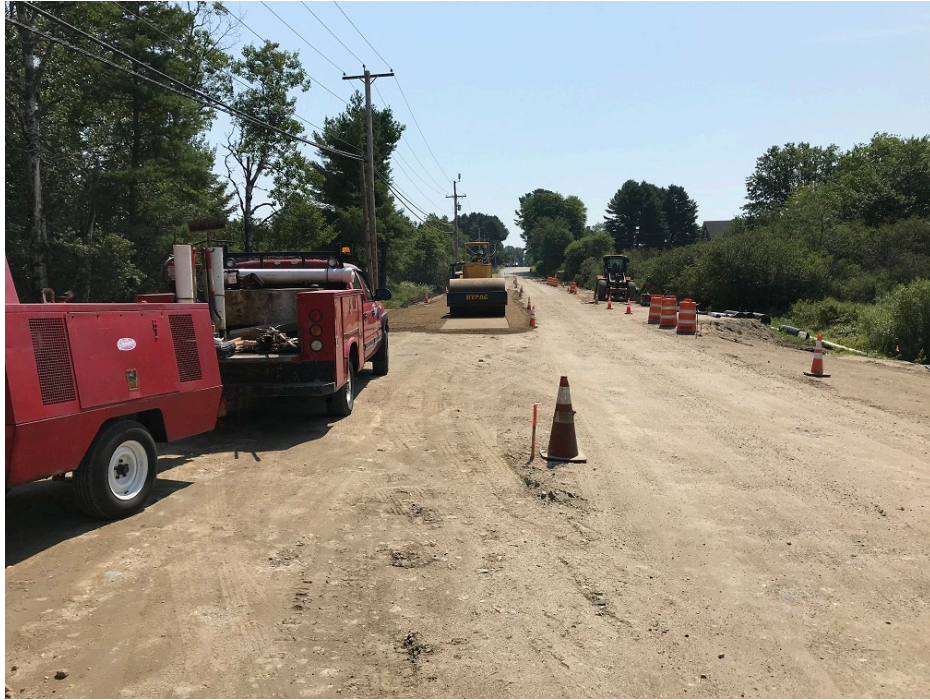
Photo 3 – Compacting base gravel
