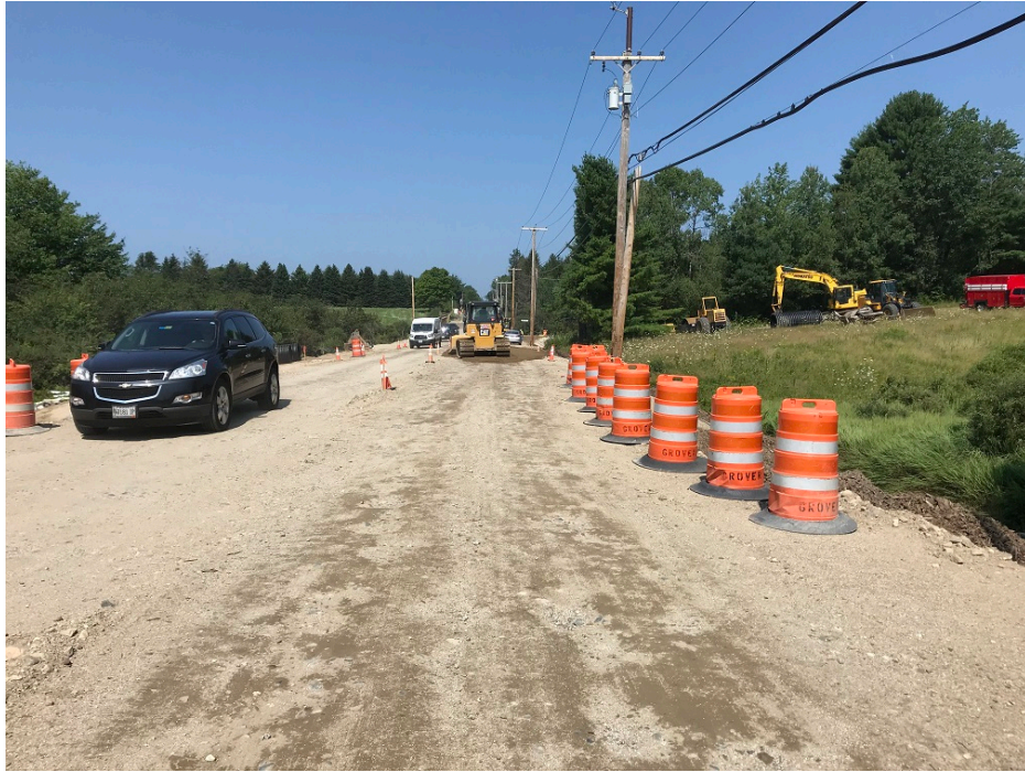
Photo 1 – Placing and grading base gravel
