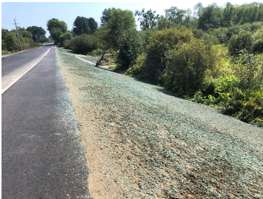
Photo 3 – Hydroseed installation, STA 6+00 looking east
