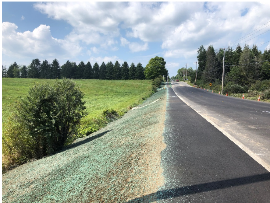
Photo 2 – Hydroseed installation, STA 6+00 looking west
