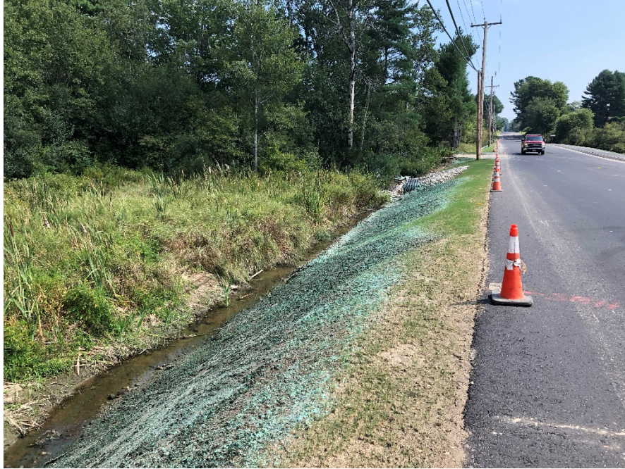
Photo 1 – Stabilized embankment repairs, STA 5+00, It.
