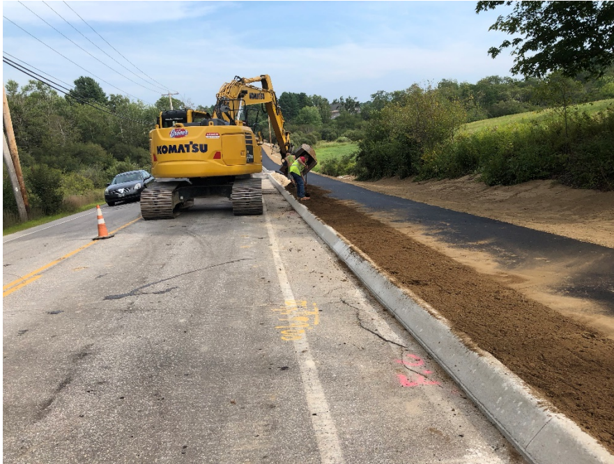
Photo 5 – Installing loam at esplanade, STA 2+00
