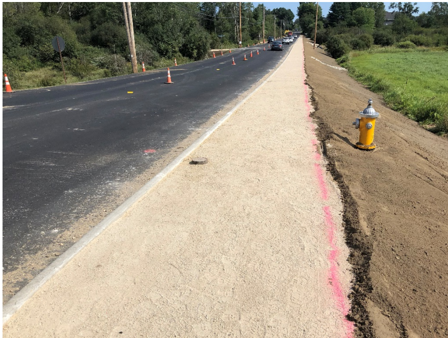
Photo 4 – Sidewalk base, STA 3+28, rt
