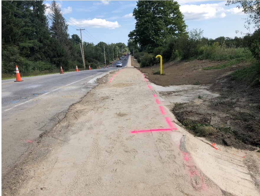
Photo 3 – Sidewalk base, STA 0+00, rt.
