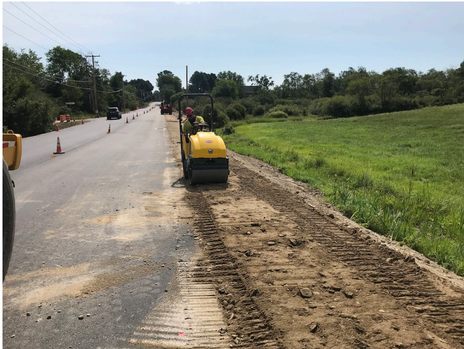
Photo 1 – Compacting subbase gravel for sidewalk
