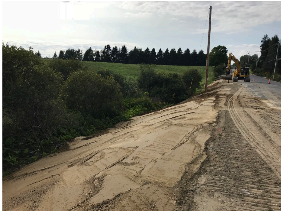
Photo 4 – Placing topsoil on back slope at north side of Tuttle Road
