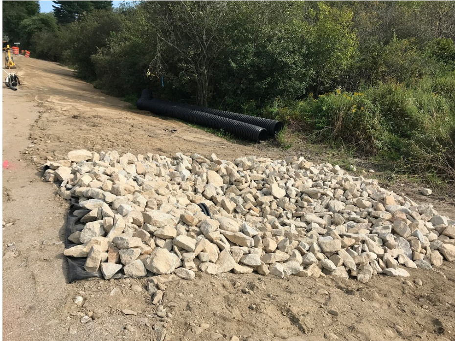
Photo 3 – Placed rip rap for storm drain outlet
