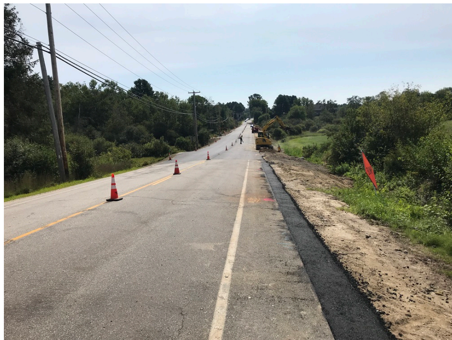
Photo 2 – Placing subbase gravel for sidewalk
