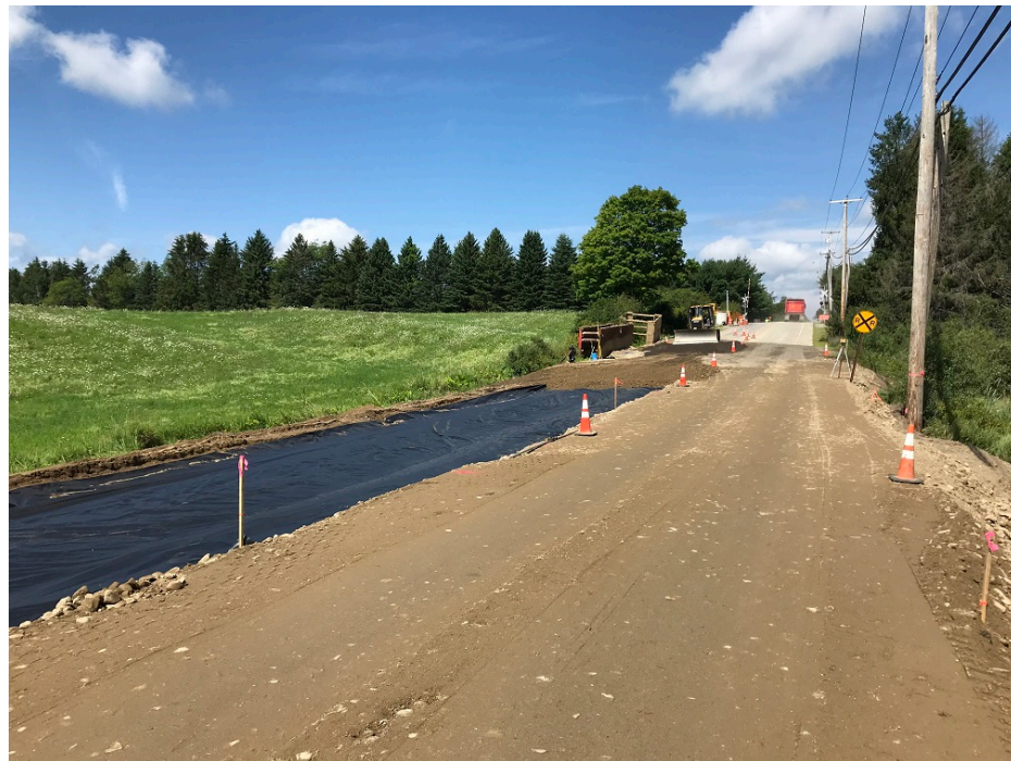
Photo 2 – Placing fabric and gravel at east end of project area
