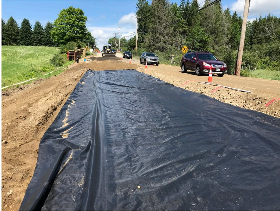
Photo 3 – Placing fabric and gravel at east end of project area
