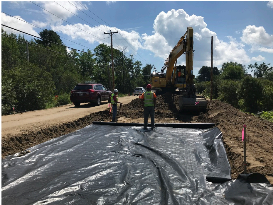
Photo 4 – Excavating for base grade
