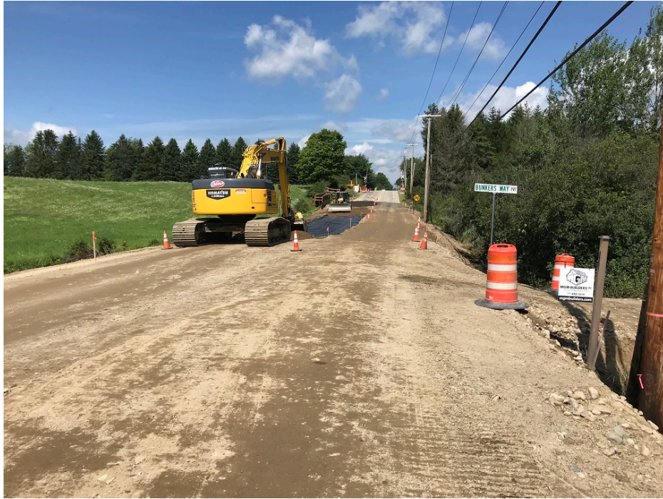
Photo 1 – Working on box cut at east end of the project
