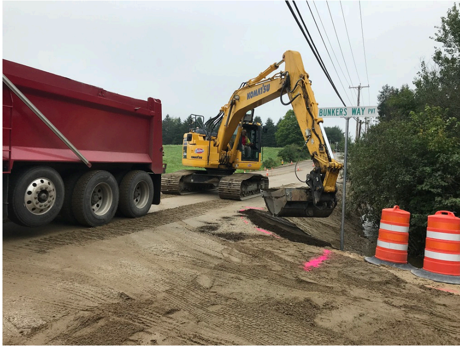
Photo 1 – Placing topsoil near Bunkers Way
