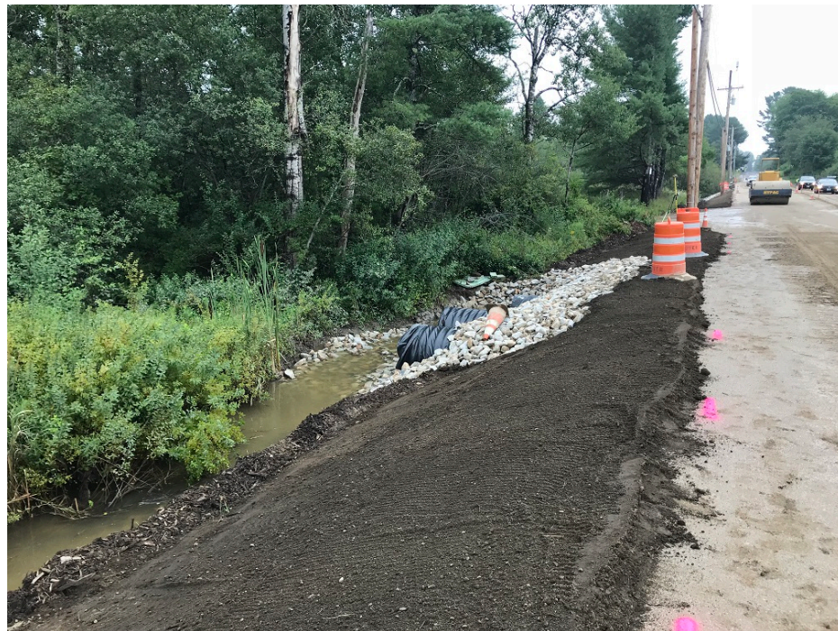
Photo 2 – Placed topsoil
