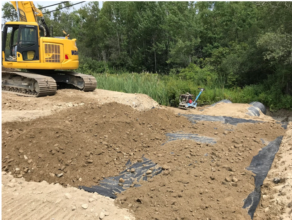
Photo 4 – Replaced fabric and gravel over dual 36 inch culverts at STA 7+00
