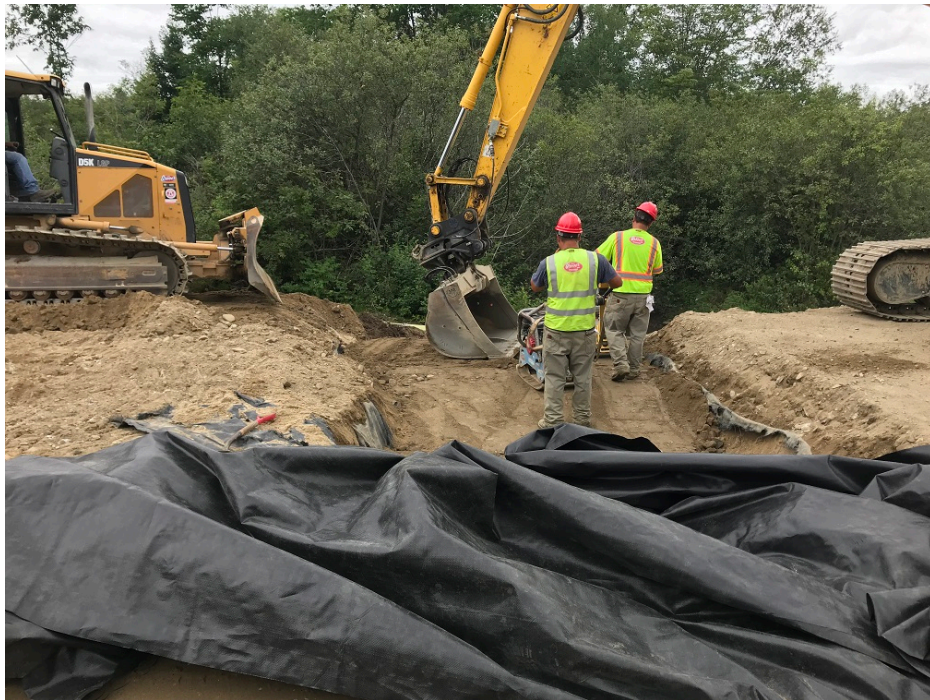
Photo 6 – Backfilling and compacting over 36 inch culvert at approximate STA 9+80
