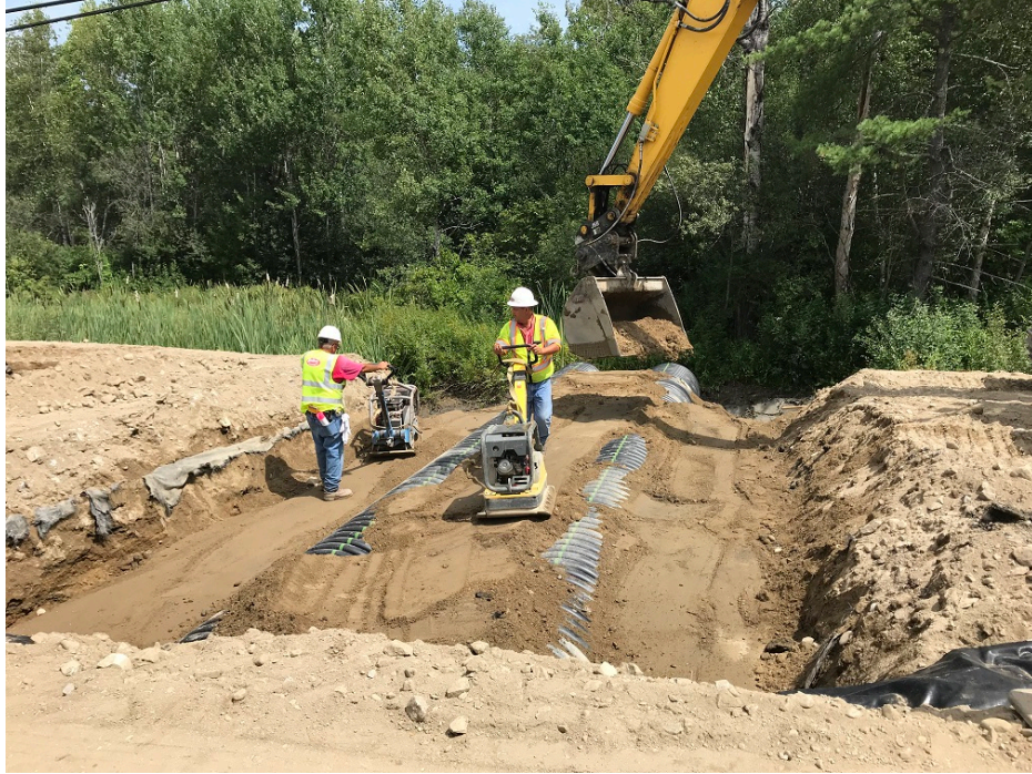
Photo 3 – Placing sand and compacting around dual 36 inch culverts at STA 7+00
