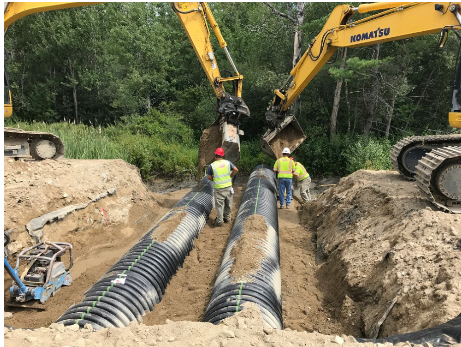
Photo 2 – Placing sand and compacting around dual 36 inch culverts at 7+00
