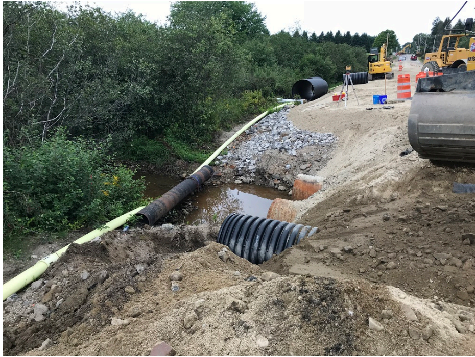
Photo 5 – Outlet for 36 inch culvert at approximate STA 9+80
