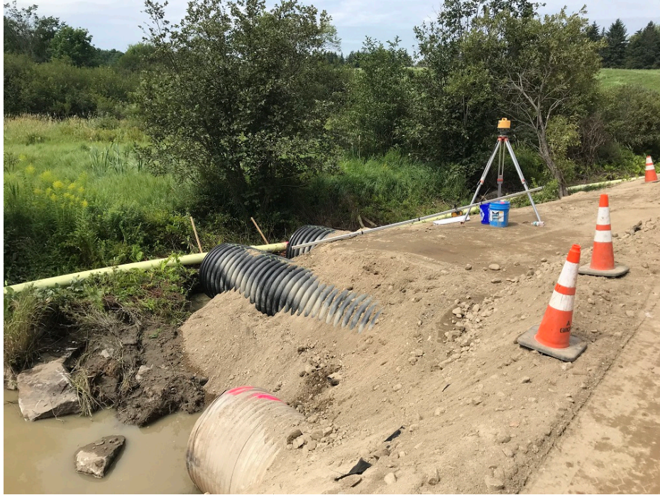
Photo 1 – Outlet for 36 inch culverts at STA 7+00
