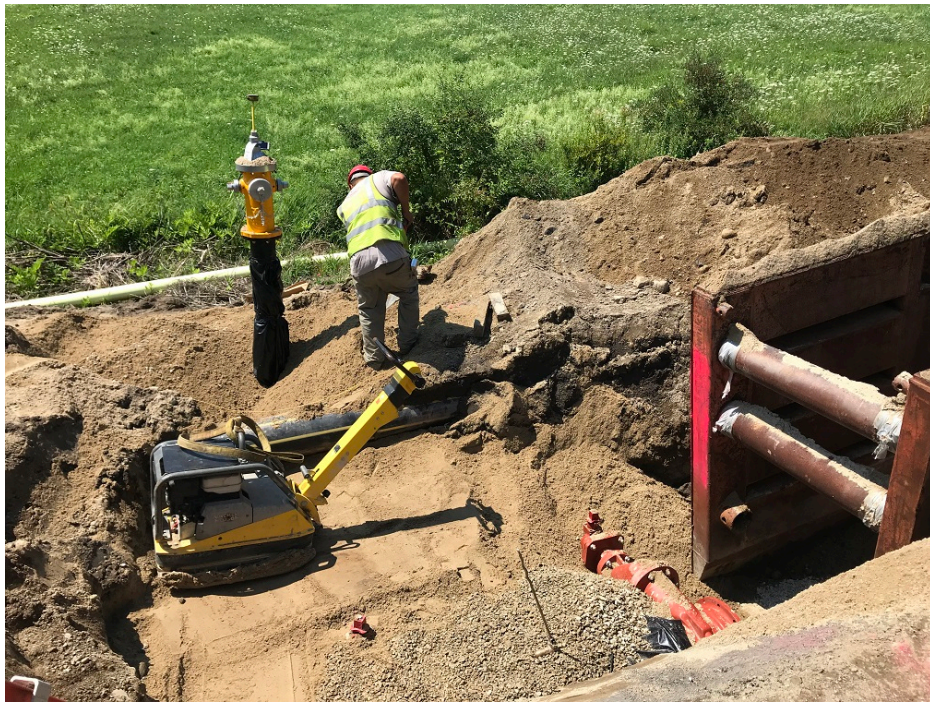
Photo 4 – Backfilling around HYD assembly
