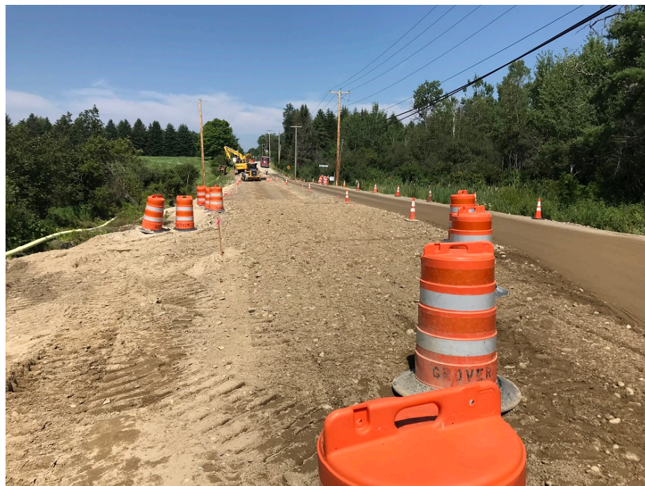
Photo 2 – Placing gravel through fill area of project
