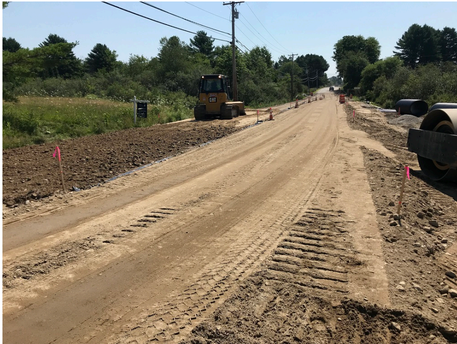
Photo 1 – Placing gravel through fill area of project
