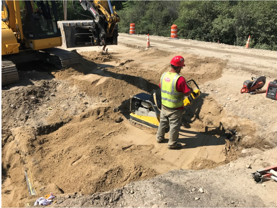
Photo 3 – Compacting sand over water service
