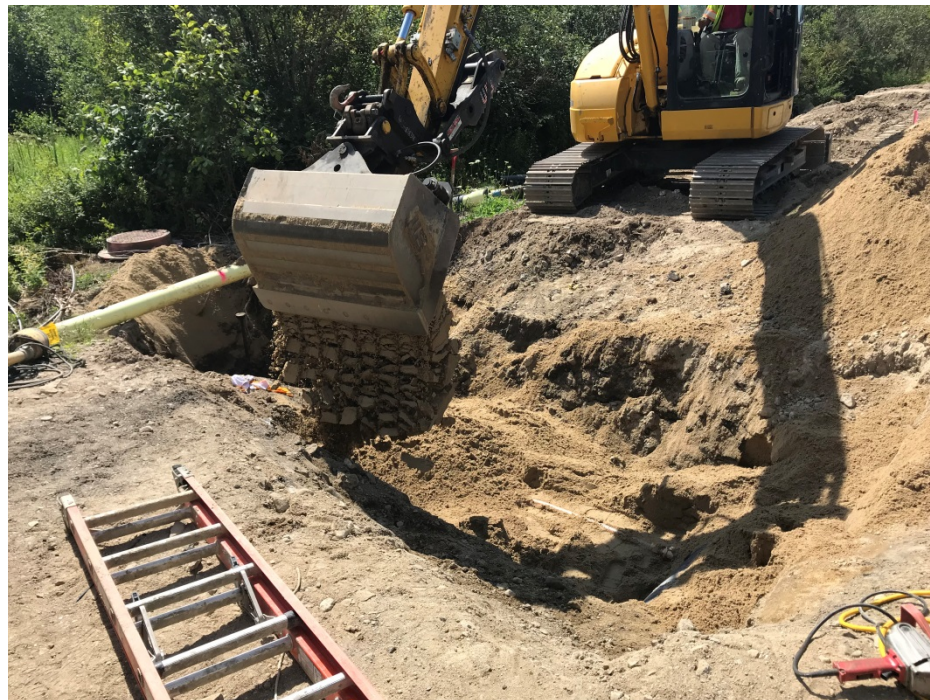
Photo 2 – Placing sand over water service at October Farms Way
