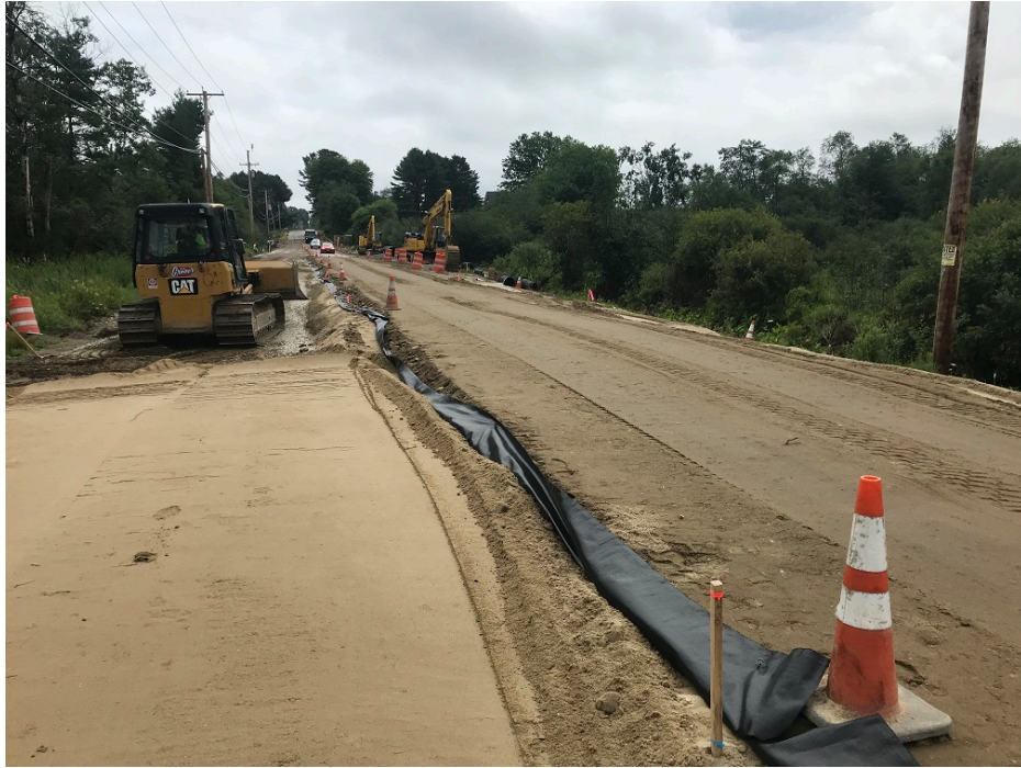
Photo 3 – Placing fill for road reconstruction
