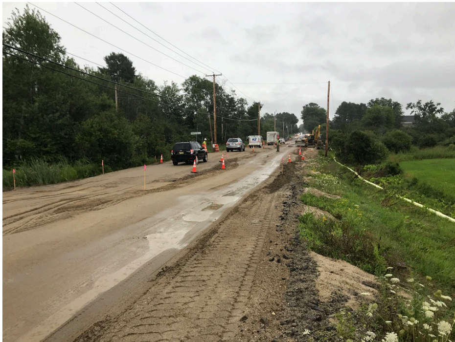
Photo 4 – Placing fill for road reconstruction
