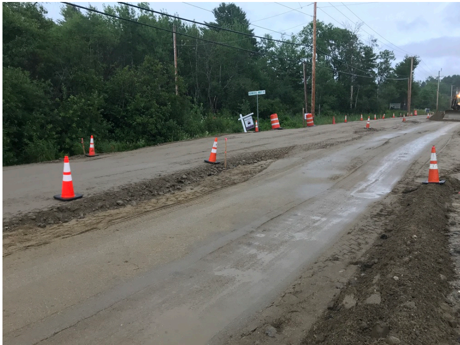
Photo 6 – Placing fill for road reconstruction
