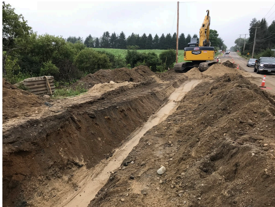
Photo 2 – Compacted sand over 16 inch HDPE water main
