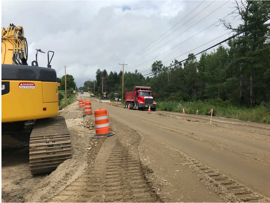
Photo 5 – Placing fill for road reconstruction
