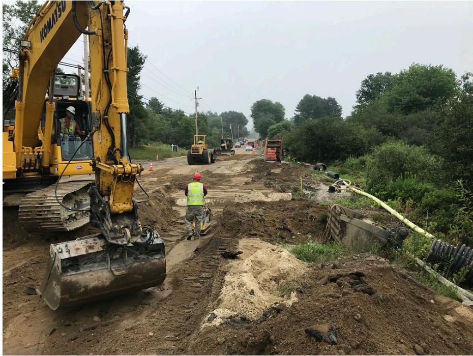
Photo 5 – Compacting the backfill in water main trench
