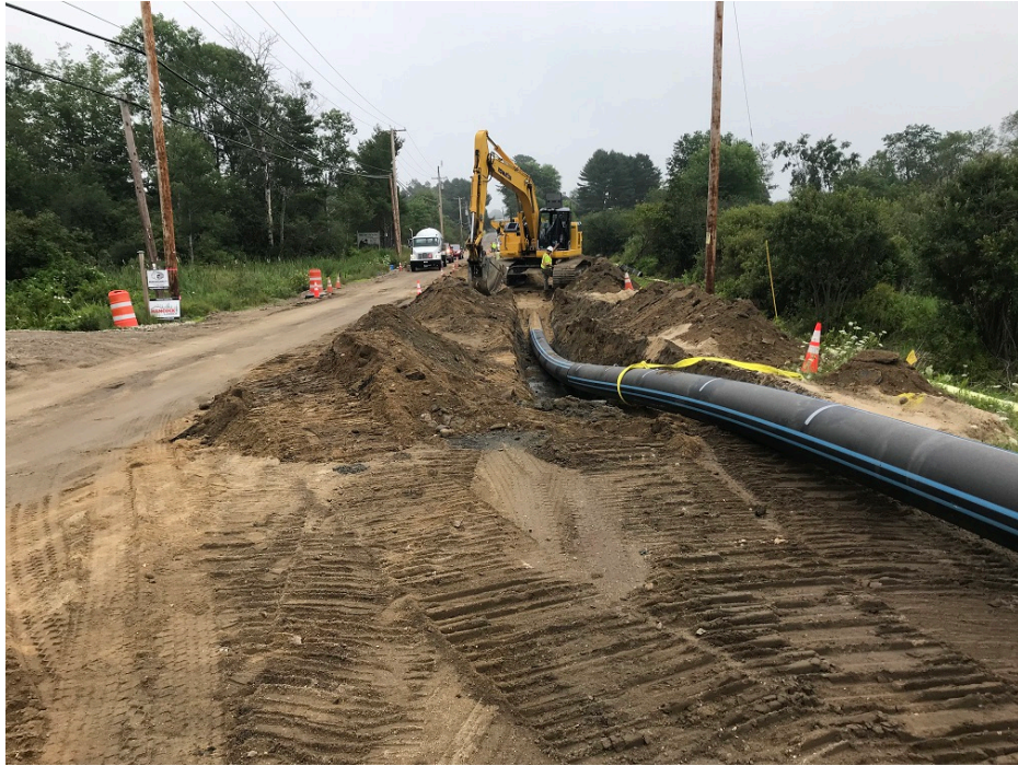
Photo 1 – Backfilling 16 inch HDPE water main
