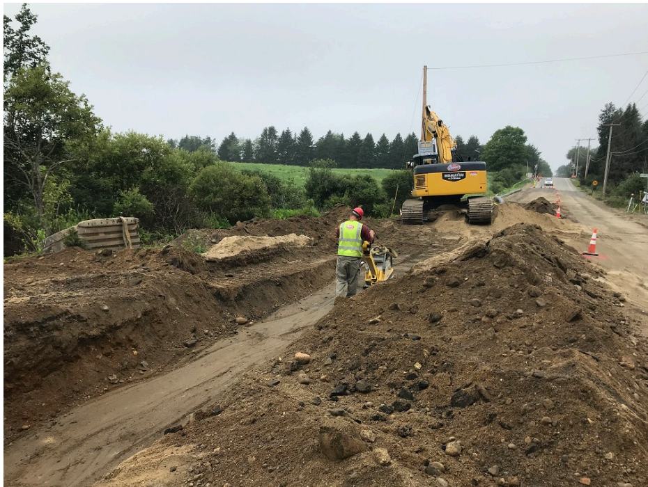
Photo 4 – Compacting the backfill in water main trench
