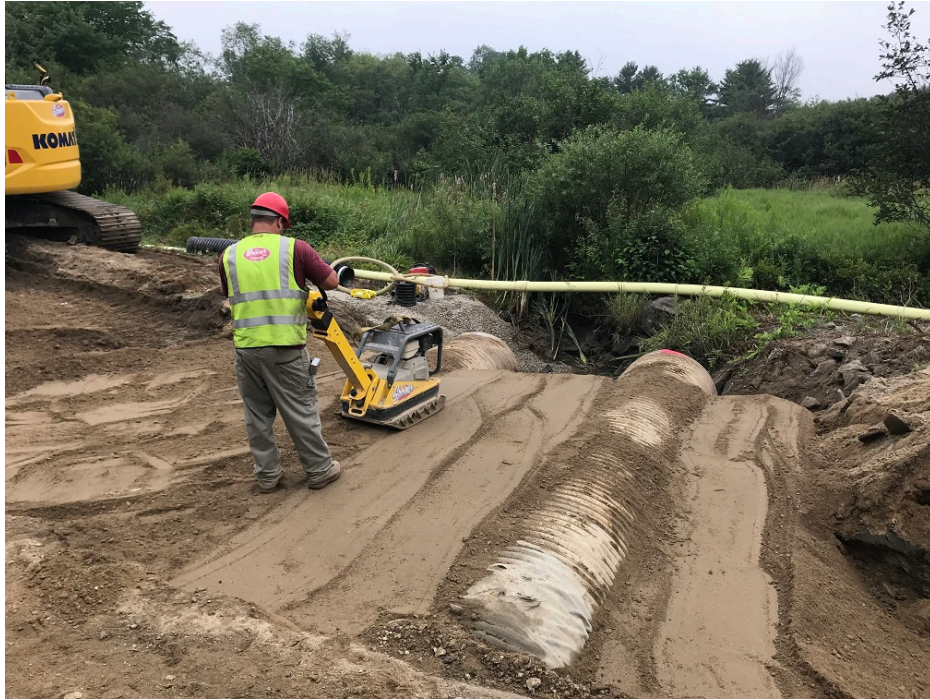
Photo 3 – Compacting gravel around existing 42 inch culverts at STA 7+00
