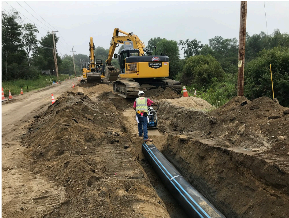
Photo 6 – Compacting the sand over 16 inch HDPE water main
