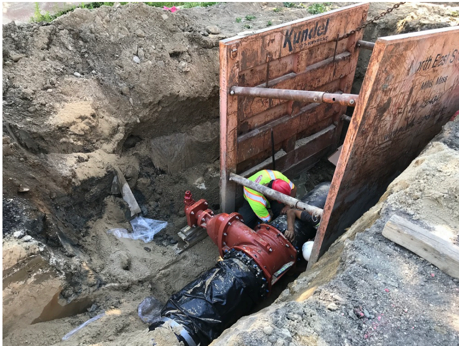
Photo 4 – Hydrant tee and valve
