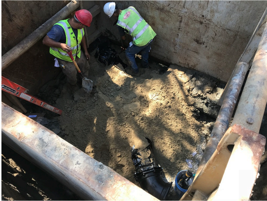
Photo 1 – Placing sand around 45 degree bends on east side of project limits
