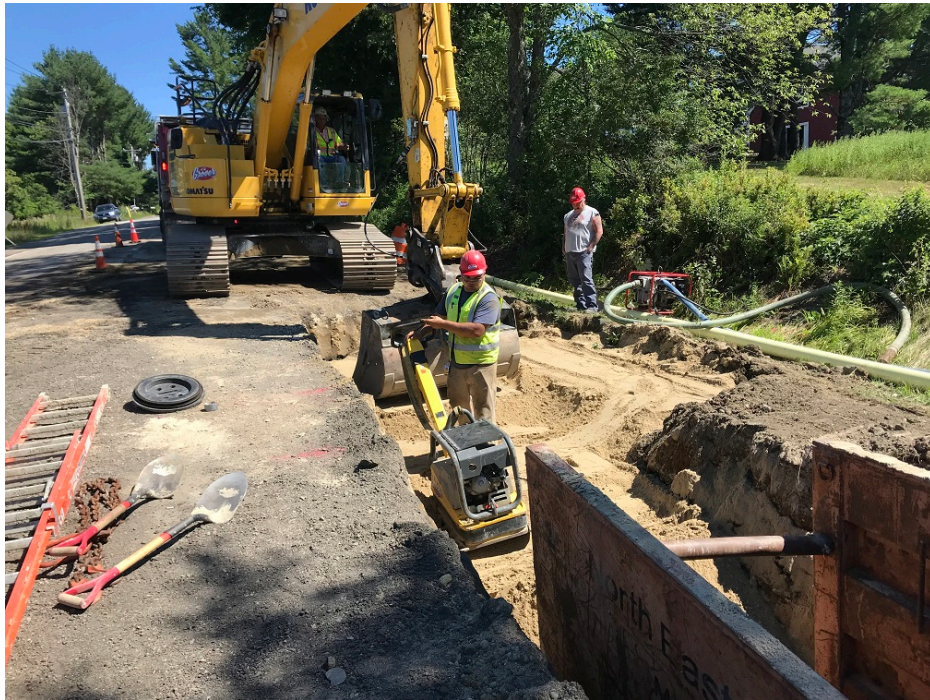
Photo 5 – Backfilling and compacting over new 16 inch water main
