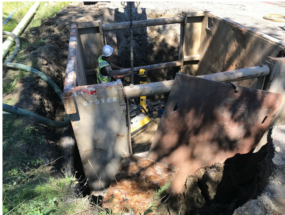
Photo 2 – Compacting the sand over new 16 inch DI
