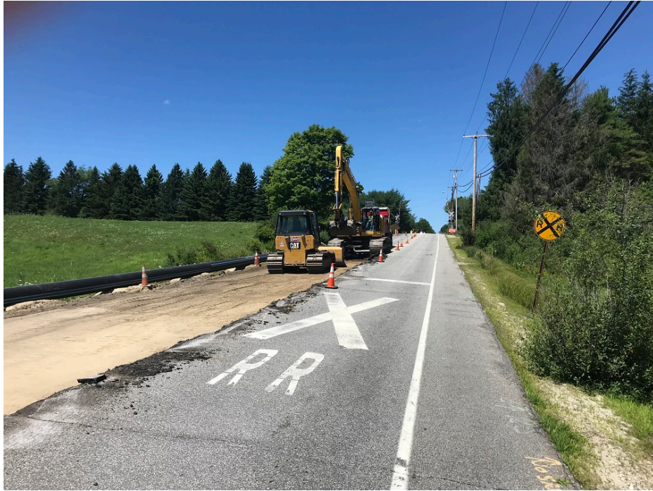
Photo 1 – Crew removing pavement near rail road tracks
