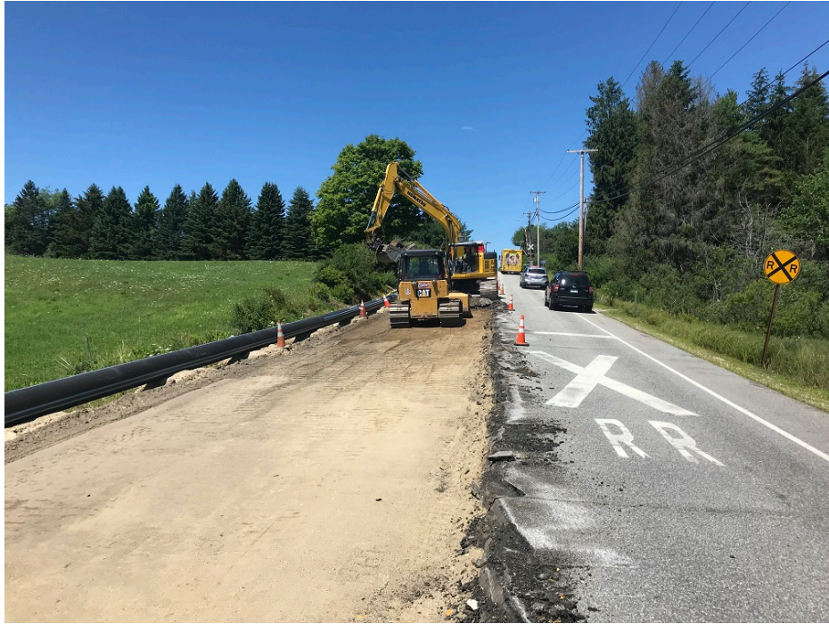
Photo 1 – Crew removing pavement near rail road tracks
