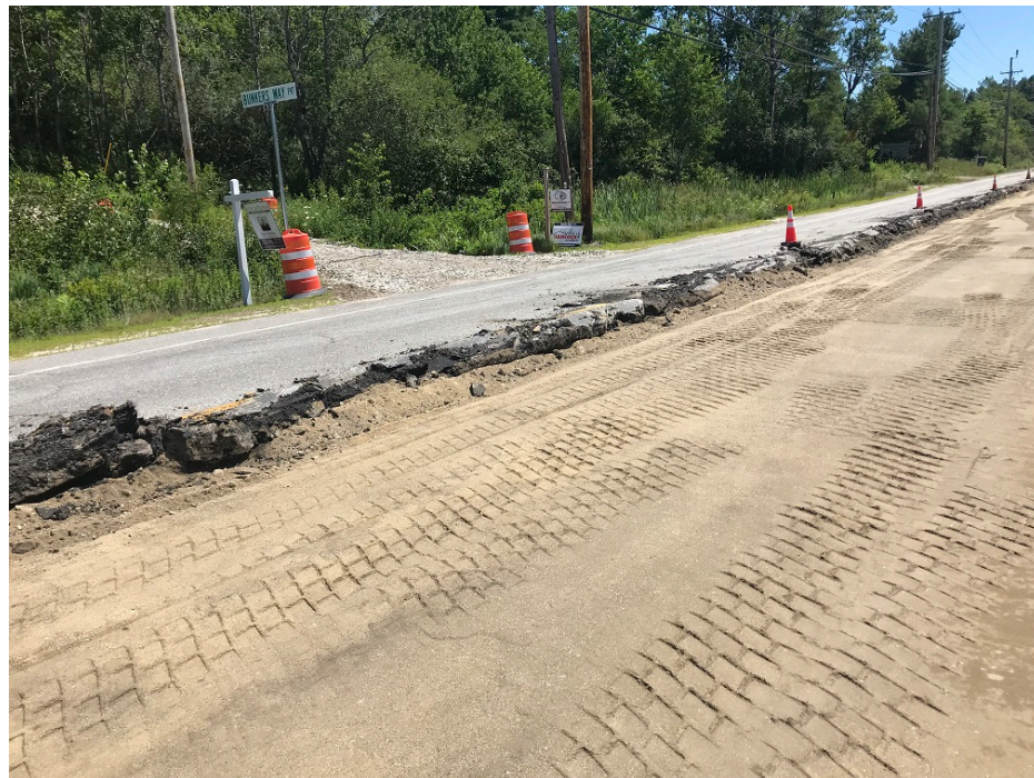
Photo 2 – 8 to 10 inches of pavement on Tuttle Road
