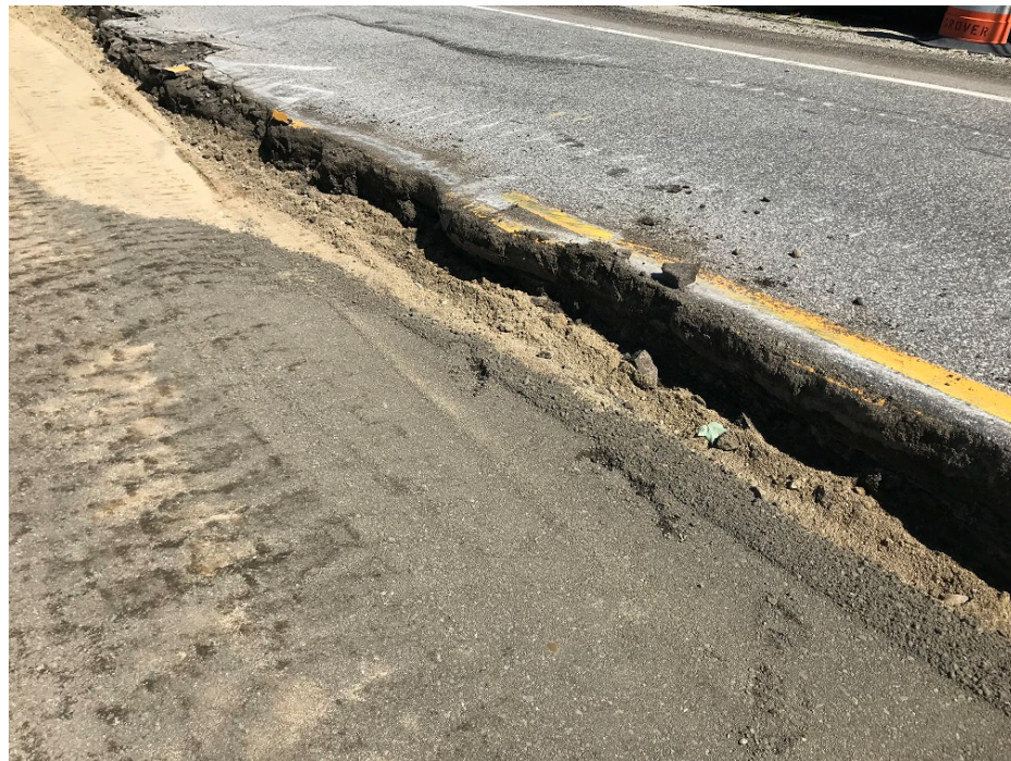
Photo 2 – 8 to 10 inches of pavement on Tuttle Road
