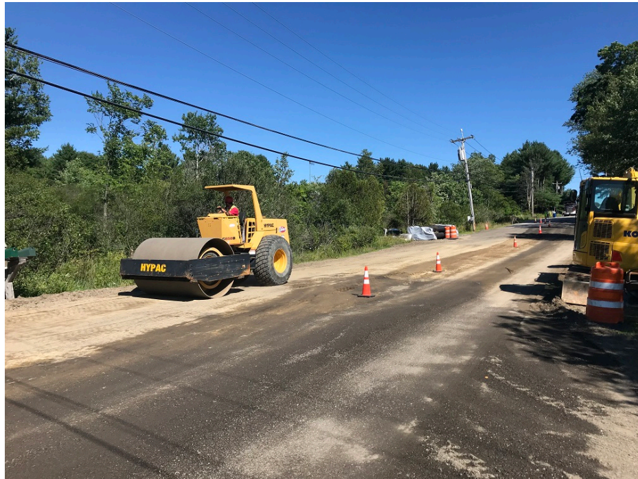
Photo 2 – Compacting gravel on north side of Tuttle Road near PWD pump house
