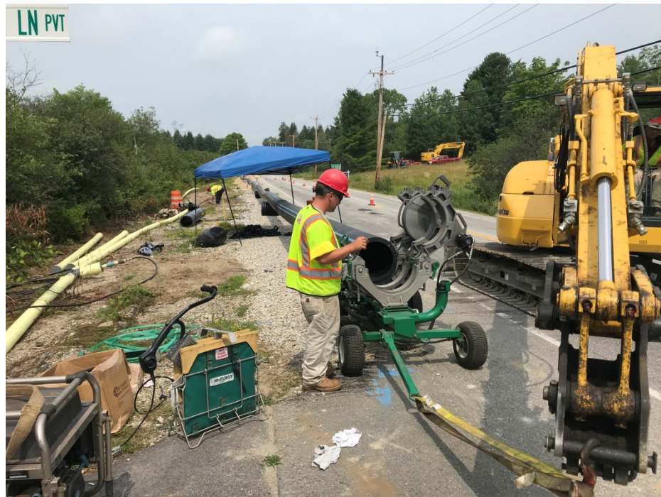
Photo 2 – Preparing to fuse 16 inch HDPE water main
