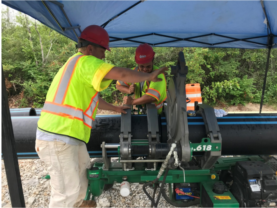
Photo 1 – Preparing to fuse 16 inch HDPE water main
