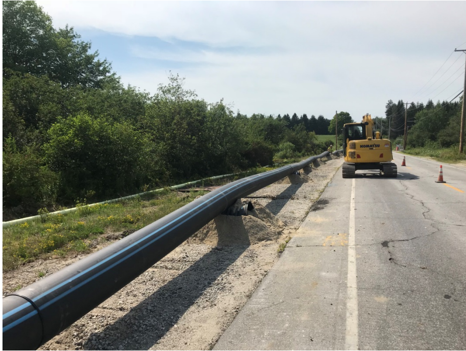
Photo 1 – Fused 16 inch diameter water main
