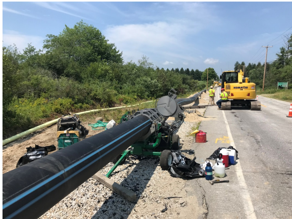
Photo 2 – Fusing 16 inch diameter water main
