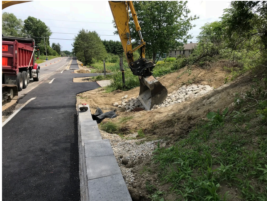
Photo 3 – Rip Rapping around field inlet near block retaining wall
