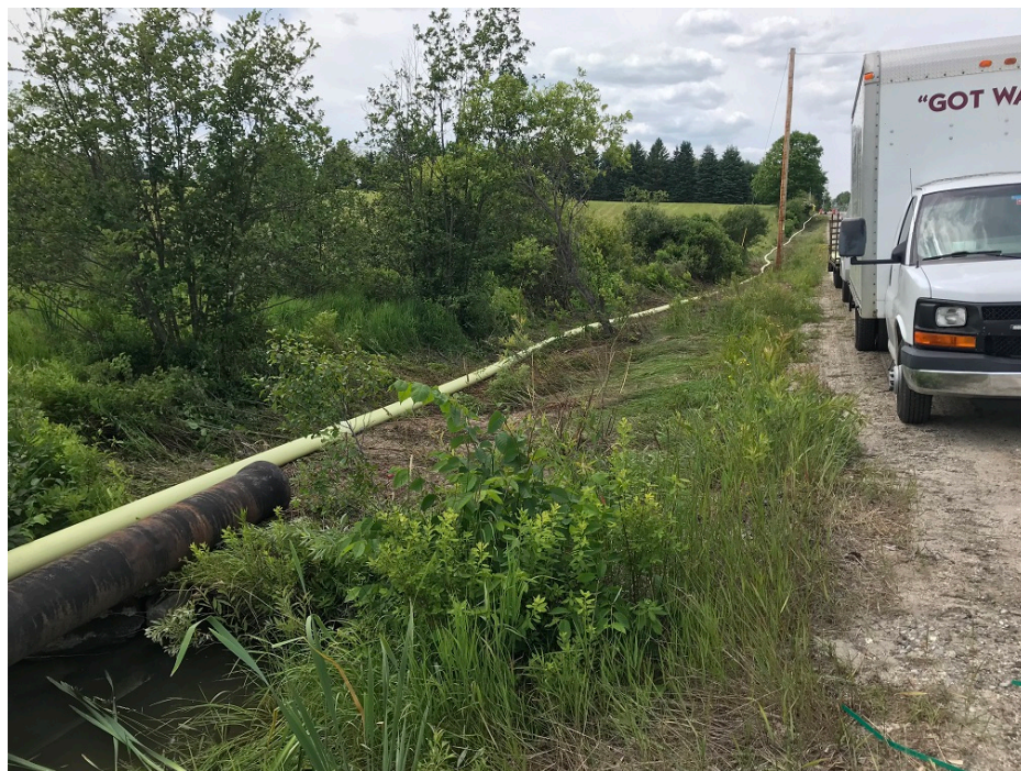
Photo 4 – Installing temporary water on east side of rail road tracks
