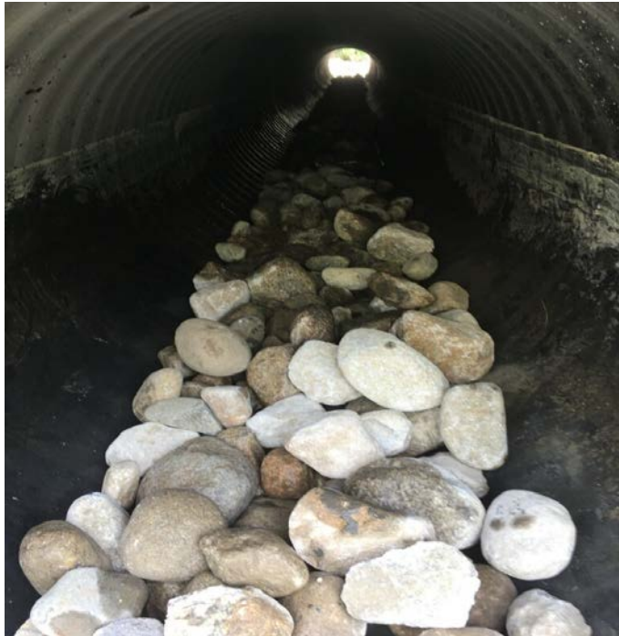
Photo 2 – Imbedded 36 inch dual culvert in front of 272 Tuttle Road
