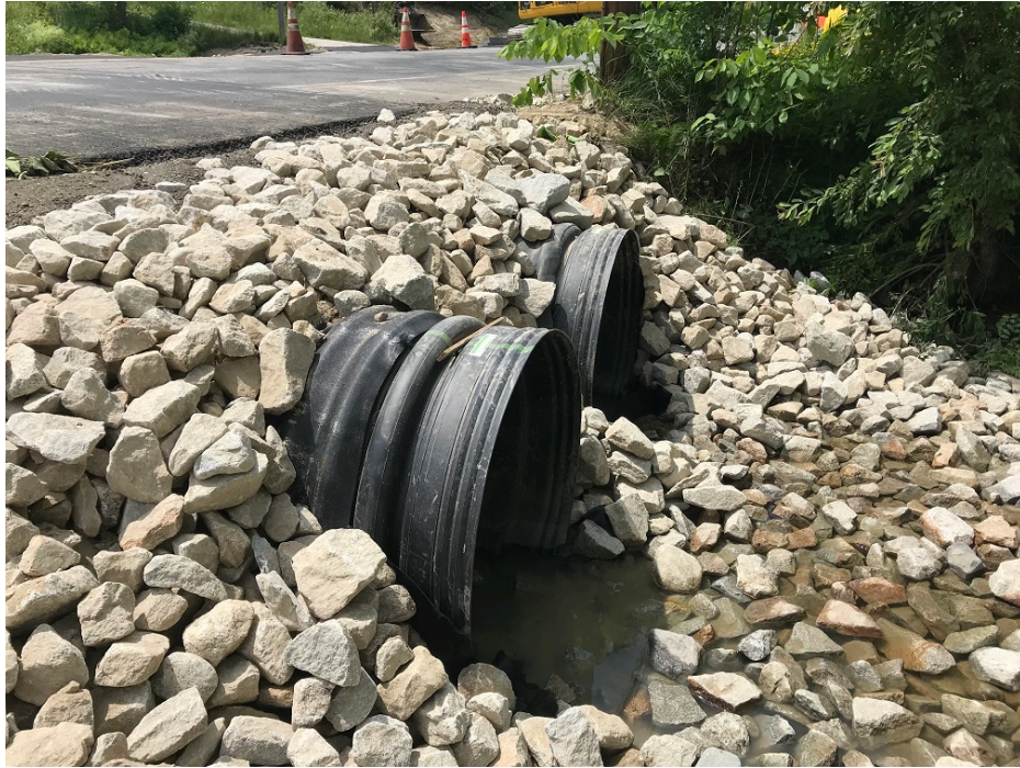
Photo 1 – Rip rap inlet for 36 inch dual culverts near 272 Tuttle Road
