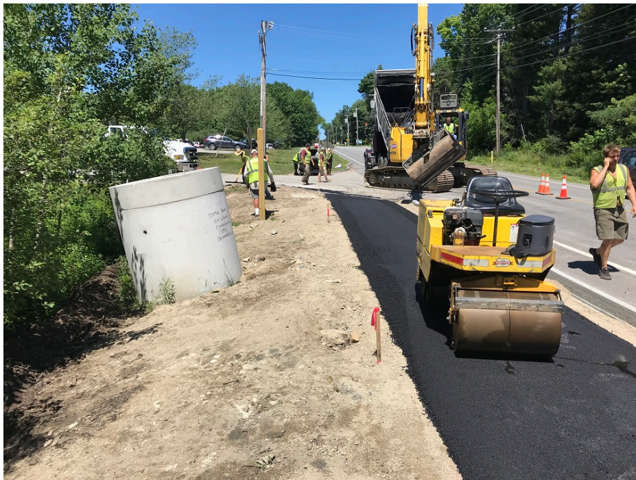
Photo 6 – Compacting paved sidewalk base course near Town Hall
