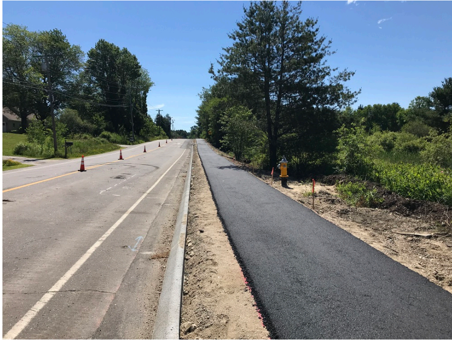
Photo 1 – Paved sidewalk base course in front of 272 Tuttle Road
