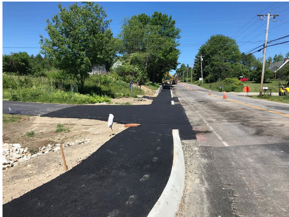
Photo 2 – Paved base course of driveway at 272 Tuttle Road
