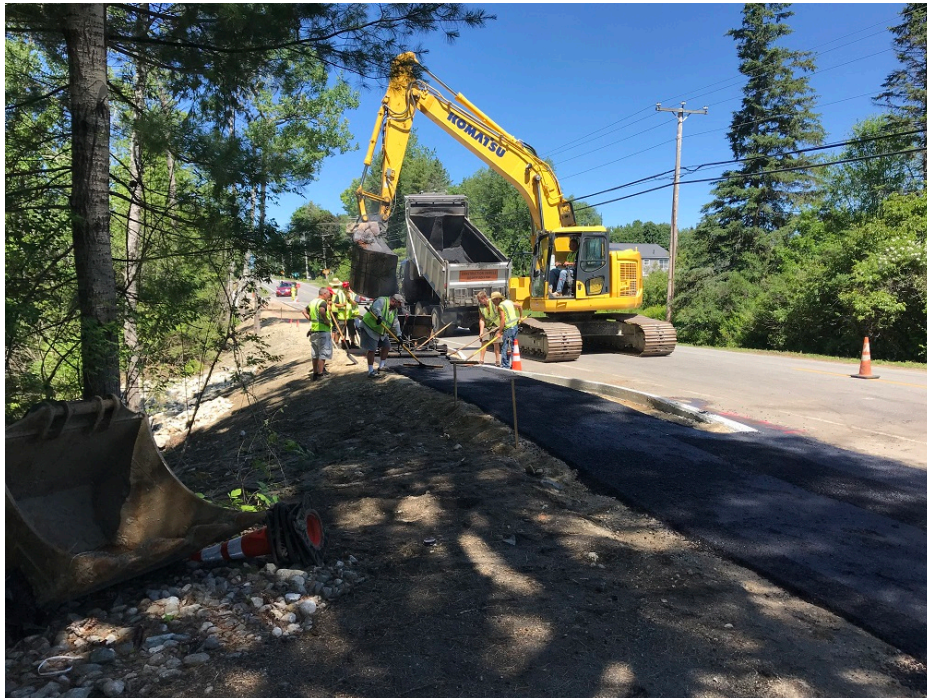
Photo 4 – Paving sidewalk base course in front of 290 Tuttle Road
