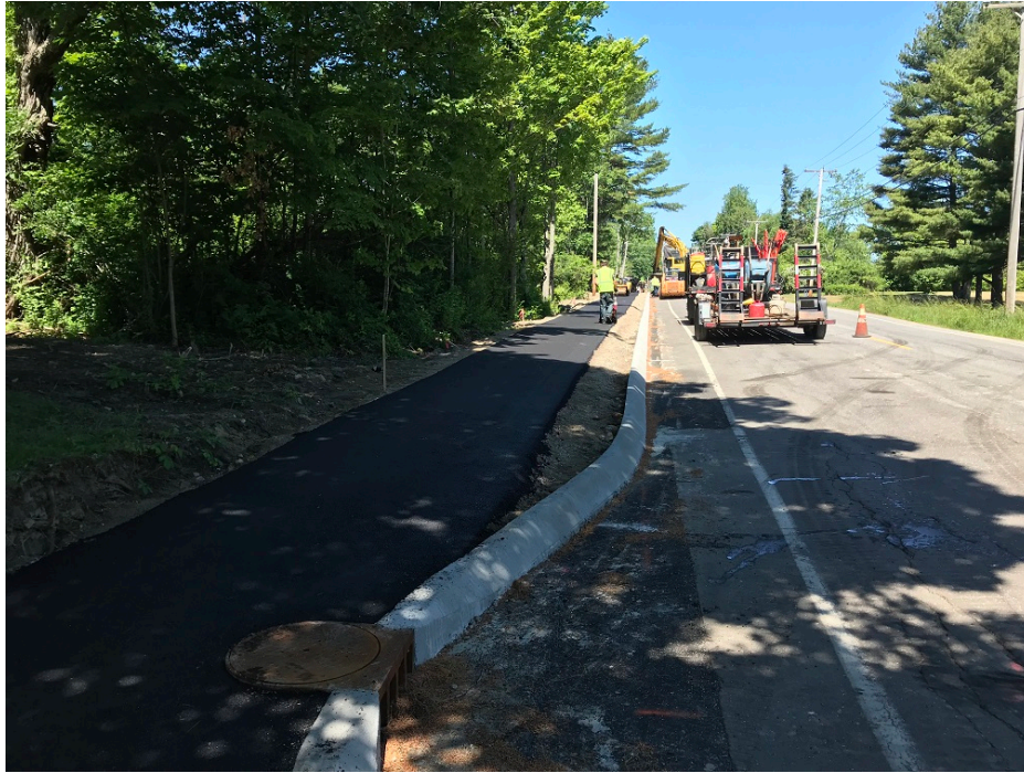
Photo 3 – Paved sidewalk base course near 290 Tuttle Road
