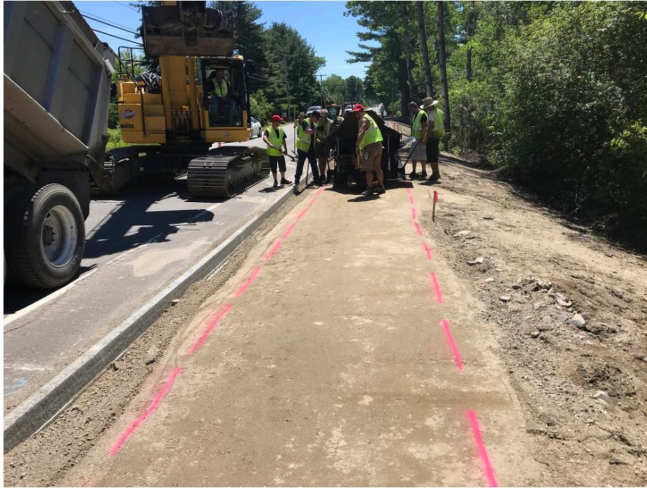
Photo 5 – Paving sidewalk base course near Town Hall
