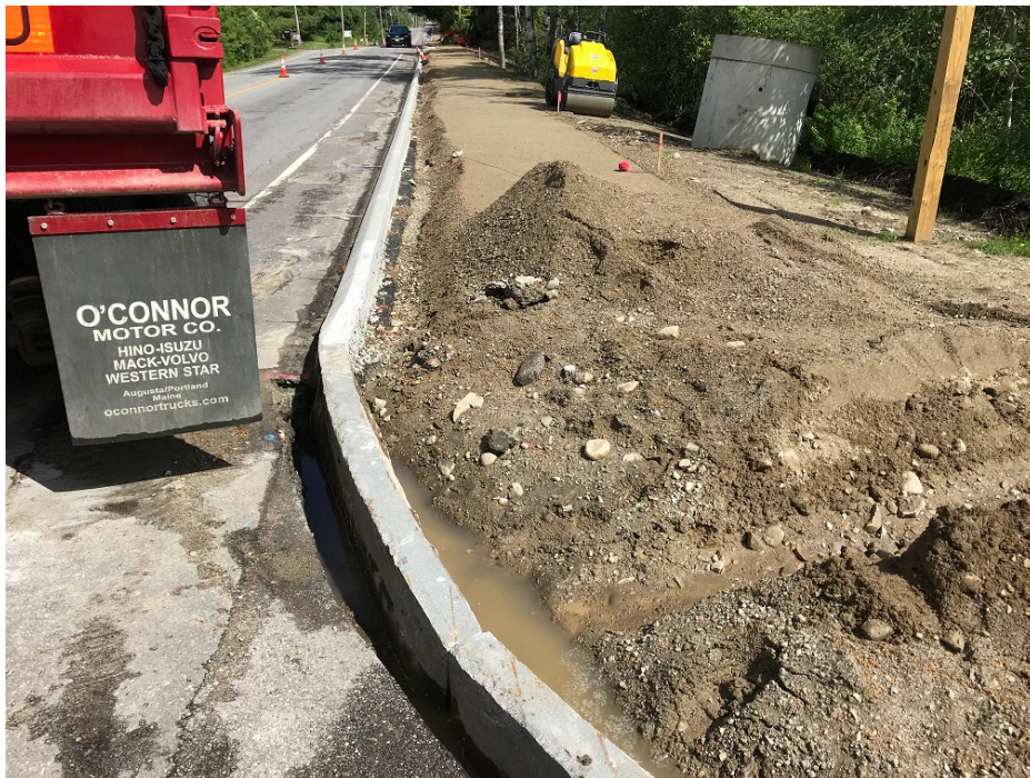
Photo 6 – Granite curb reset to match new concrete slipform curb
