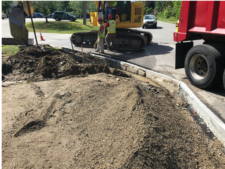
Photo 4 – Resetting granite curb at Town Hall Entrance to match new sidewalk
