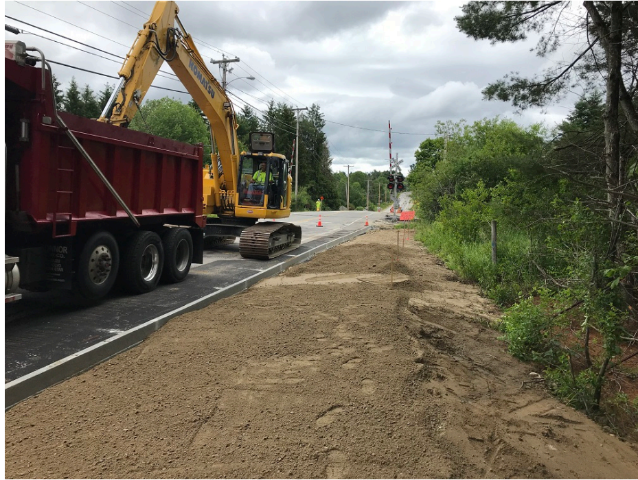
Photo 3 – Placing gravel for new sidewalk near rail road tracks
