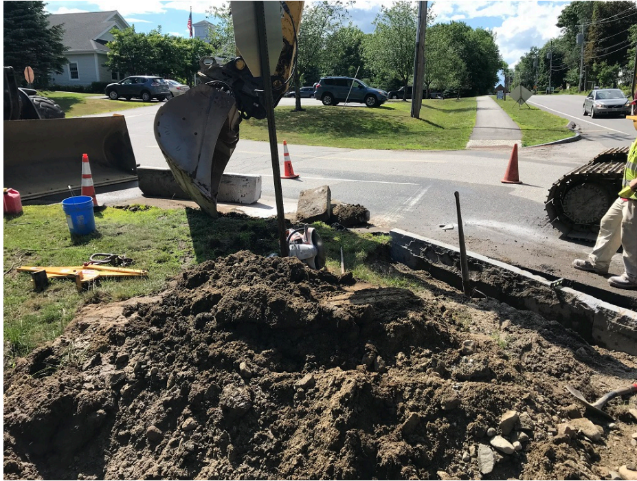
Photo 5 – Removing and resetting granite curb at Town Hall entrance
