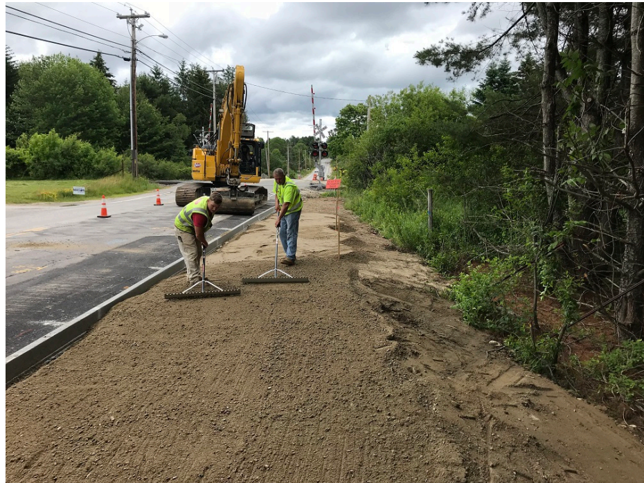
Photo 2 – Grading gravel for new sidewalk near rail road tracks
