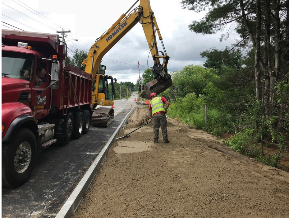
Photo 1 – Placing and grading gravel for new sidewalk near rail road tracks
