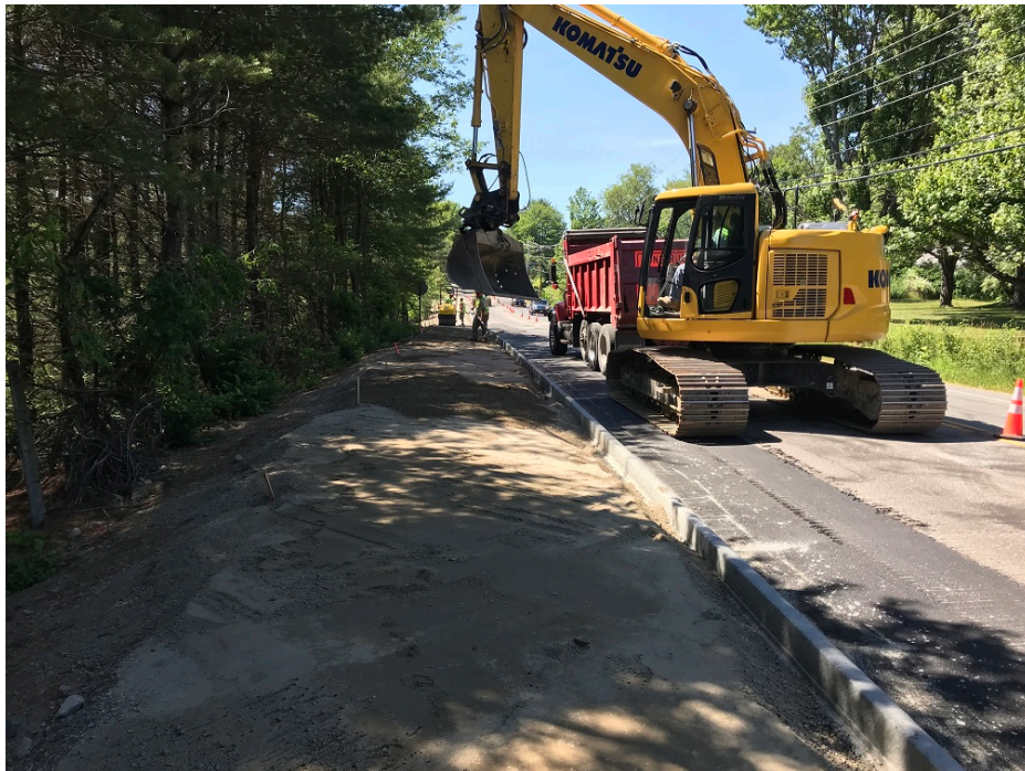
Photo 4 – Placing gravel and grading sidewalk extension near rail road tracks
