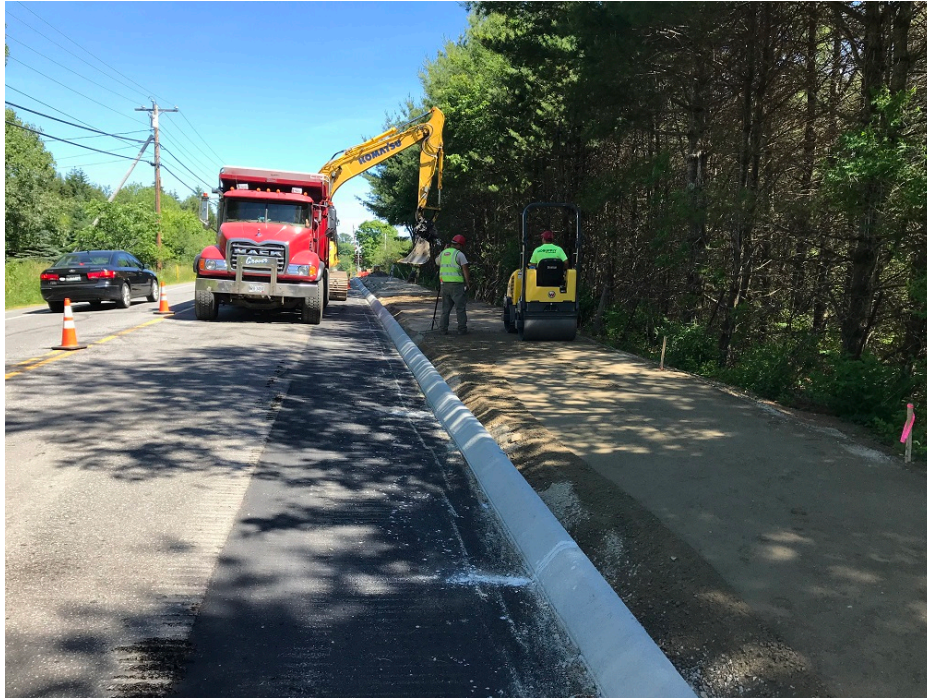
Photo 5 – Compacting graded gravel for sidewalk extension near rail road tracks
