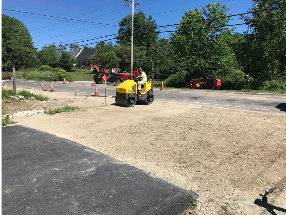
Photo 3 – Compacting driveway entrance at 272 Tuttle Road
