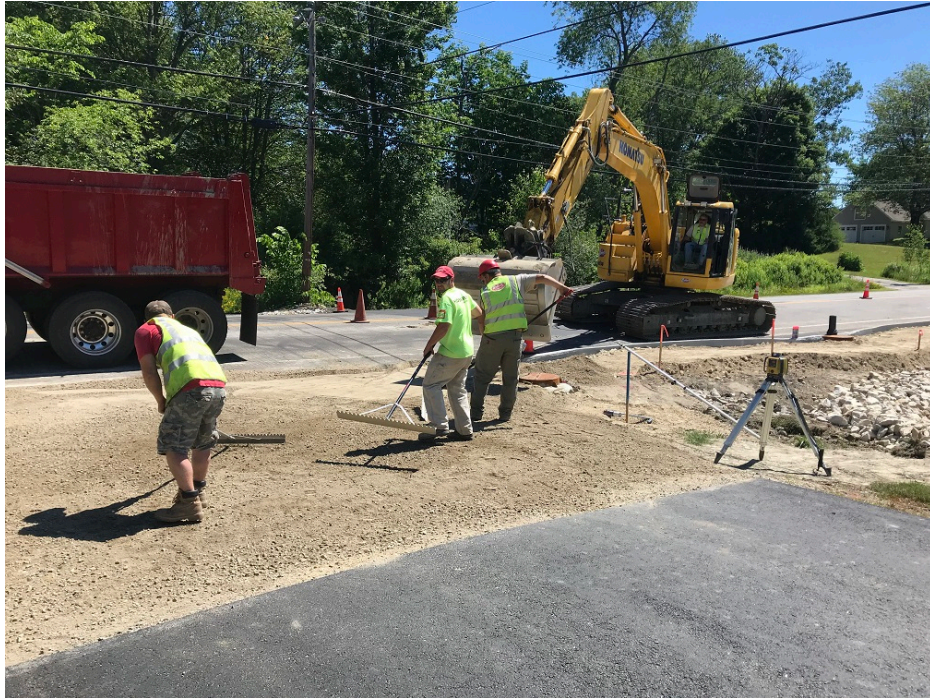
Photo 1 – Placing gravel and grading at 272 Tuttle Road
