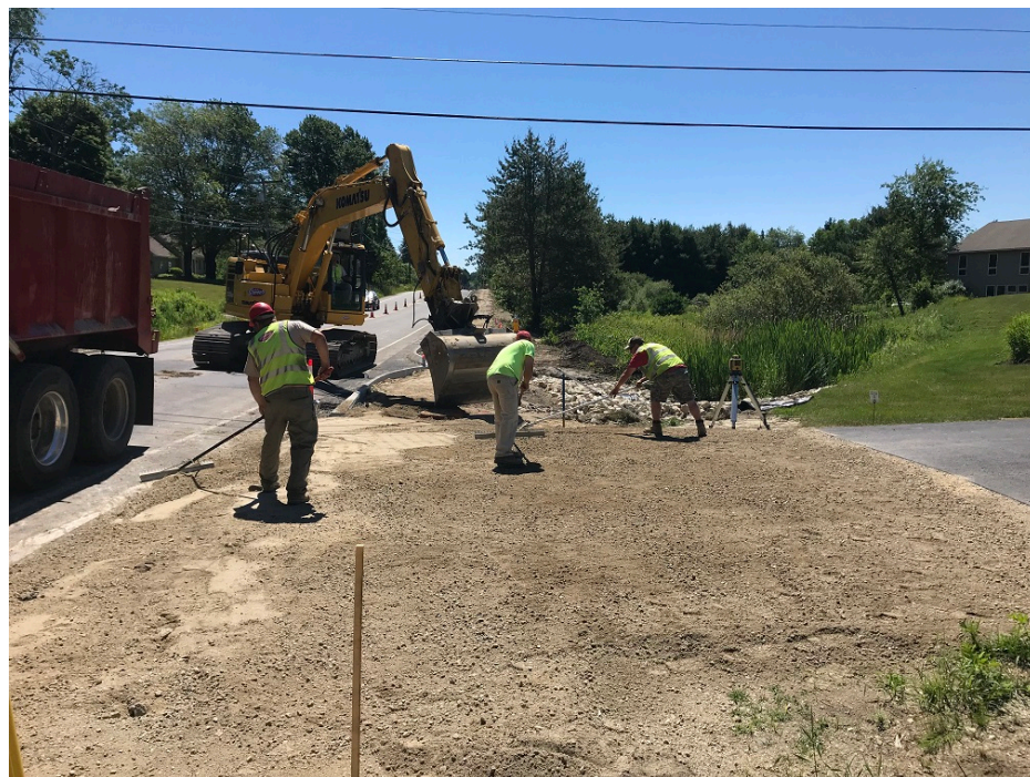
Photo 2 – Placing gravel and grading the driveway entrance at 272 Tuttle Road
