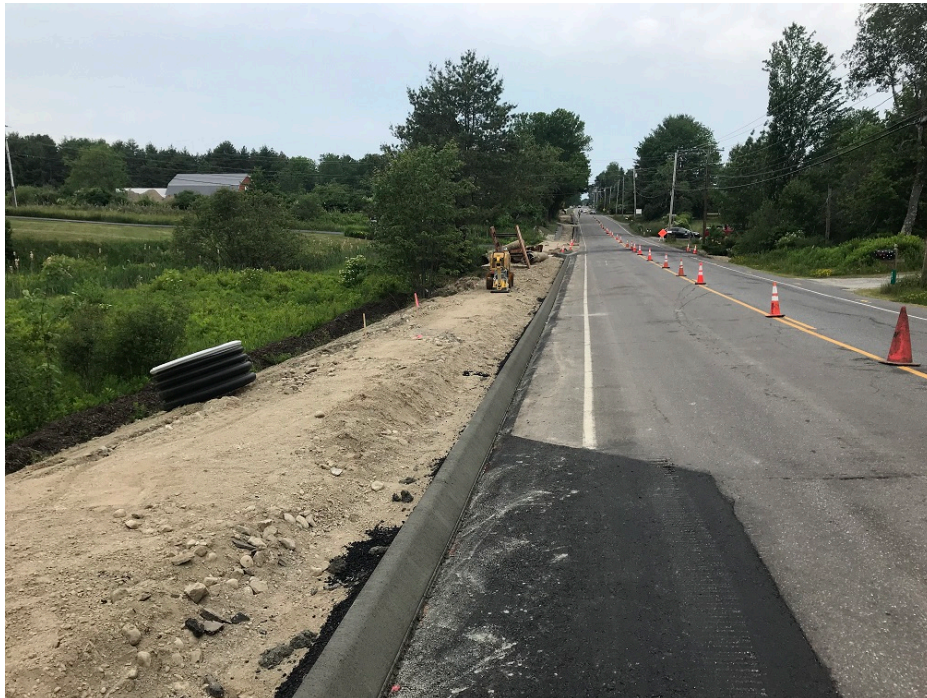
Photo 6 – Concrete slipform curb in front of 272 Tuttle Road
