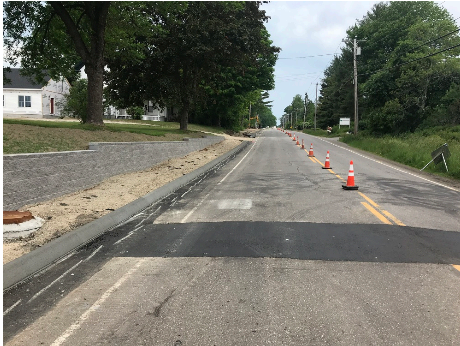
Photo 4 – Concrete slipform curb in front of 280 Tuttle Road
