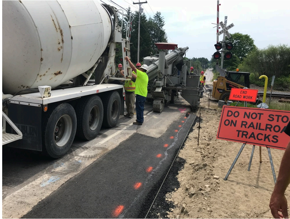
Photo 3 – Beginning curb placement near rail road tracks
