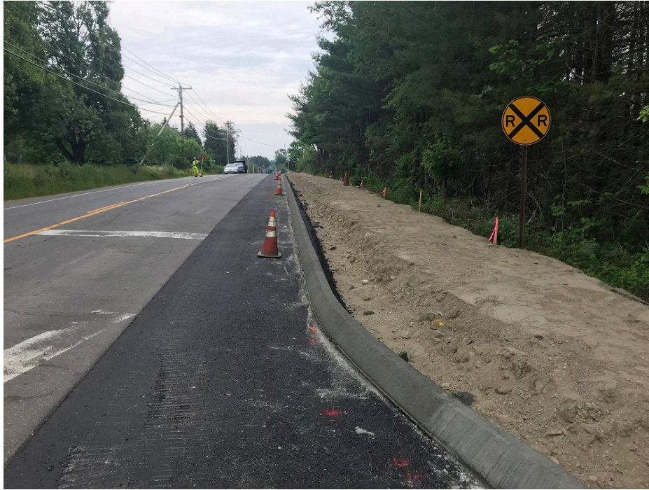
Photo 5 – Concrete slipform curb near rail road tracks
