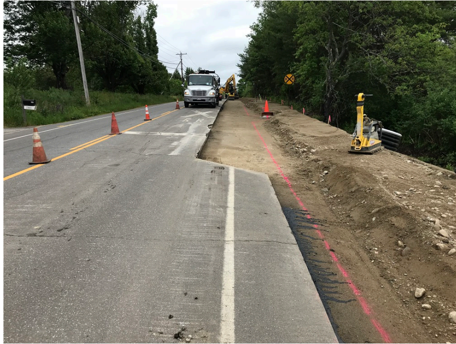
Photo 3 – Placing tack coat on pavement joint
