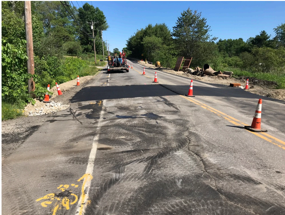
Photo 6 – Cross trench paving over dual 36 inch culverts
