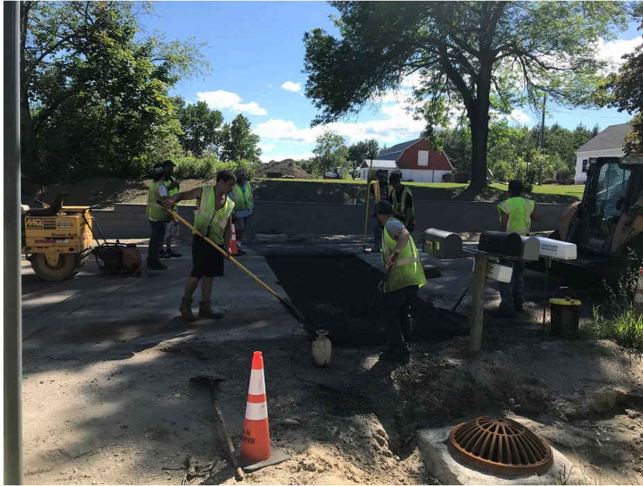
Photo 5 – Paving cross trench in front of rock retaining wall at 280 Tuttle Road
