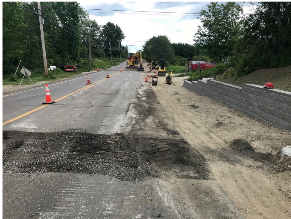
Photo 2 – Prepped curb pad in front of 280 Tuttle Road
