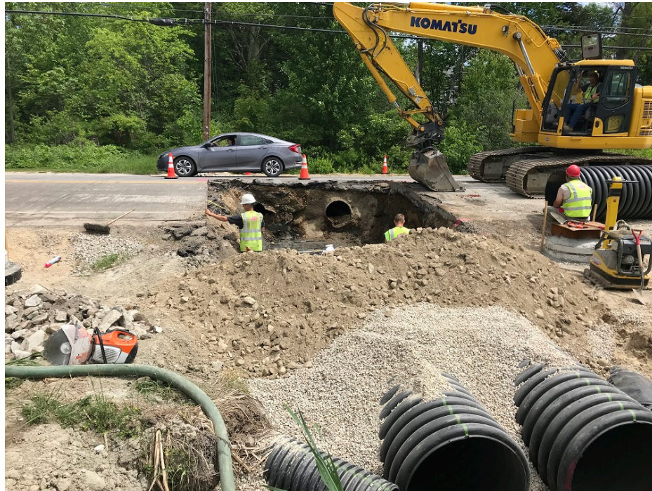
Photo 3 – Installing 36 inch HDPE dual culverts
