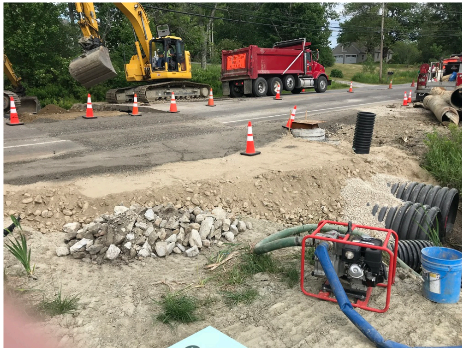
Photo 4 – 36 inch HDPE dual culverts installed
