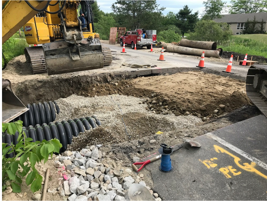
Photo 3 – Backfilling 36 inch HDPE dual culverts
