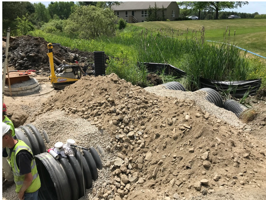
Photo 2 – First two sections of 36 inch HDPE dual culverts
