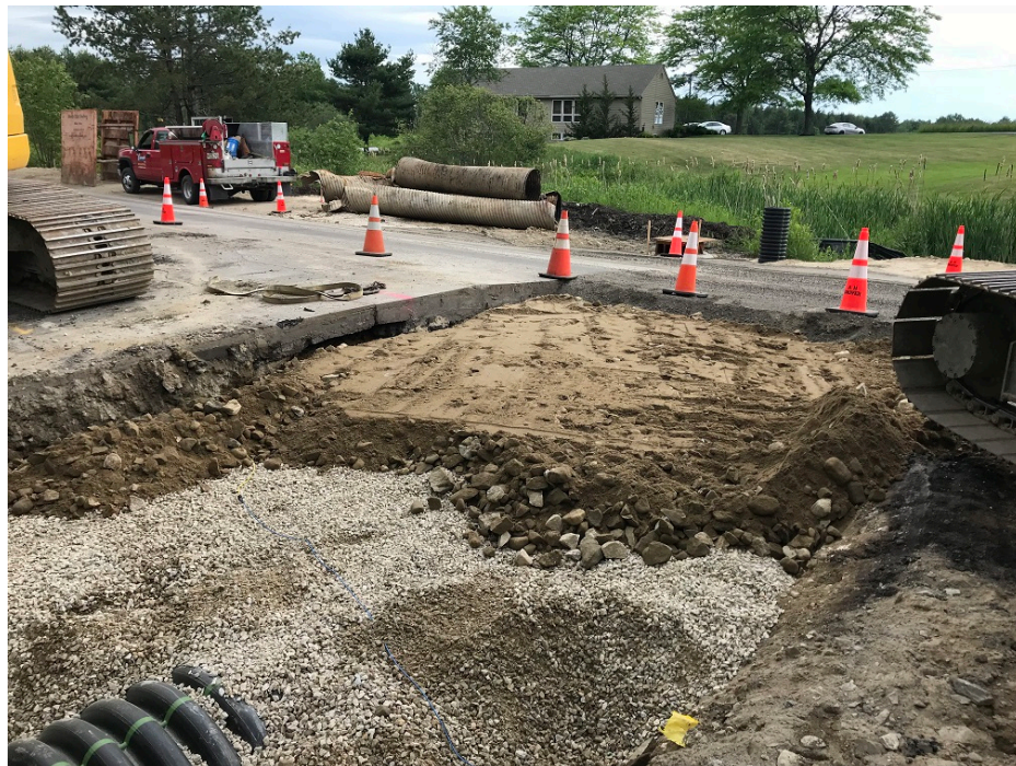
Photo 4 – Backfilling 36 inch HDPE dual culverts
