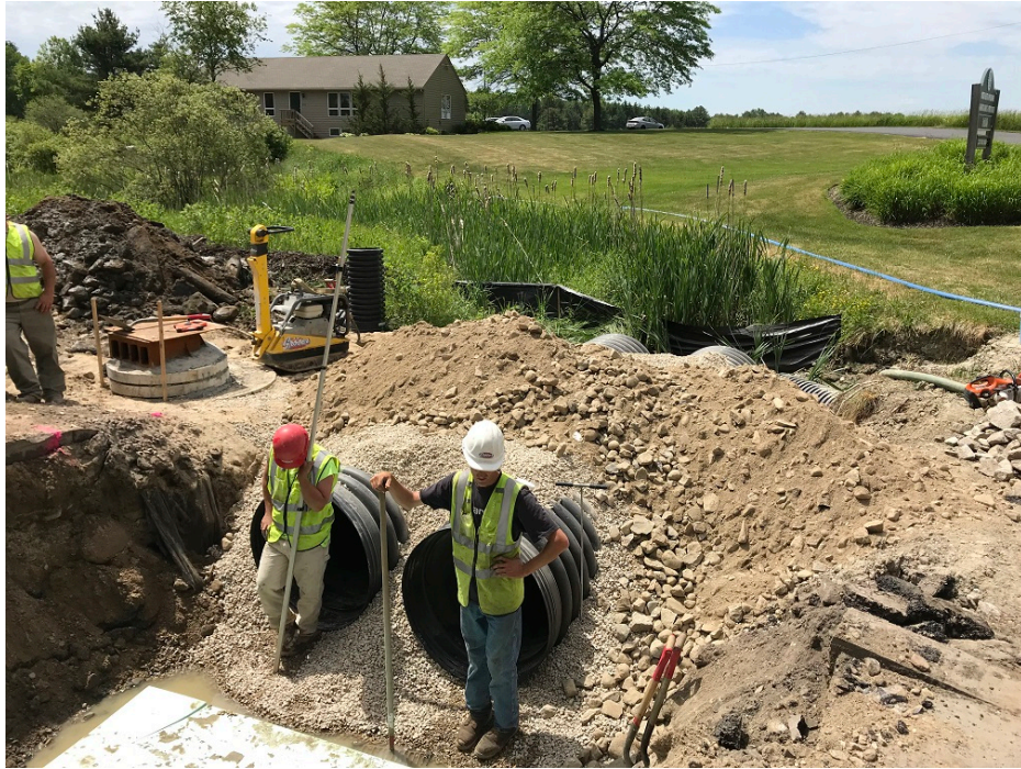
Photo 1 – Installing the first two sections of 36 inch HDPE dual culverts
