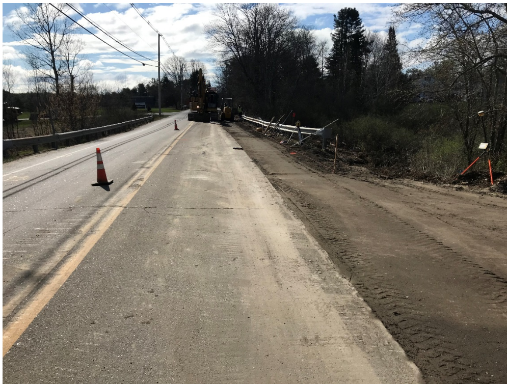
Photo 2 – Graded curb pad approximate STA 17+00
