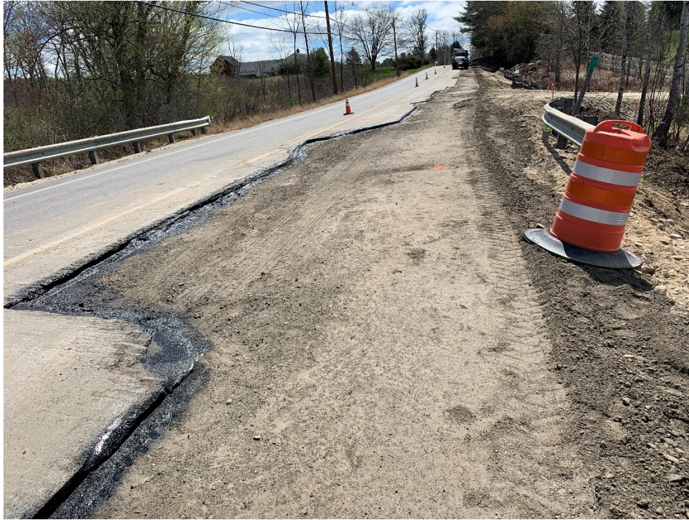
Photo 1 – Graded curb pad with tack coat approximate STA 10+00
