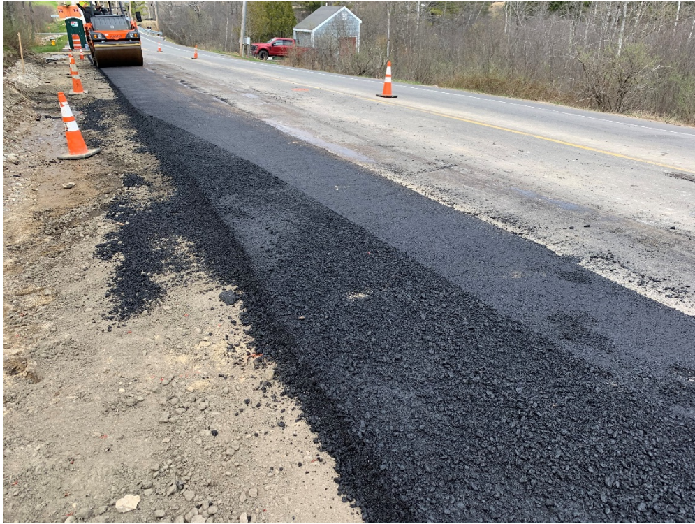
Photo 3 – Placing and compacting pavement approximate STA 2+00
