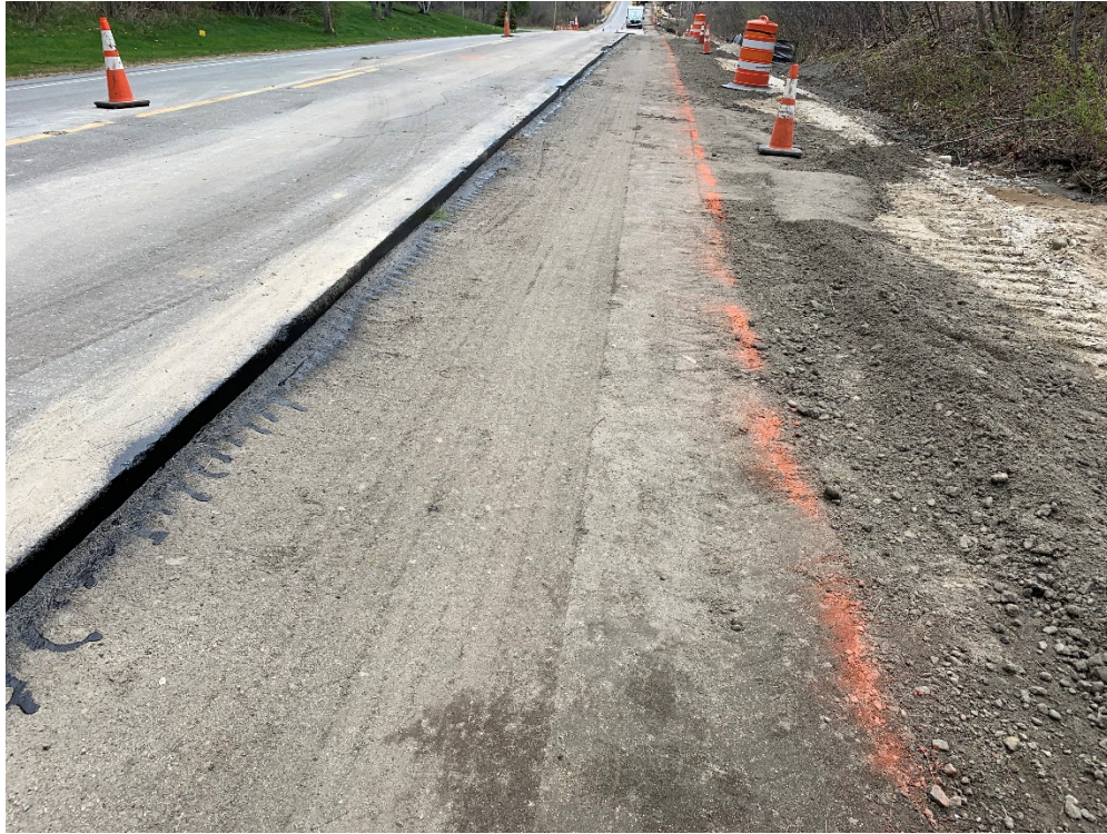
Photo 5 – Paved curb pad with tack coat approximate STA 5+50
