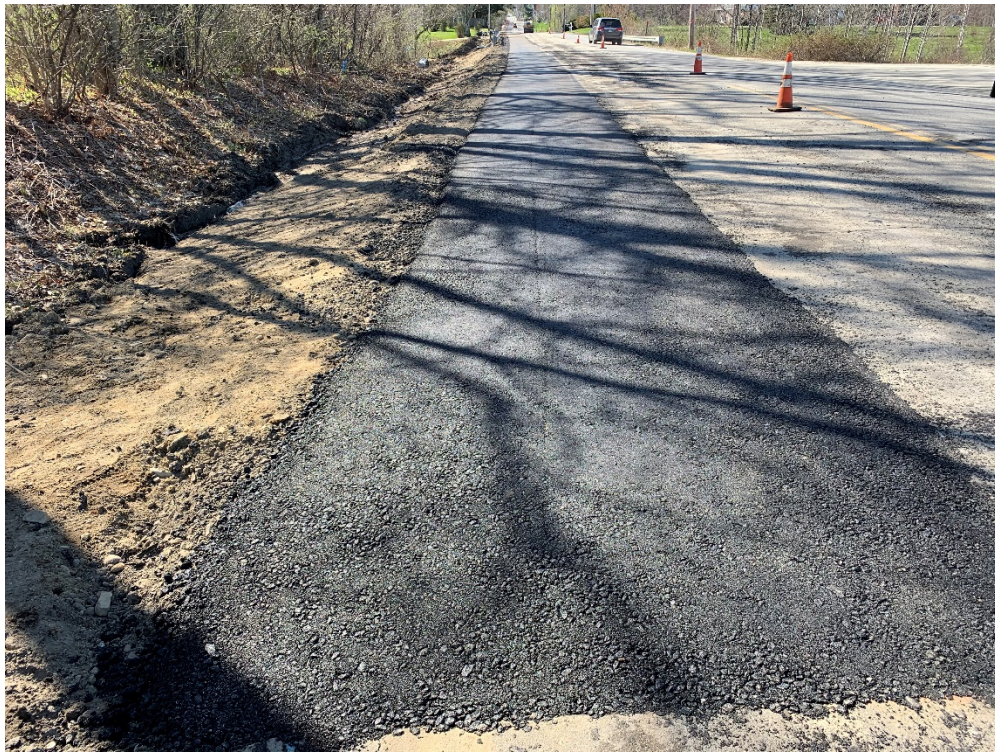
Photo 6 – Paved curb pad in front of 196 Tuttle Road
