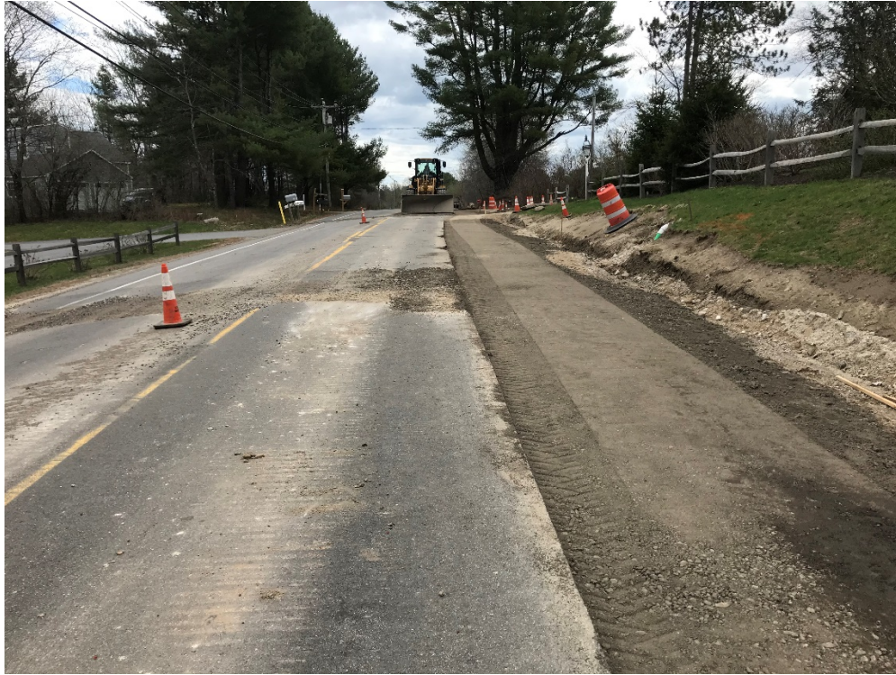
Photo 1 – Curb pad, graded for pavement approximate STA 1+75
