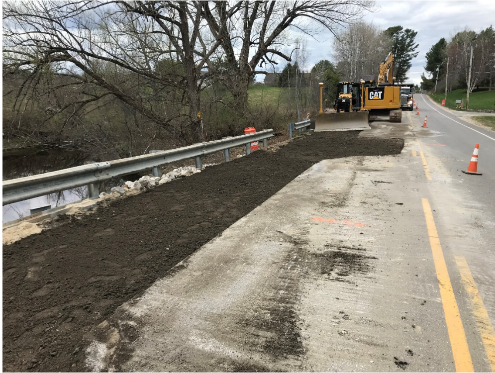
Photo 3 – Graded curb pad approximate STA 9+50
