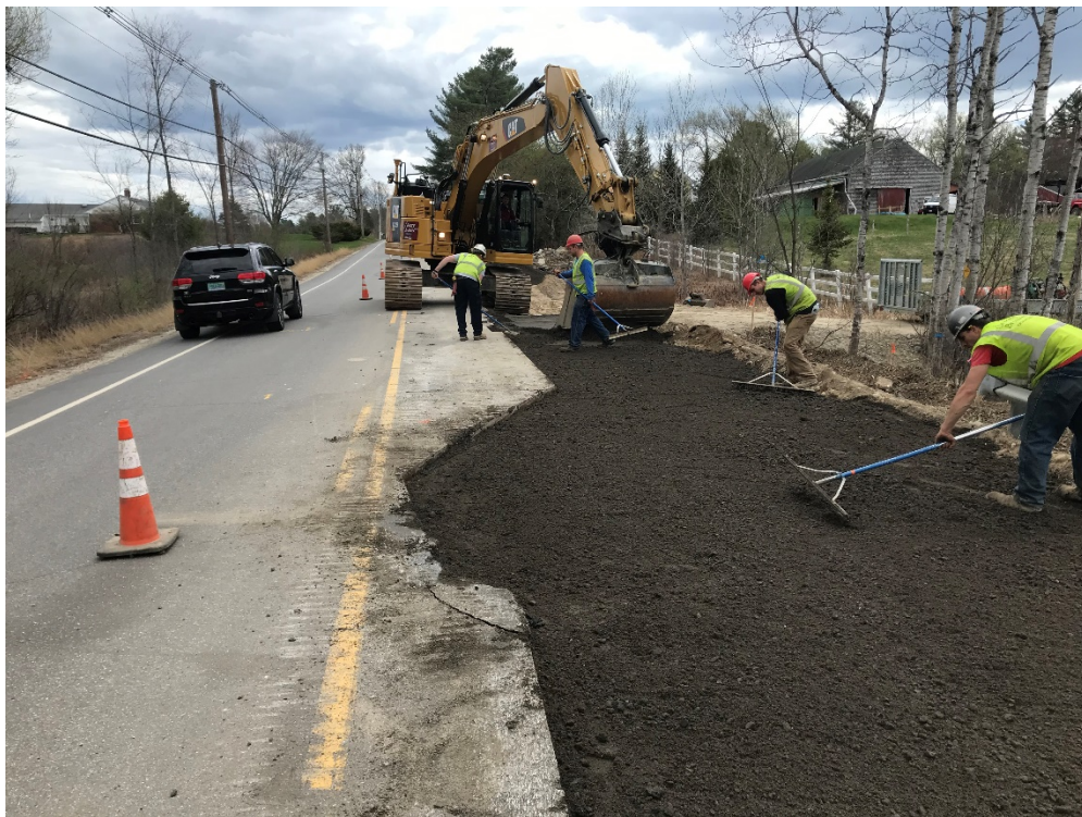
Photo 4 – Placing and grading reclaim for curb pad
