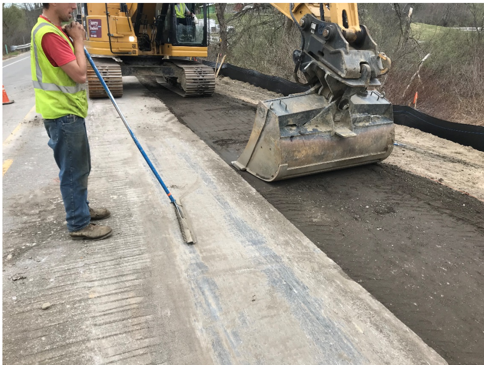
Photo 2 – Placing and grading reclaim for curb pad approximate STA 10+50
