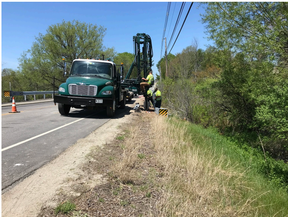
Photo 4 – Installing guardrail over 12 – foot culvert on northwest side of Tuttle Road
