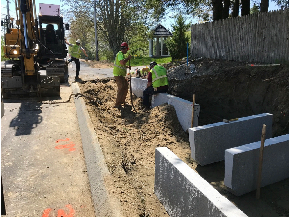
Photo 1 – Installing granite wall in front of 198 Tuttle Road
