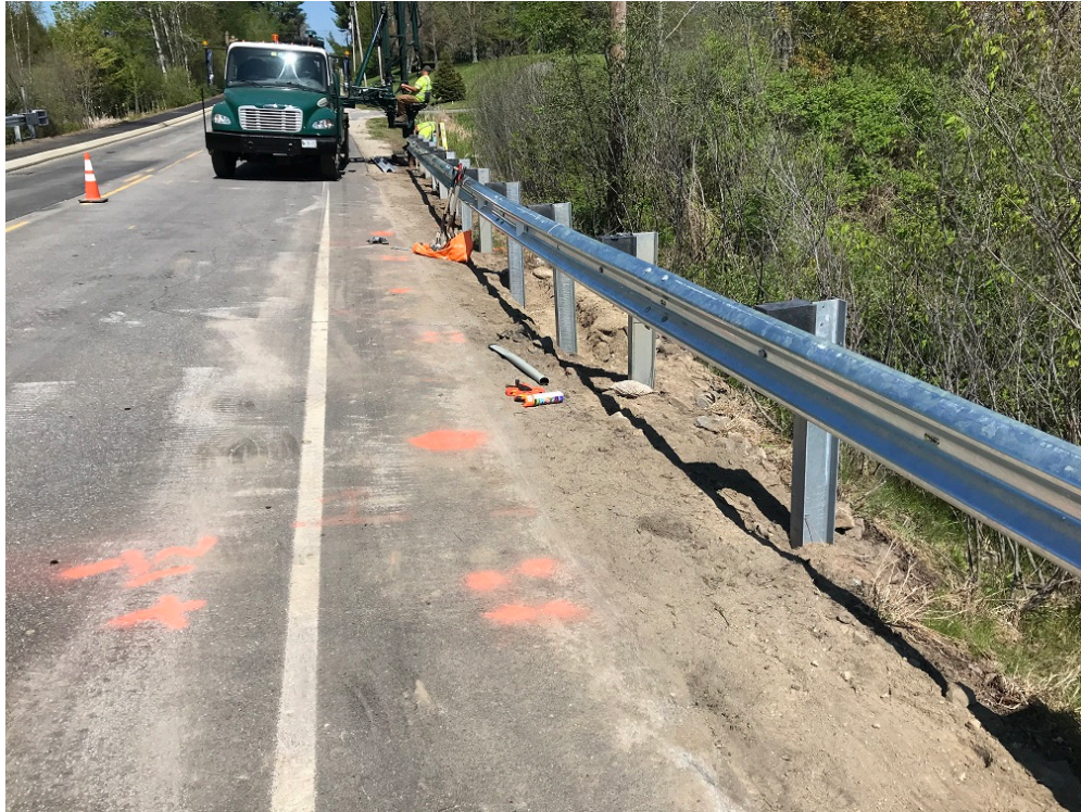
Photo 3 – Installing guardrail over 12 – culvert on northwest side of Tuttle Road
