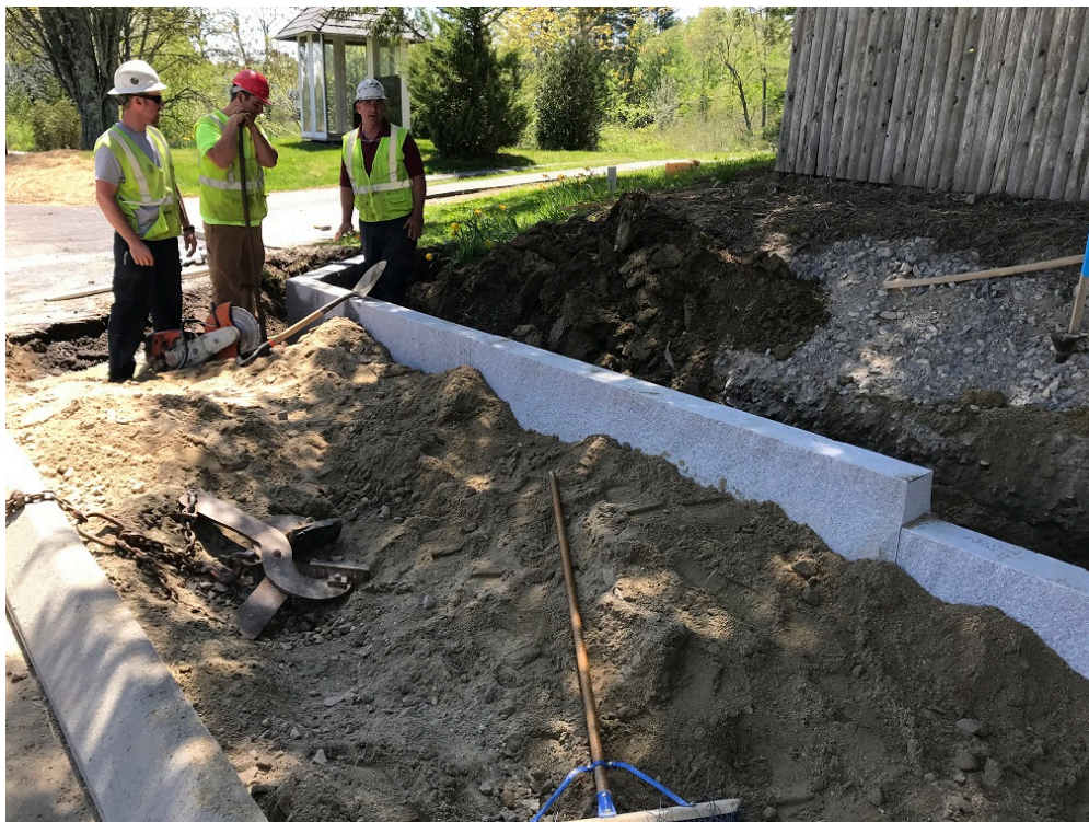
Photo 2 – Installing granite wall in front of 198 Tuttle Road
