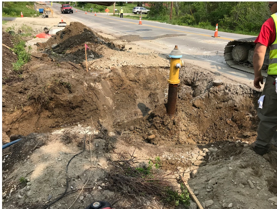
Photo 4 – Excavating around old fire hydrant at STA 8+72 to relocate
