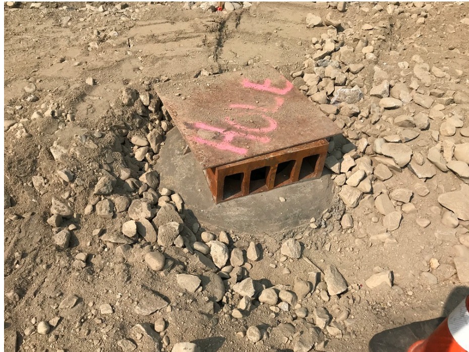
Photo 2 – Frame and grate at CB 2 complete
