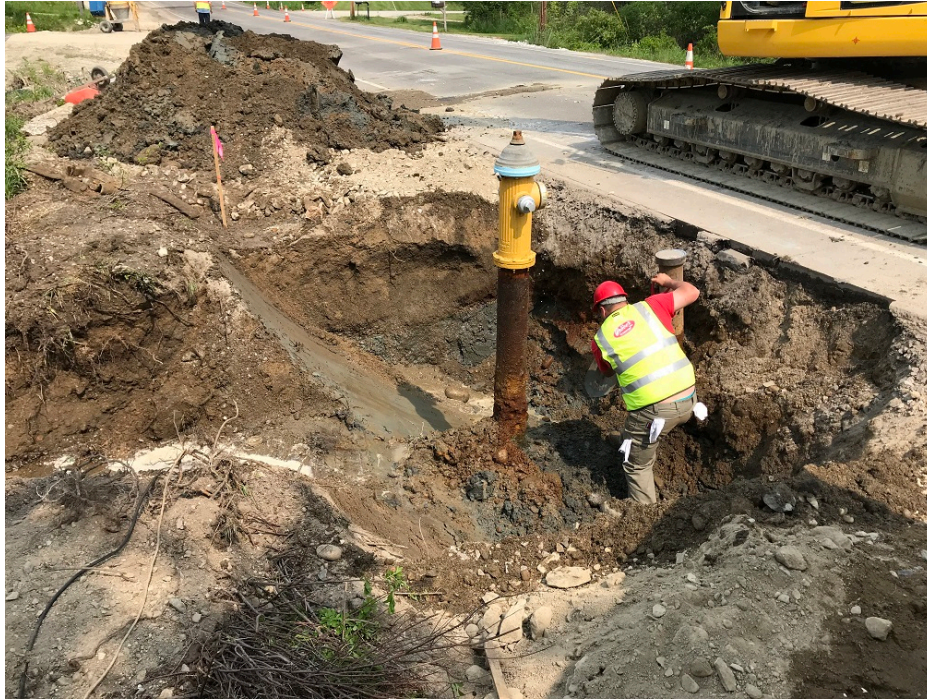
Photo 3 – Excavating around old fire hydrant at STA 8+72 to relocate
