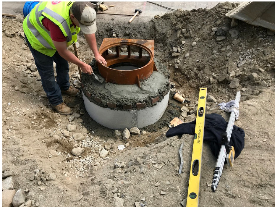
Photo 2 – Setting frame and grate at CB 2
