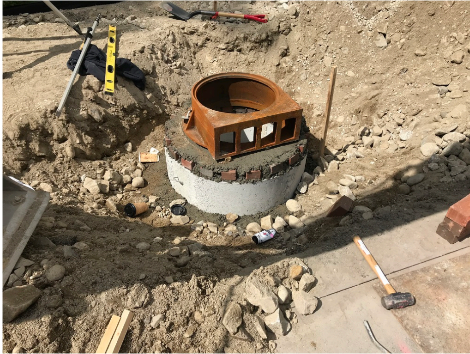
Photo 1 – Setting frame and grate at CB 2
