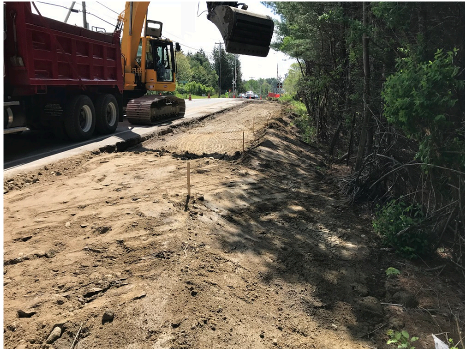
Photo 4 – Constructing sidewalk back slope near rail road tracks
