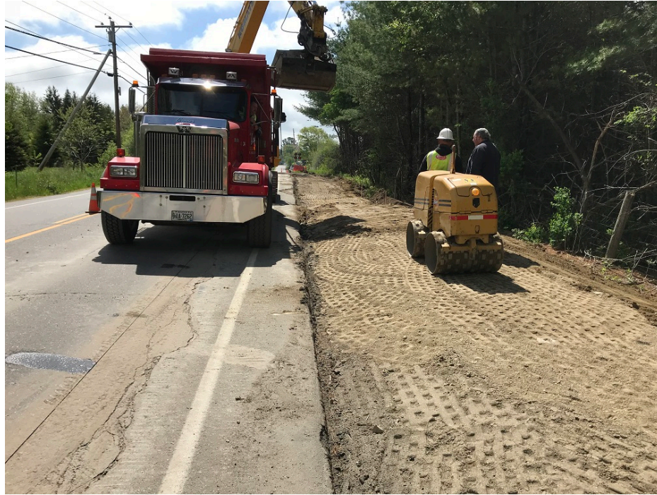
Photo 3 – Constructing sidewalk near rail road tracks
