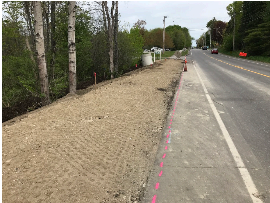
Photo 4 – Subgrade for sidewalk extension near Town Hall
