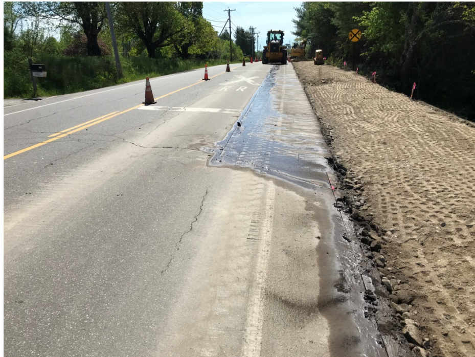
Photo 2 – Saw cutting pavement for curb installation
