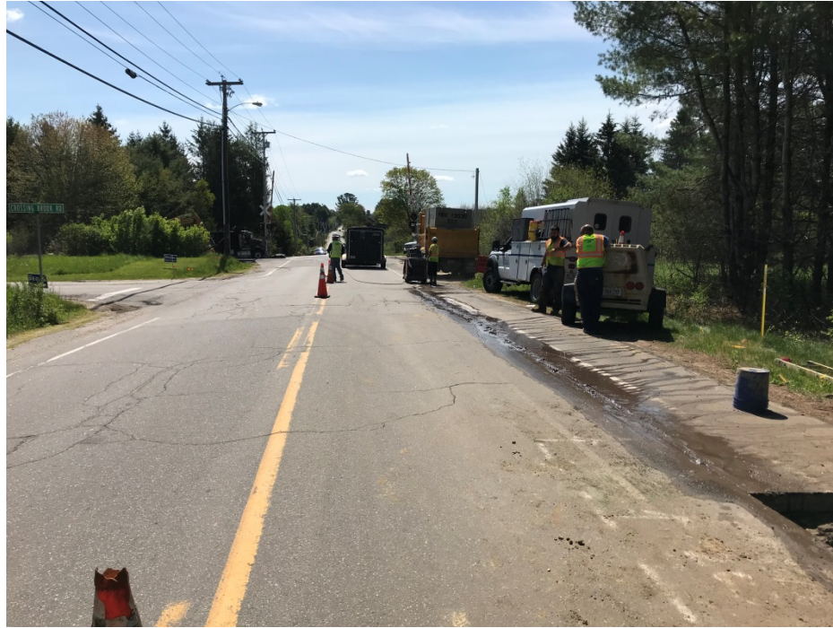
Photo 3 – Saw cutting pavement for curb installation
