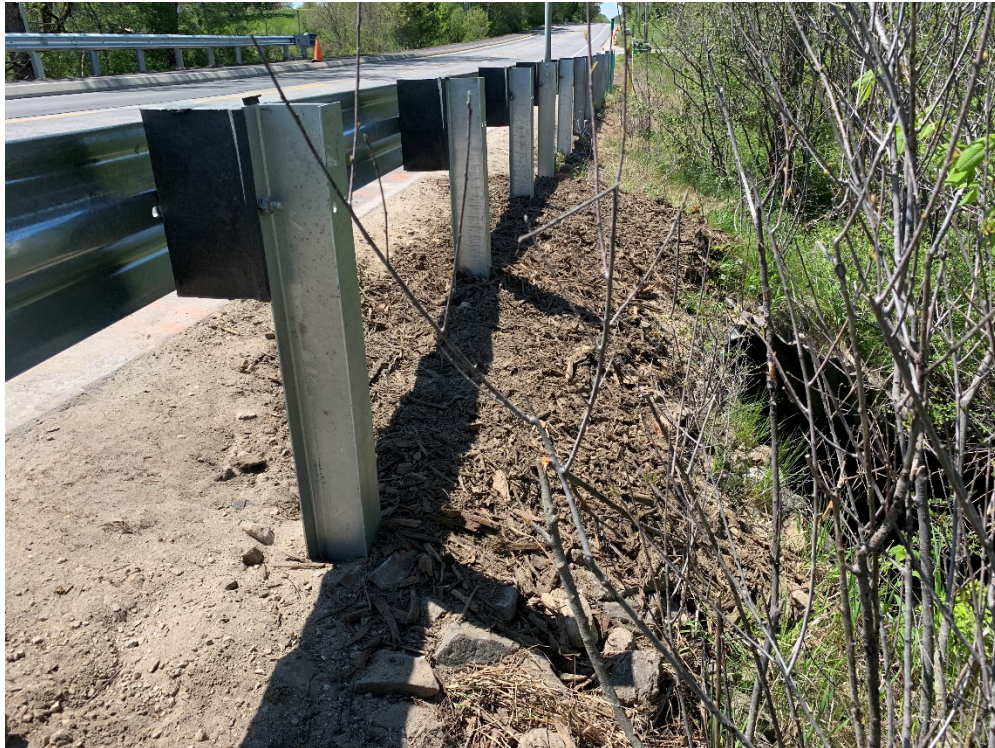
Photo 6 – Back of new guardrail installed above the 12-foot CMP culvert in Tuttle Road, looking northwest.
