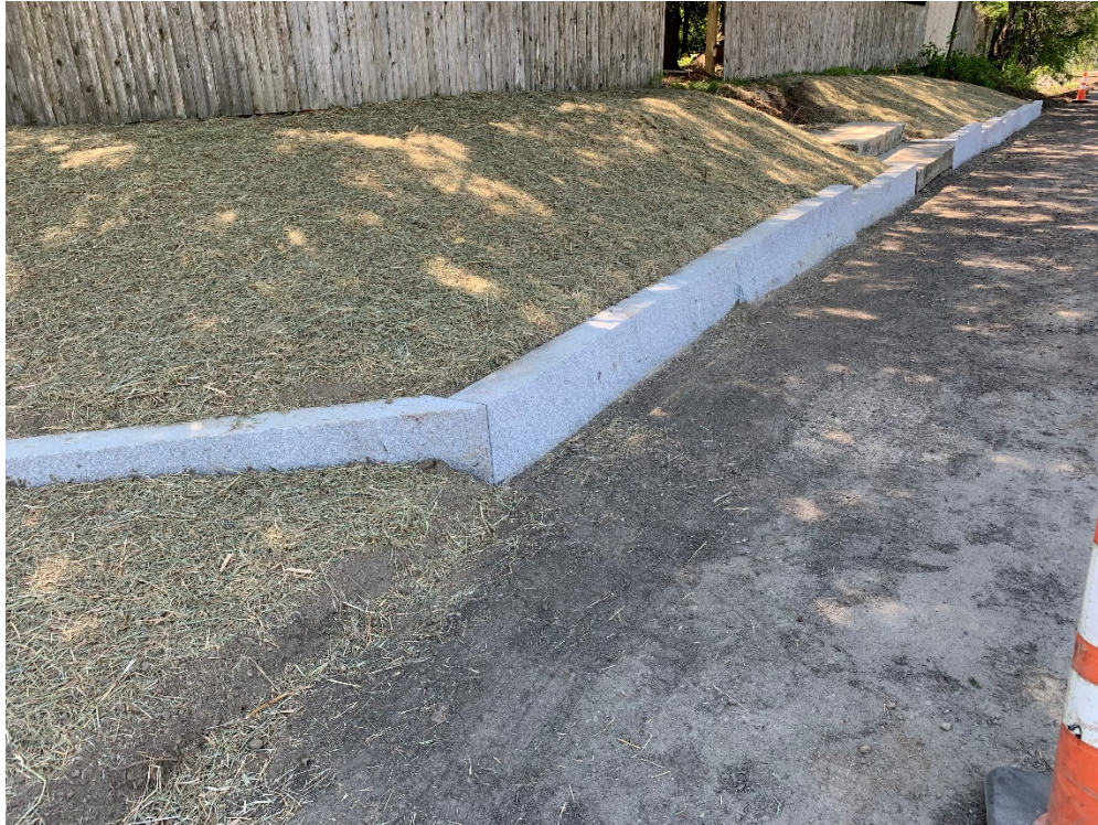
Photo 5 – Granite curb installed as substitute for retaining wall along back of Tuttle Road sidewalk from approximate STA 14+75 to 15+35, 6' R, looking northwest.
