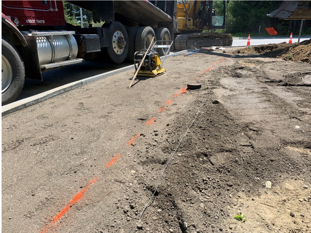
Photo 3 – Compaction of reclaimed pavement in Crossing Brook Road sidewalk, looking southwest.
