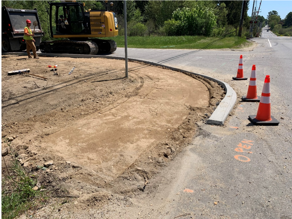
Photo 1 – Subbase gravel placement and compaction in Crossing Brook Road sidewalk from Tuttle Road, looking east.
