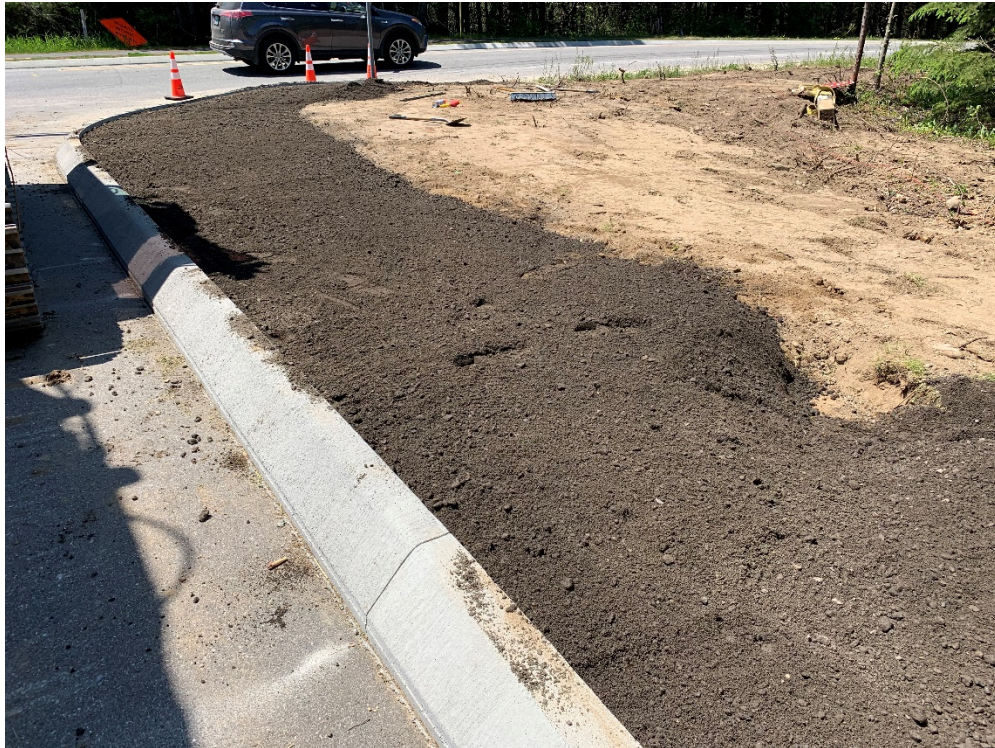
Photo 2 – Placed reclaimed pavement in Crossing Brook Road sidewalk, looking southwest.
