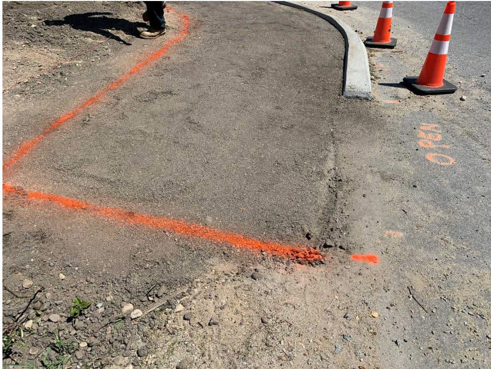
Photo 4 – Compacted reclaimed pavement at sidewalk ramp from Tuttle Road, looking southeast.
