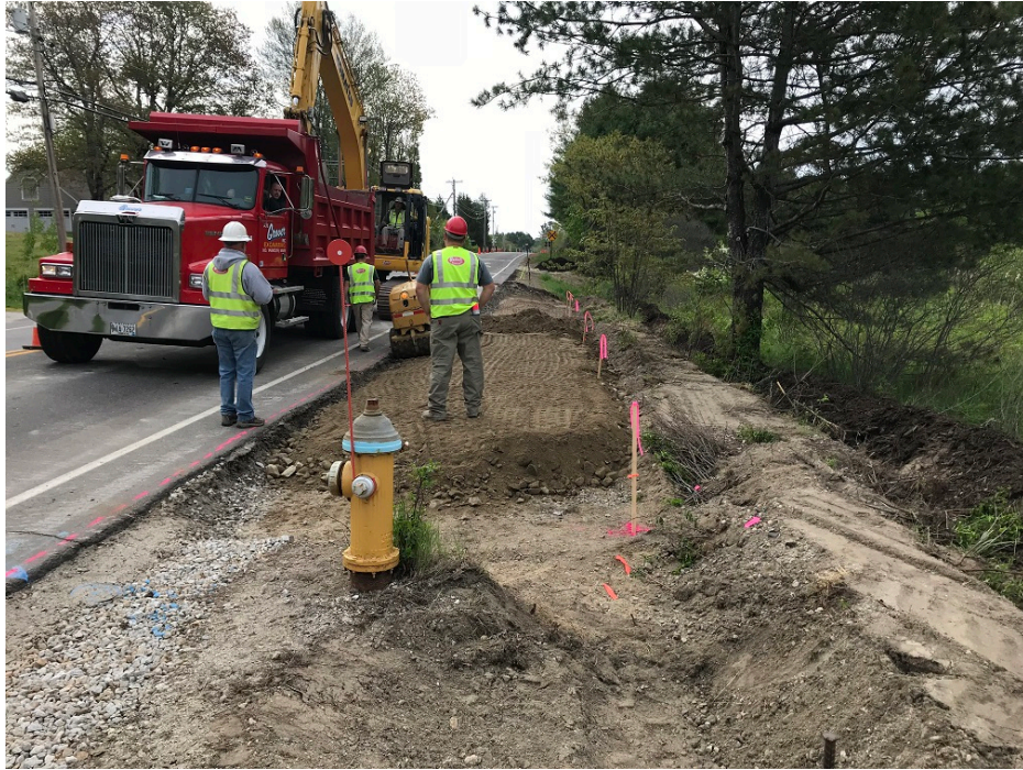
Photo 1 – Working on subgrade for sidewalk toward rail road tracks
