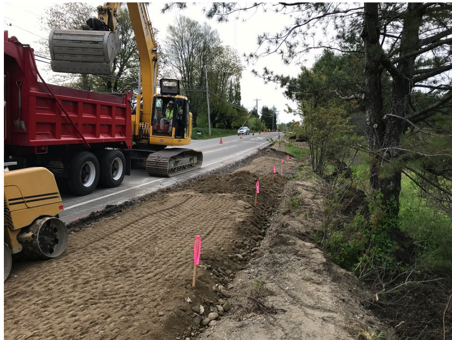
Photo 2 – Placing sidewalk subgrade material for sidewalk extension
