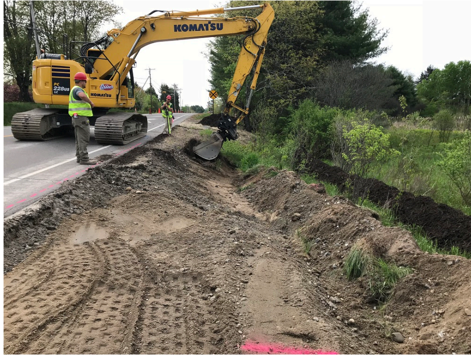
Photo 3 – Removing vegetative soil in area of sidewalk extension
