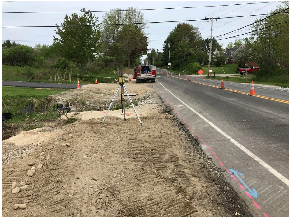
Photo 4 – Sidewalk extension subgrade
