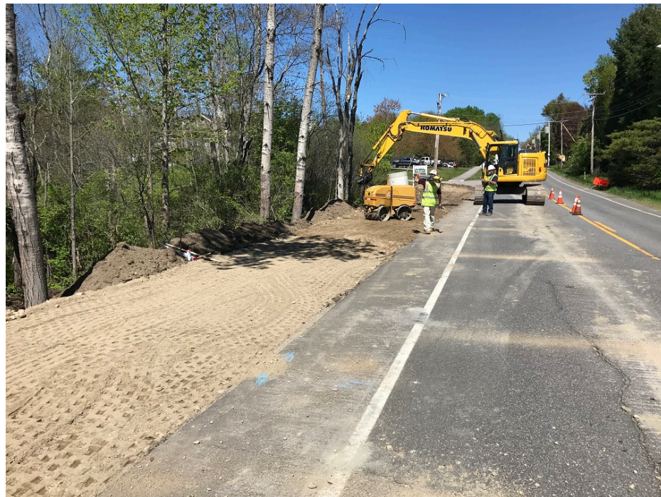
Photo 2 – Compacting sidewalk subgrade
