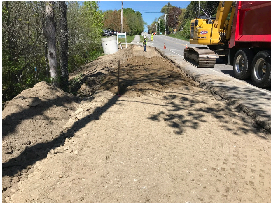
Photo 4 – Working on sidewalk subgrade
