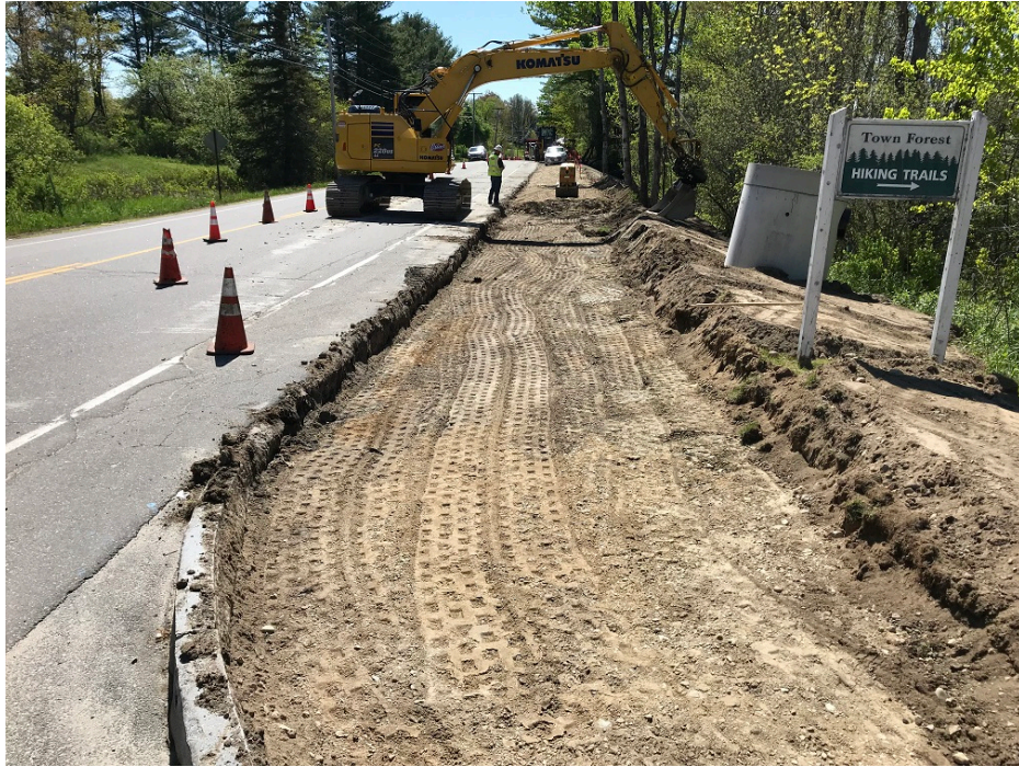
Photo 1 – Working on subgrade for sidewalk
