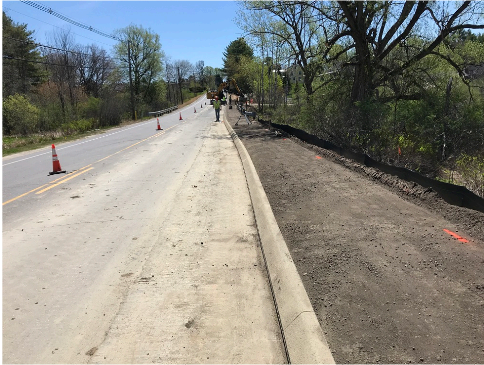
Photo 5 – Graded and compacted reclaim pavement
