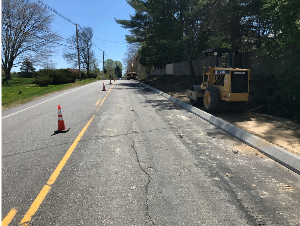
Photo 3 – Compacting subbase gravel in front of 196 Tuttle Road
