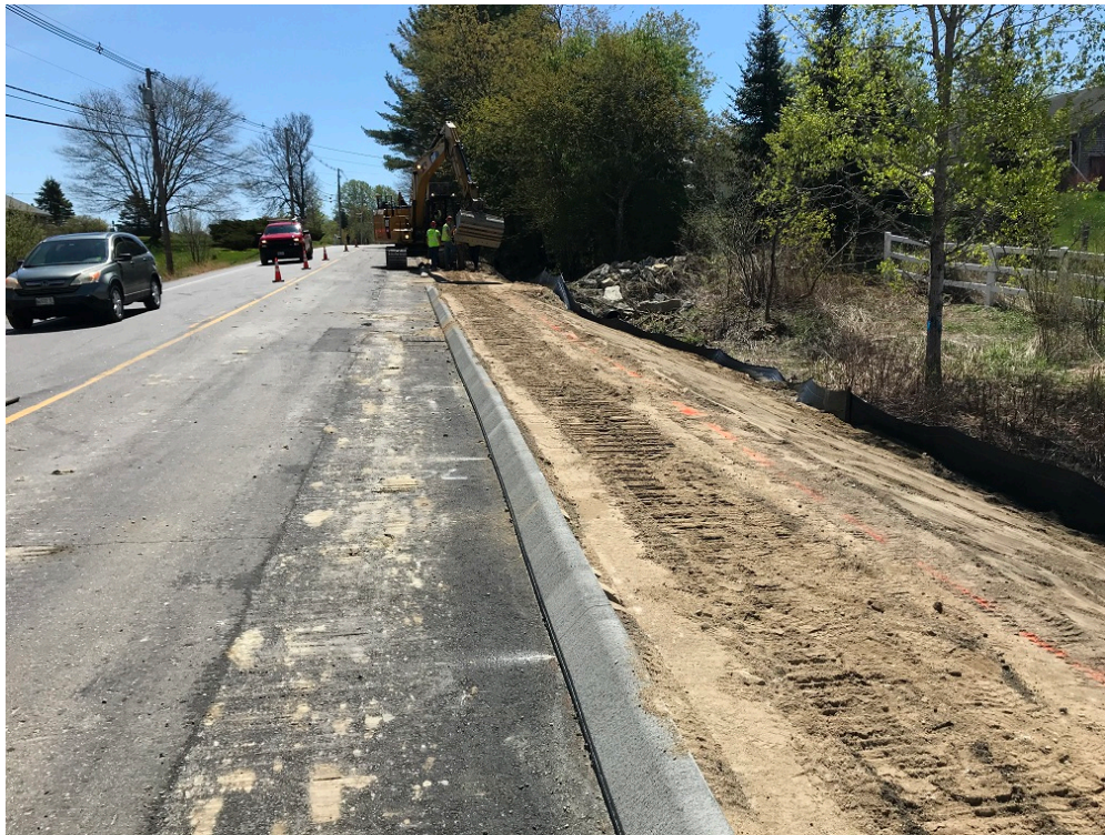
Photo 2 – Grading subbase gravel at approximate STA 12+00
