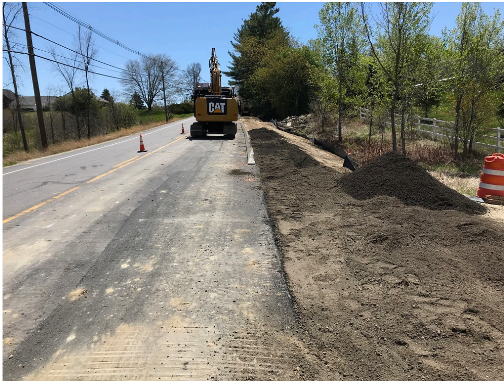
Photo 6 – Placing reclaim pavement at approximate STA 12+00
