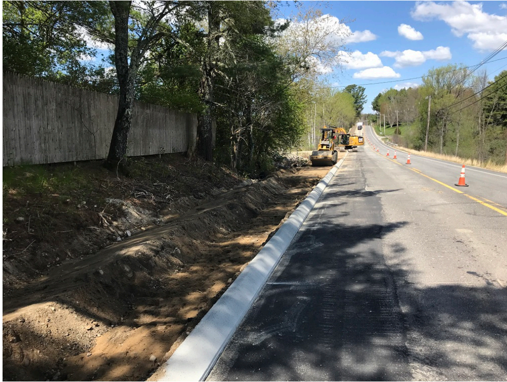
Photo 1 – Excavating for subgrade in front of 196 Tuttle Road
