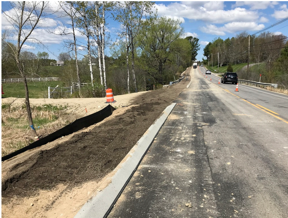
Photo 4 – Placing reclaim pavement at approximate STA 13+00
