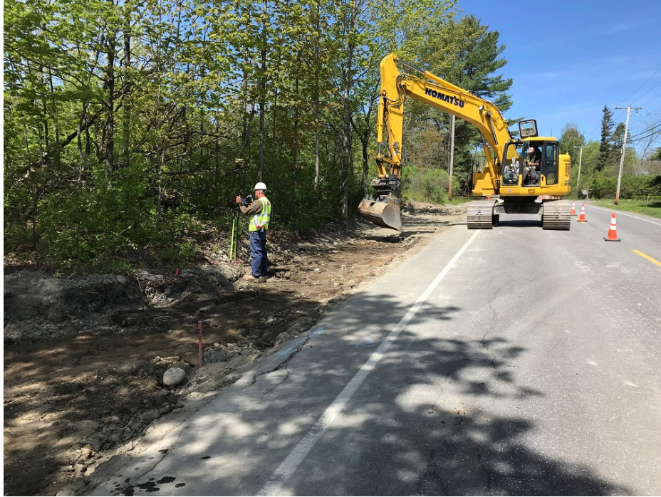
Photo 3 – Setting grades for sidewalk extension subgrade
